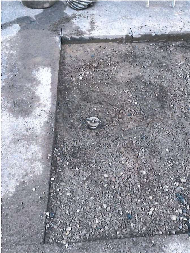
Bottom Left: Photo of the fill pipe with the cover removed.
