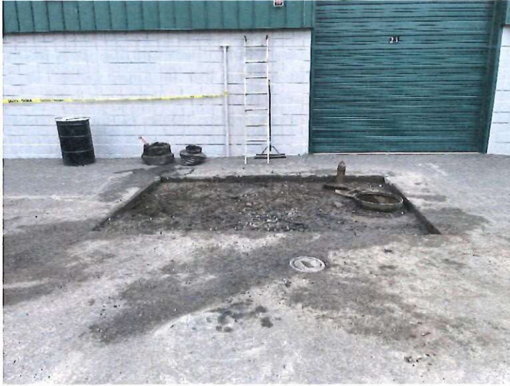
Top: Photo of the cut asphalt above the UST around and between the fill pipe (left) and manhole for tank access (right). Photo taken facing north.
