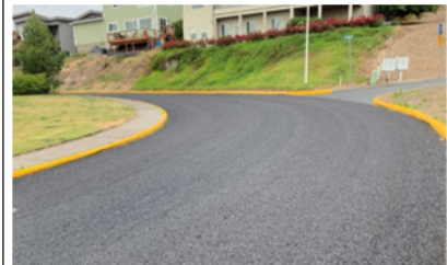
Pictured: A recent fog seal application on E Scenic Dr. – The Dalles.
