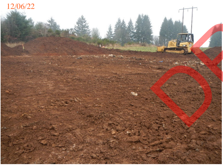
Existing cap soil was pushed to the west side of the USWDC, note exposed solid waste beneath the former soil cap.
