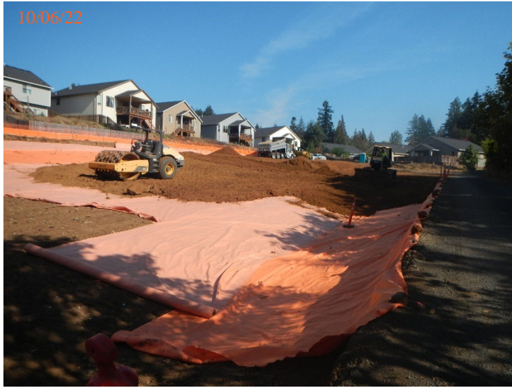
Cap placement activities – view northeast.
