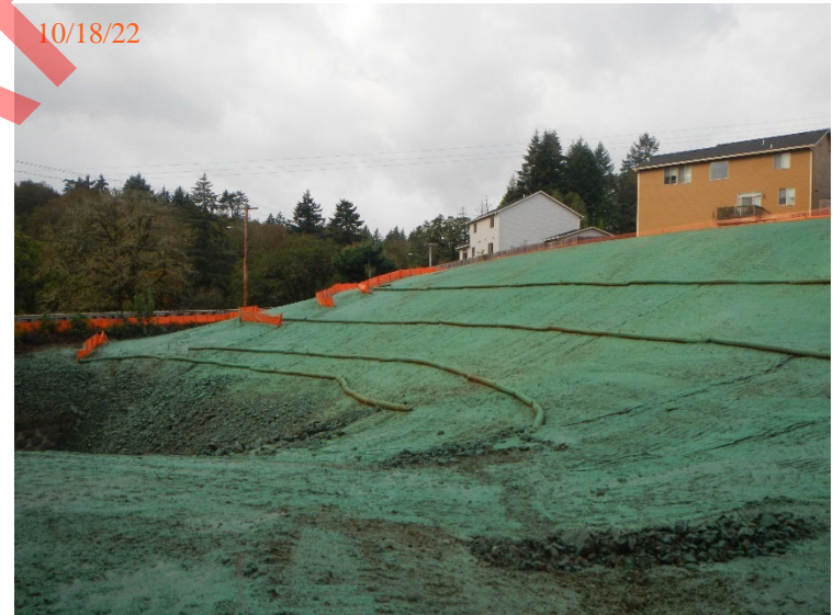
Hydroseed/mulch slopes above the outfall.
