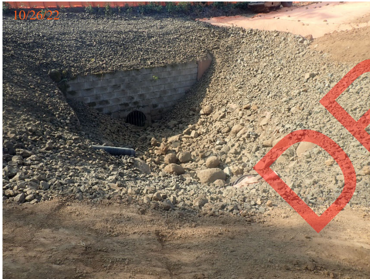
Riprap complete on slopes above outfall.
