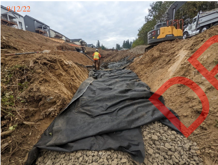
Burrito-wrapping drainpipe and drain rock with the non-woven geotextile.
