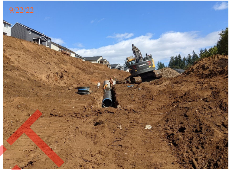
Installation of 30-in ID, double-wall storm water pipe in trench
