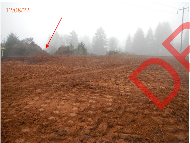
View of the northern portion of the USWDC following soil capping. Arrow pointing to borrow area for clean cap soil.
