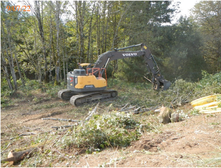
Excavator clearing trees and removing root balls.
