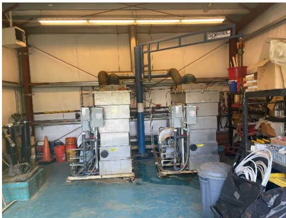
Groundwater is extracted and sent to a small building where the treatment system is housed. The groundwater treatment system is characterized as a shallow tray air stripper system. This photo shows the system being utilized.
