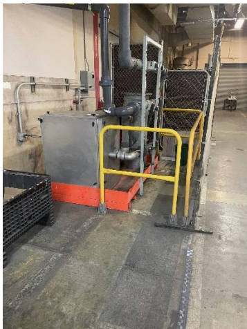
This photo shows a vacuum pump that helps drive the soil vapor remediation system. The pump is located within a building and this photo shows the pump is located alongside a wall and to the side of operational traffic. The pump is on a skid showing that pump is mobile and can be moved if need be.
