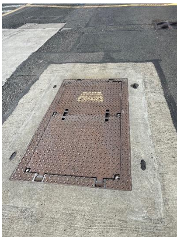
This photo shows the vault for groundwater extraction well E-15. This well is in a general industrial area of the site and shows durable construction.
