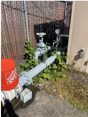
This photo shows the treated groundwater discharge pipe from the shallow tray stripper system. The clean treated groundwater is discharged into the Gresham stormwater system and eventually flows to the Gresham wastewater treatment plant with final discharge to the Columbia River.
