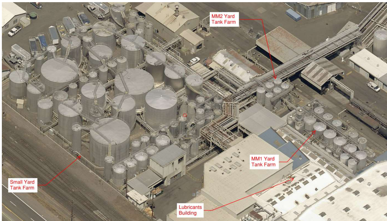
Figure 2-4: Aerial of Small Yard, MM1 and MM2 Tank Farm
