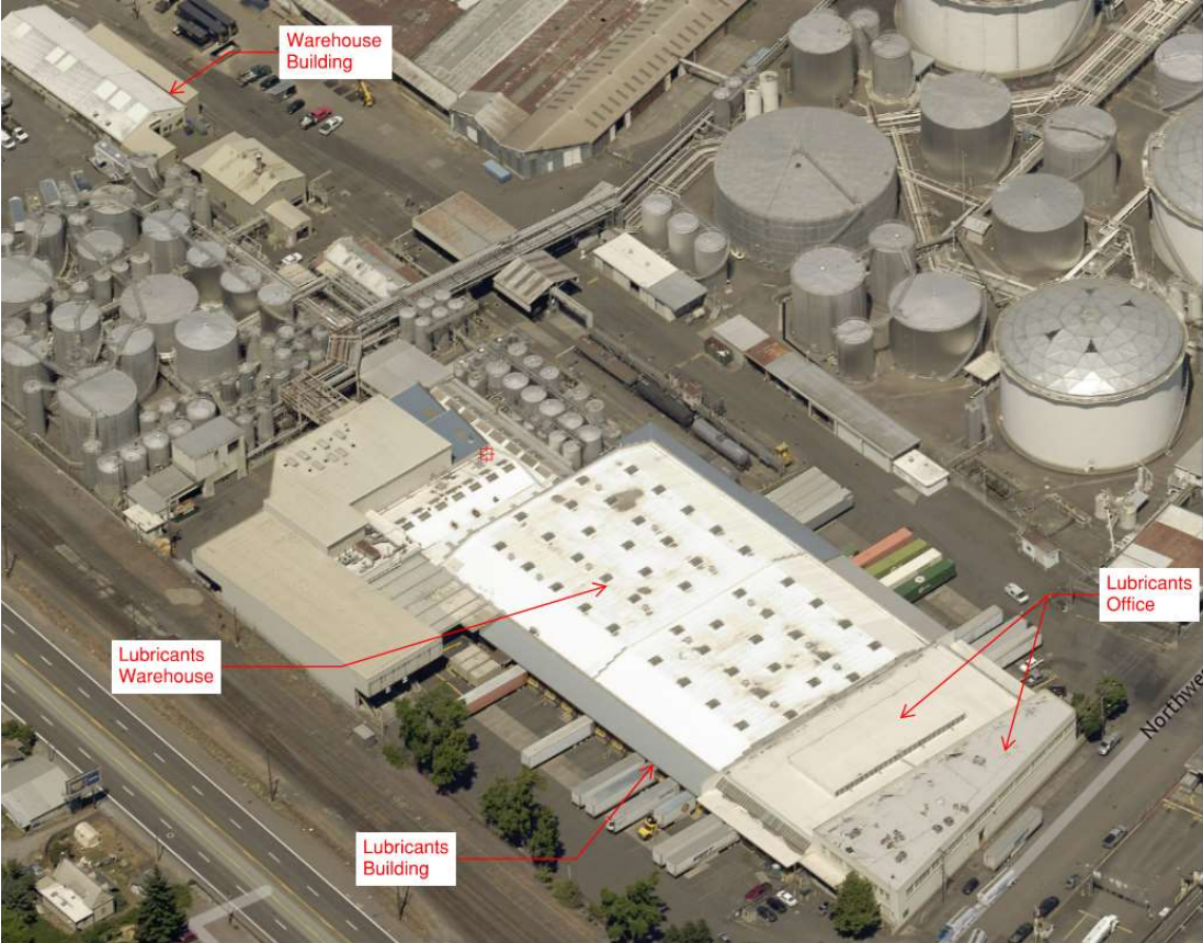
Figure 2-7: Aerial view of Lubricants and Maintenance Building
