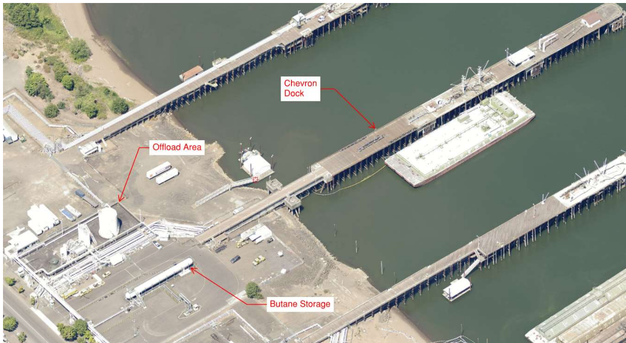
Figure 2-5: Aerial of Offload Area, Butane Storage and Dock
