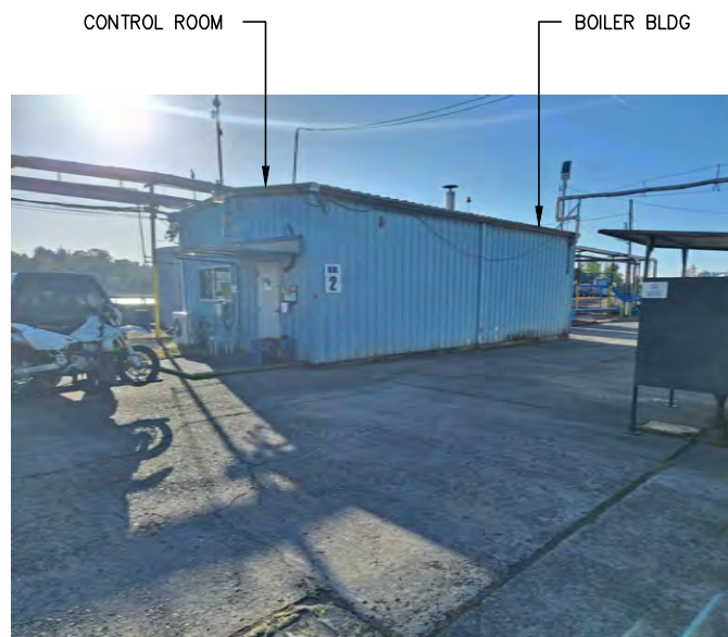
PHOTO #2 - CTRL RM/BOILER BDLG
