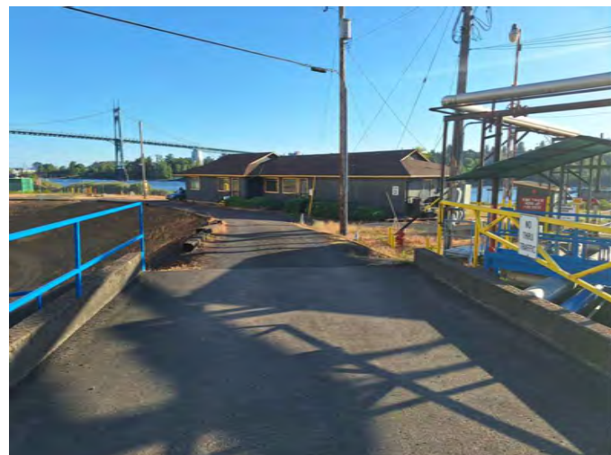
PHOTO #1 - OFFICE BLDG
