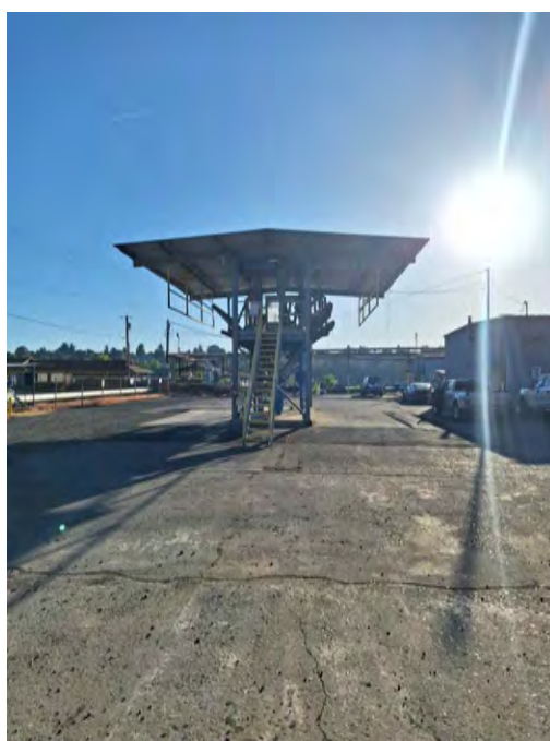
PHOTO #4 - TRUCK LOAD RACK
