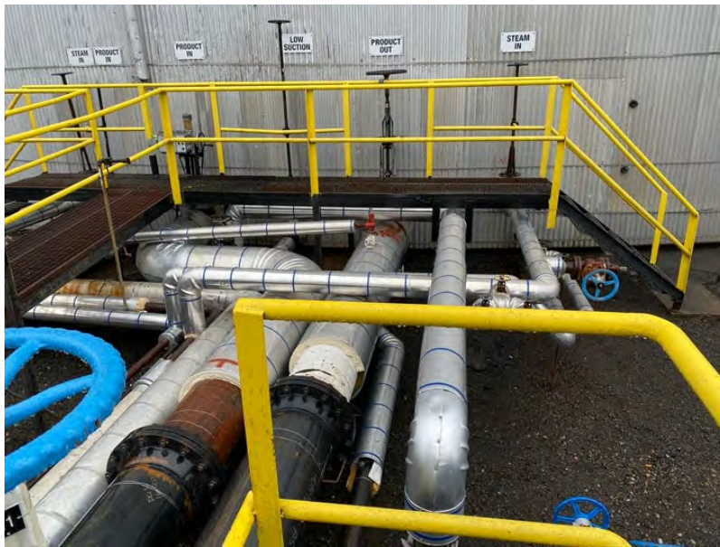
Figure 14. Tank 105 and the attached piping system.
