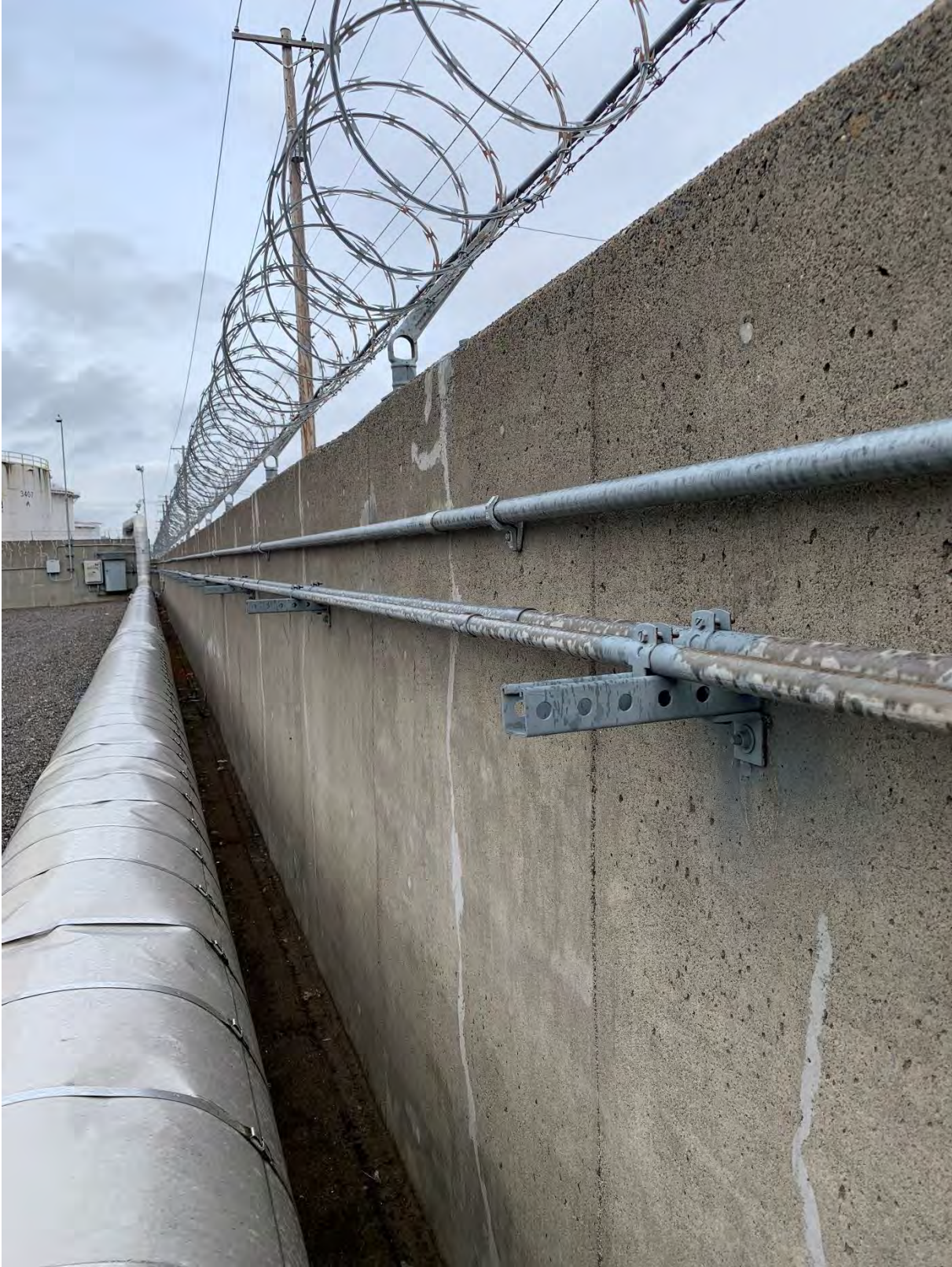
Photo 4 - 6.0-foot Concrete Cantilever Wall
