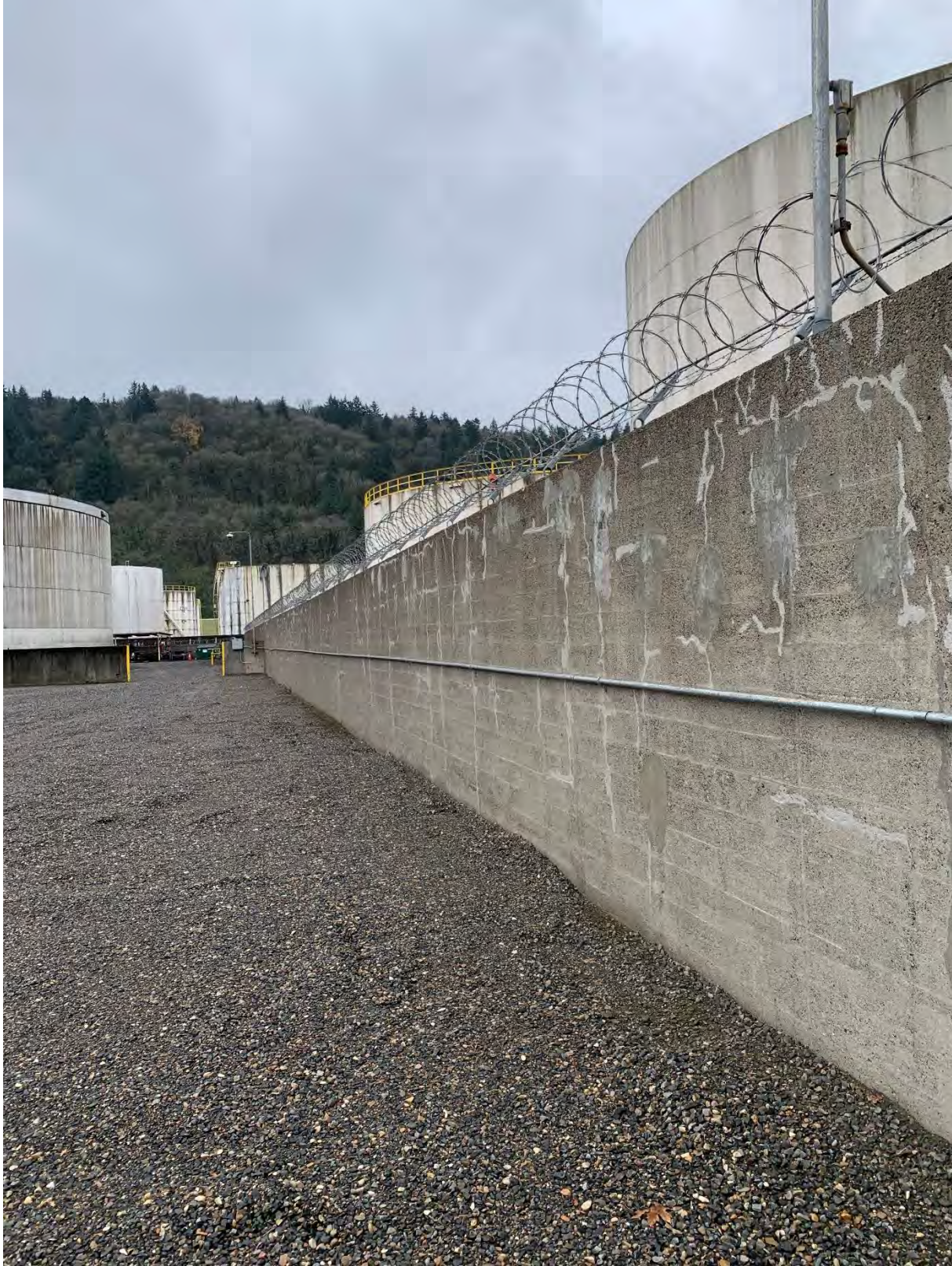
Photo 5 - 9.3-foot Concrete Containment Wall
