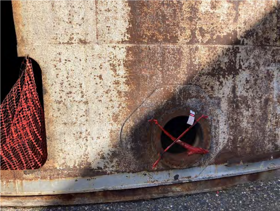
Figure 9. Tank 127 non-code features.
