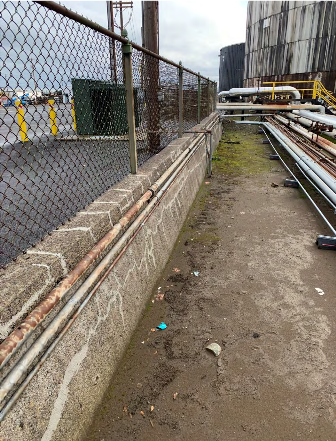
Photo 1 - 3.0-foot Concrete Gravity Wall
