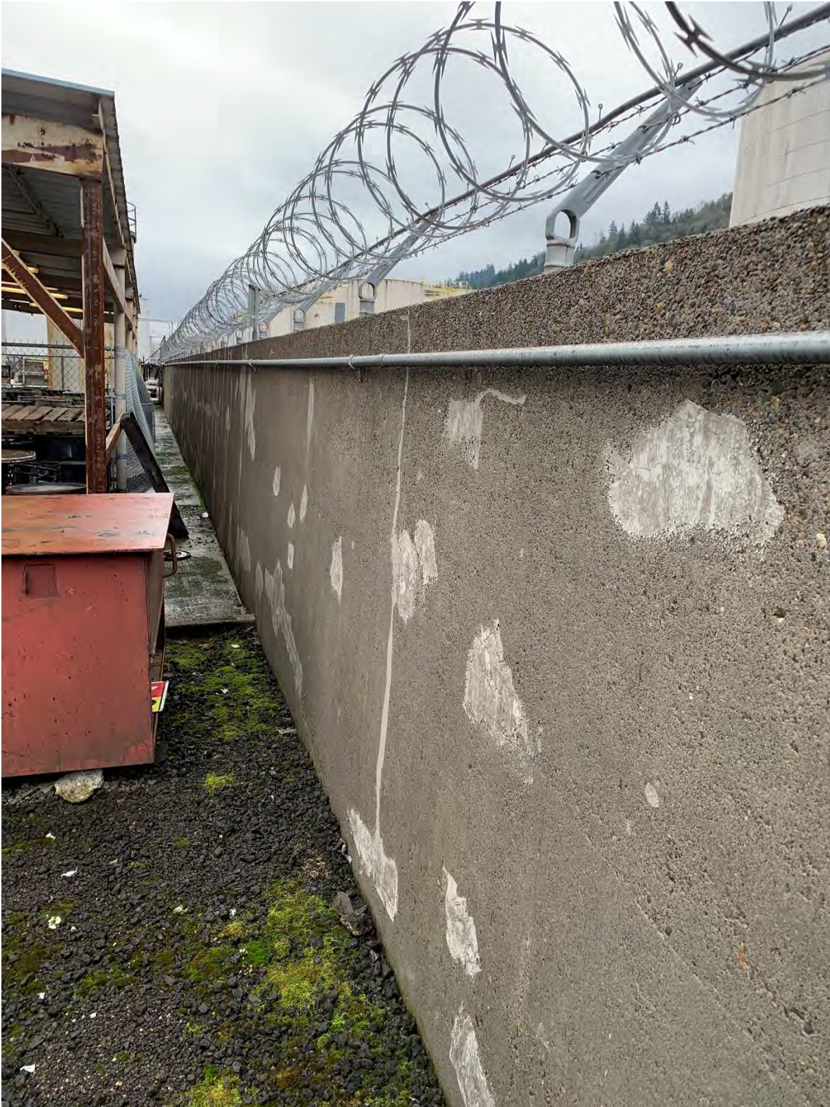
Photo 3 - 6.5-foot Concrete Cantilever Wall
