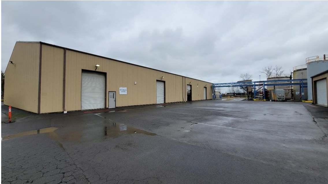
Picture 7. Typical view of light-framed storage building.
