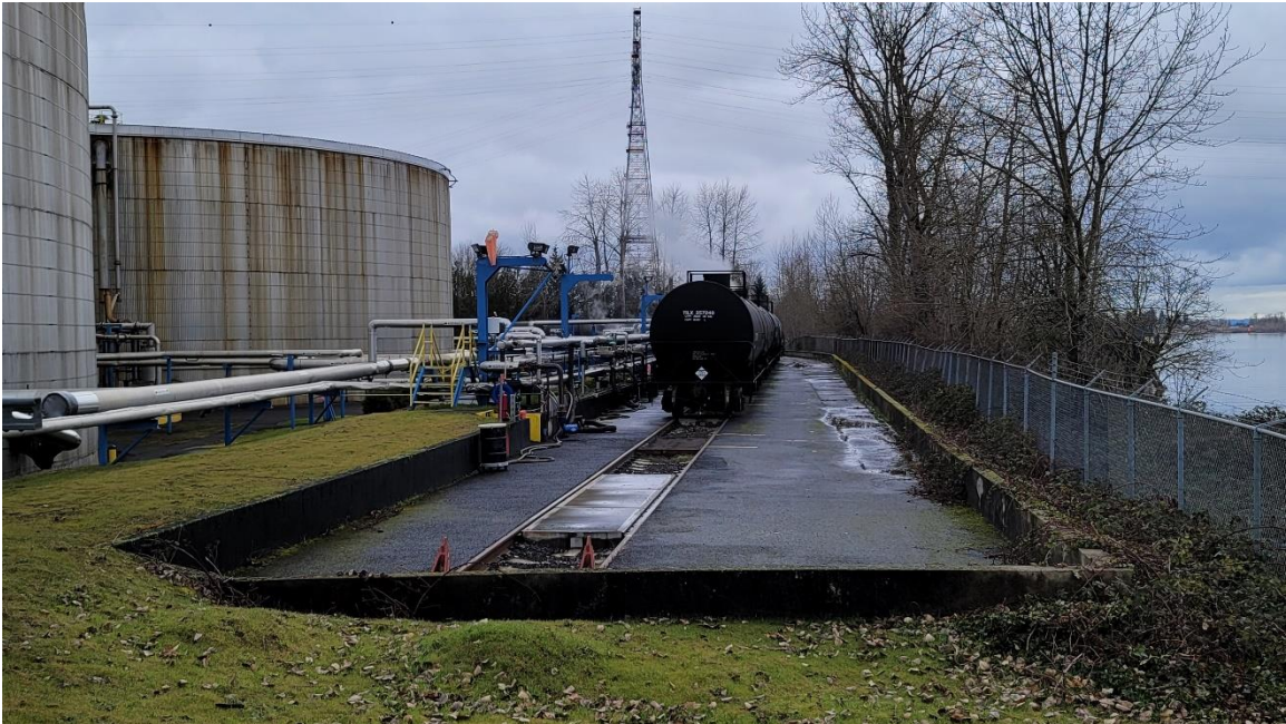
Picture 11. Typical view of Rail Spur.
