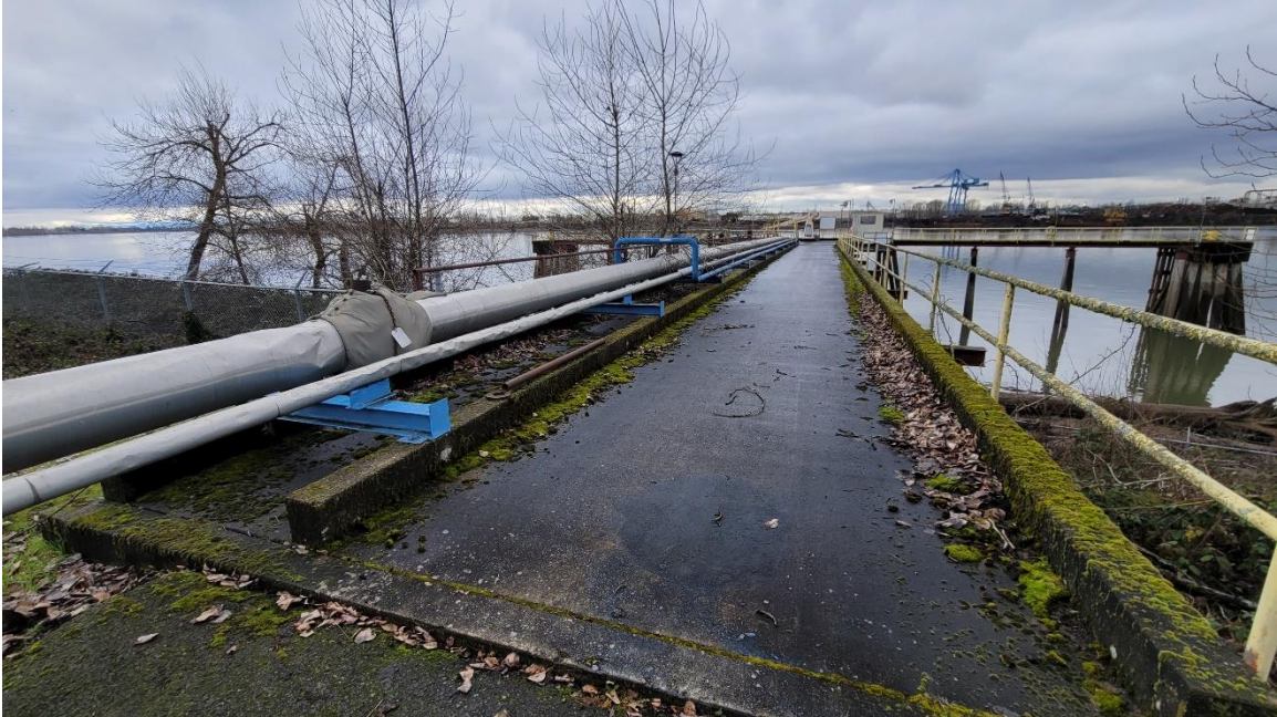
Picture 13. View of piping at dock structure.
