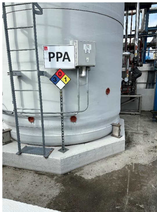
Picture 6. View of anchorage provided at smaller tank.
