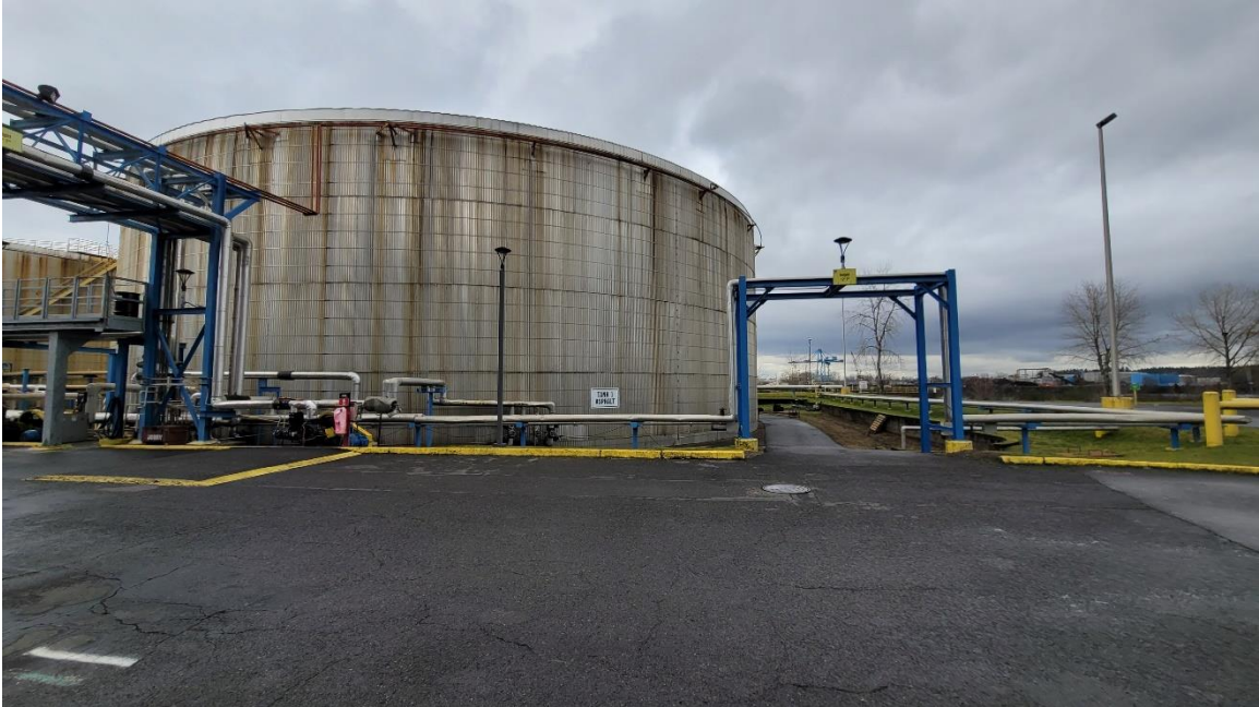
Picture 9. View of large tank at tank farm area.
