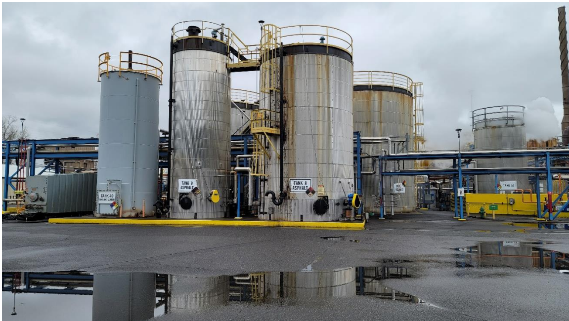
Picture 2. View of tanks at Process Area.
