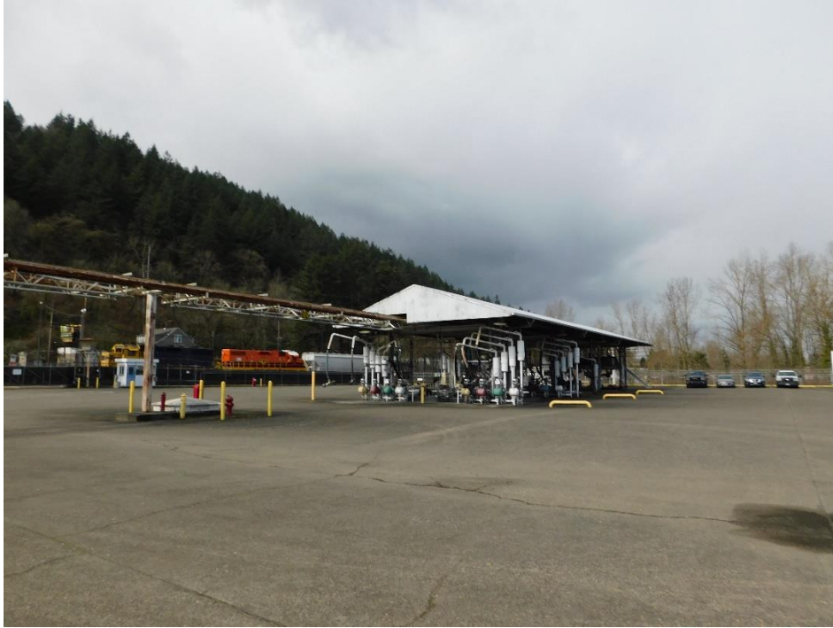
Picture 1. View of out-of-service truck loading rack and pipe bridge at Area 01.
