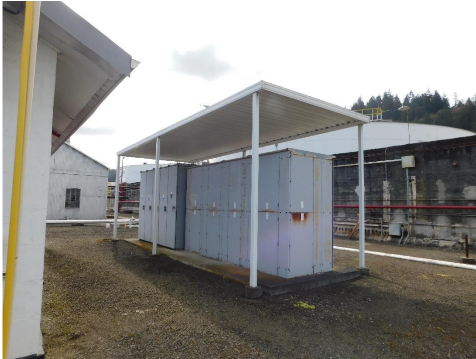
Picture 13. Typical view of canopy structure at Area 02.
