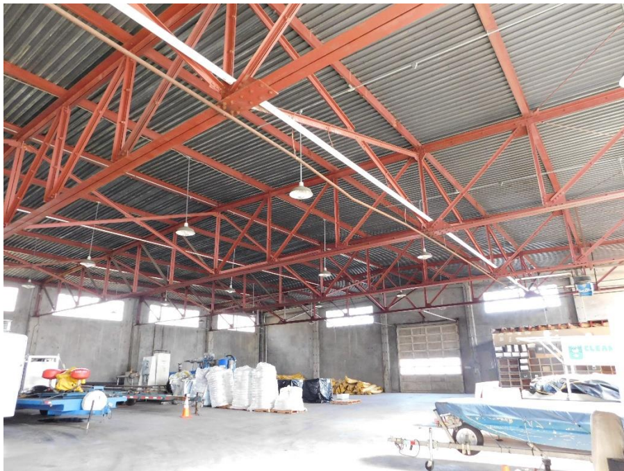
Picture 4. New roof structure at Warehouse A.
