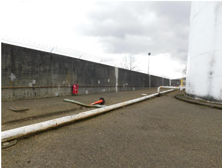
Picture 8. Typical containment wall structure.
