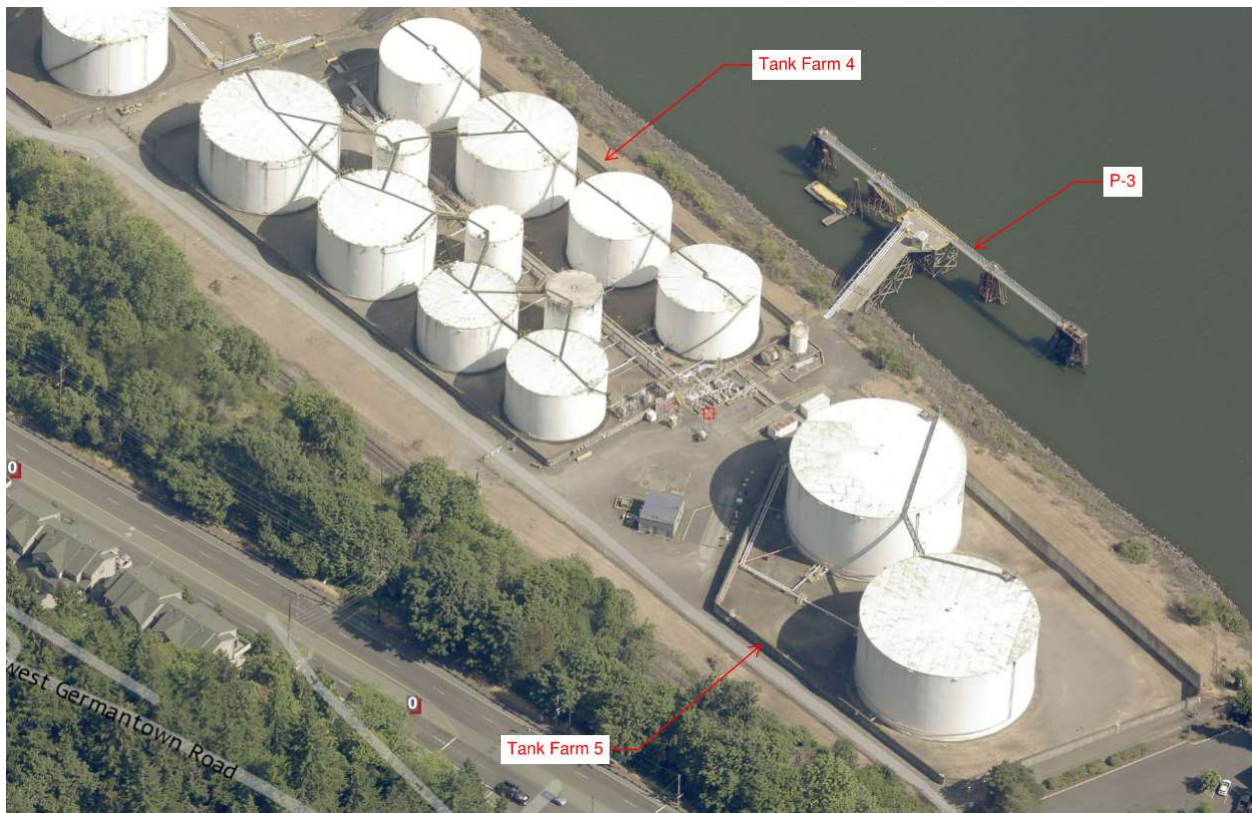
Figure 2-5: Aerial of Tank Farm 4 & 5 and P-3 Dock
