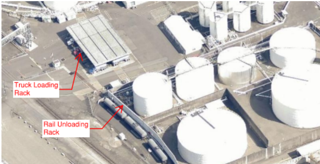
Figure 2-6: Aerial of Loading Racks
