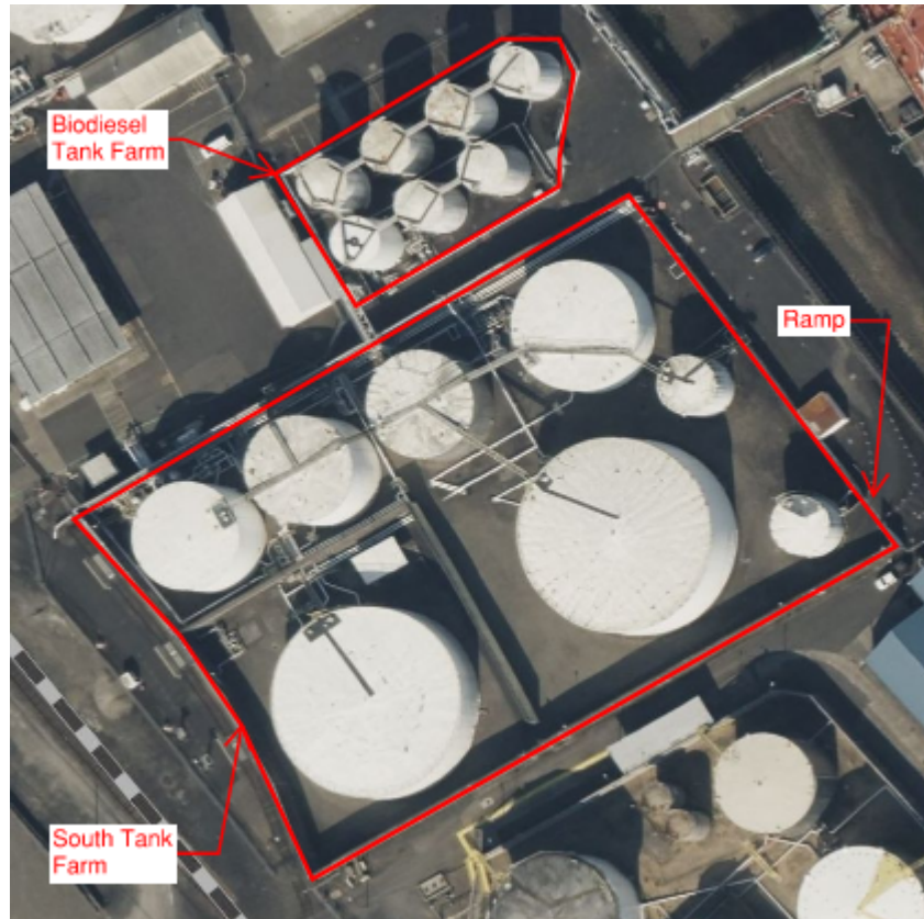
Figure 2-4: Aerial of South Tank Farm and Biodiesel Tank Farm
