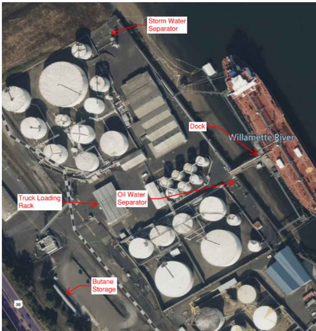
Figure 2-5: Aerial of Water Separators, Butane Storage, and Dock
