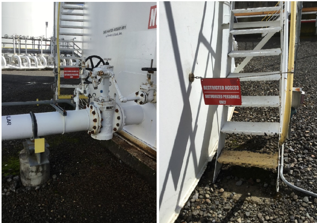
Figure E-1: Example Over-Constrained Conditions
