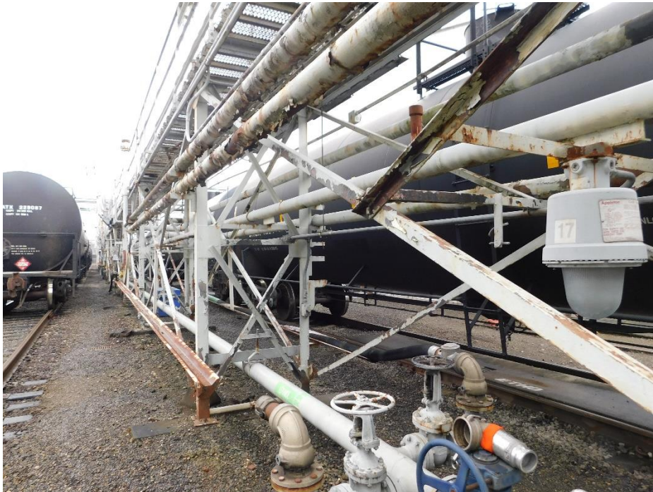
Picture 18. Typical view of rail transfer platform.
