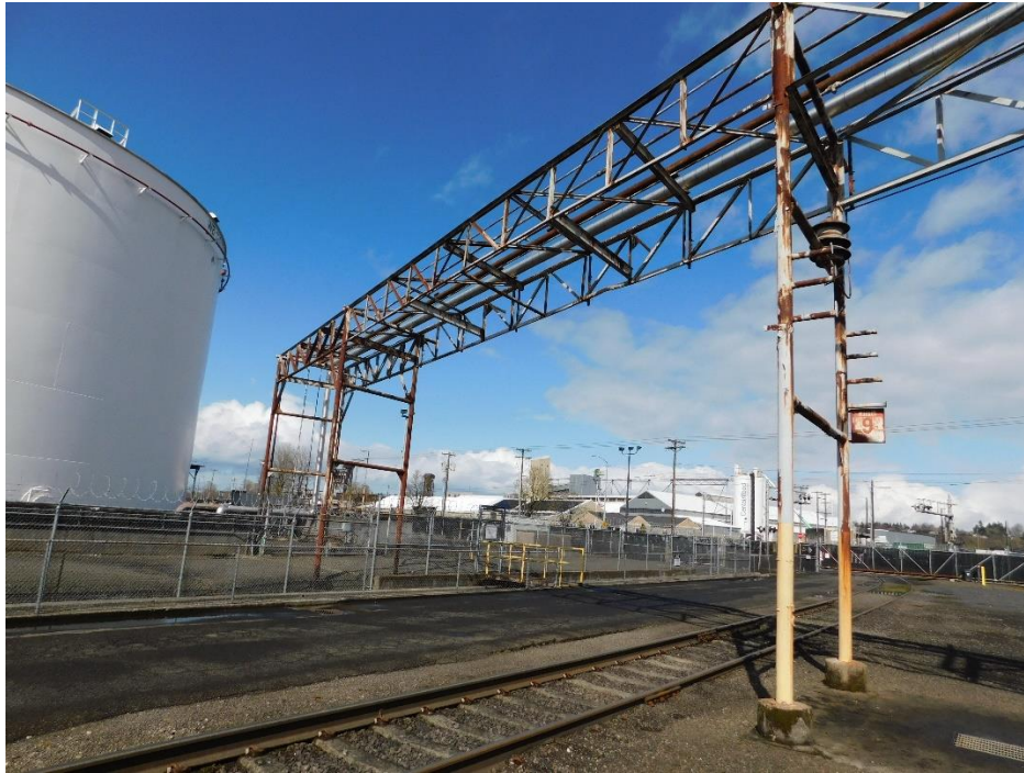
Picture 21. View of "Pipe Bridge 3" at Rail Transfer Area.
