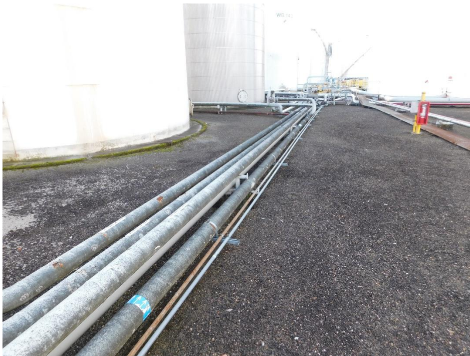
Picture 2. Typical view of pipe runs at North Yard.
