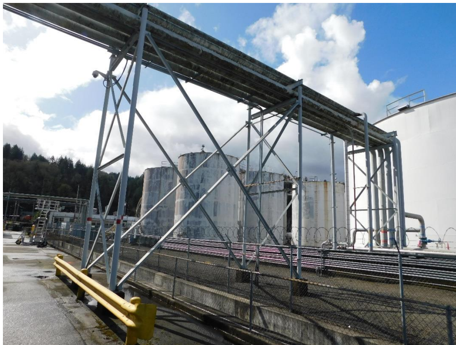
Picture 20. View of "Pipe Bridge 2" at Rail Transfer Area.
