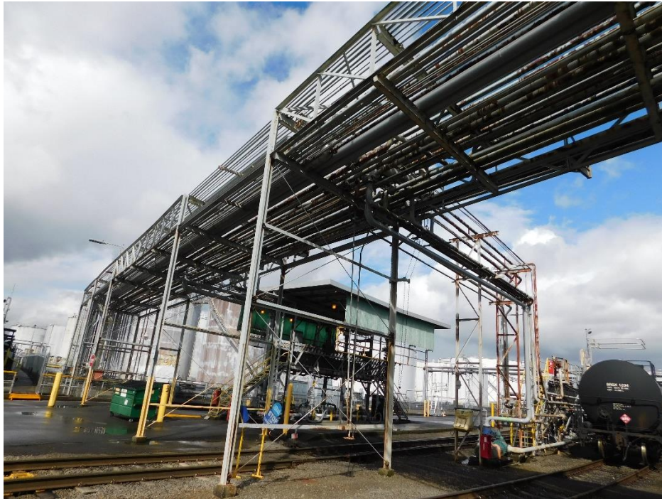
Picture 19. View of "Pipe Bridge 1" at Rail Transfer Area.
