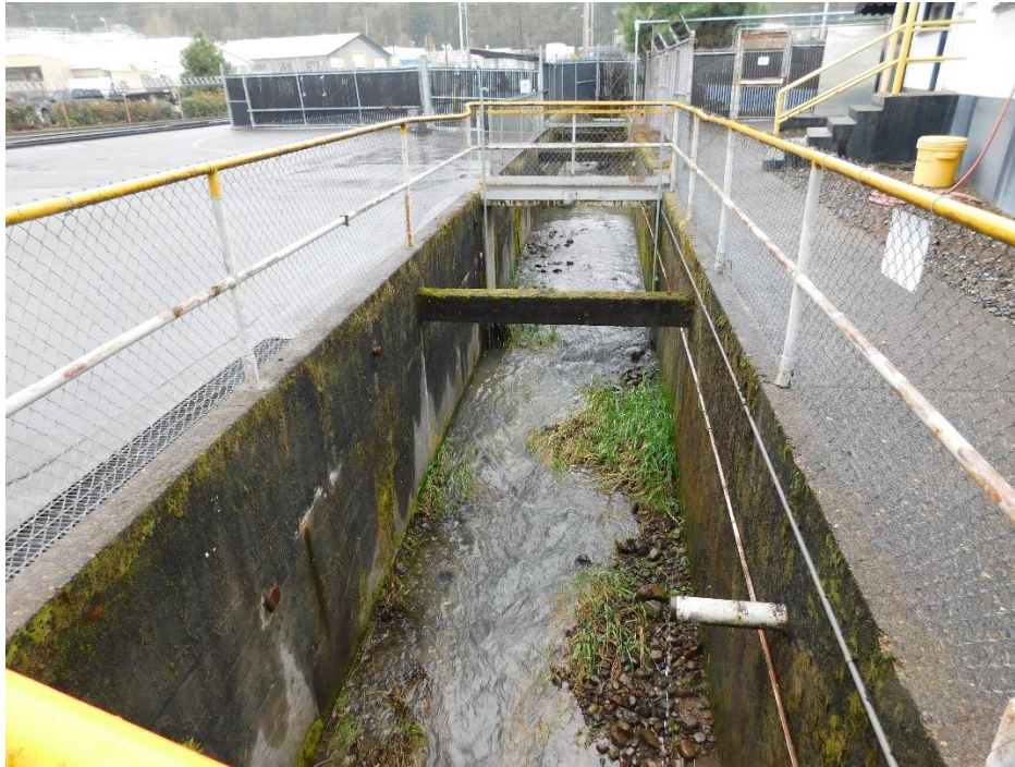
Picture 9. Saltzman Creek storm flume.
