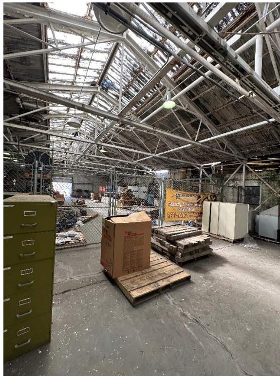
Picture 22. Typical view of light framed structure at Warehouse area.
