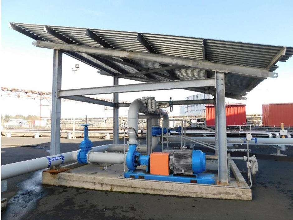
Picture 13. Typical view of canopy structure at North Yard.
