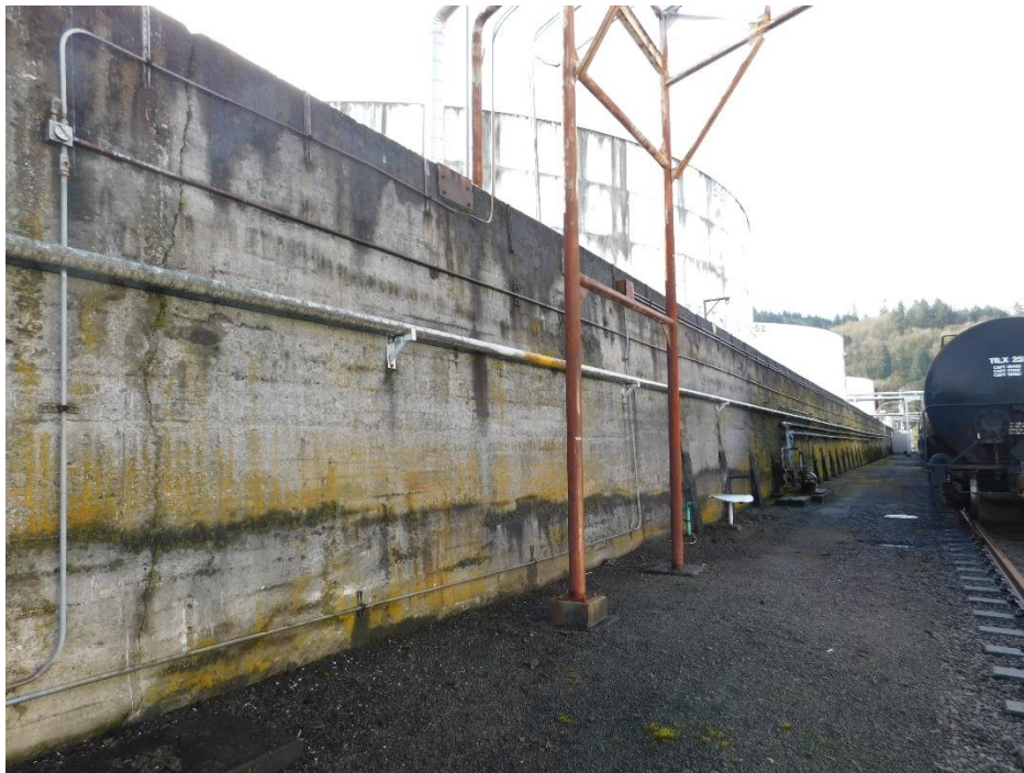
Picture 16. Typical view of containment walls at South Yard.
