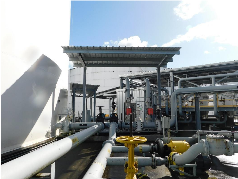
Picture 17. View of typical canopy structure at South Yard.
