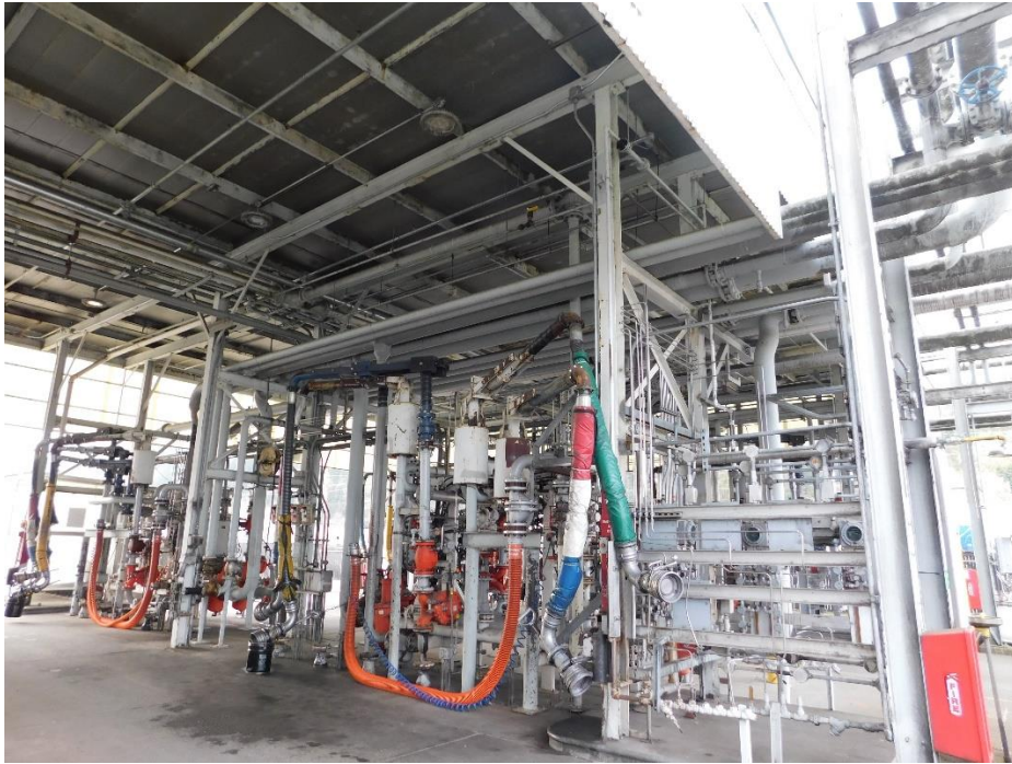
Picture 7. North Yard truck loading rack framing.
