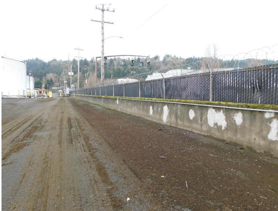
Picture 8. Containment wall structure at North Yard.
