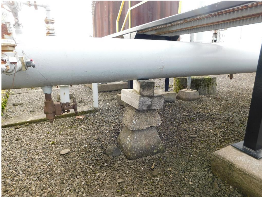
Picture 5. Pipe supported by wood and concrete blocks at North Yard.
