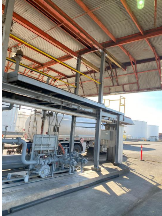
Picture 3. View of typical truck loading rack framing.
