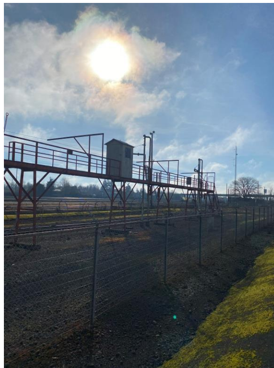
Picture 10. Tank car loading rack at South Yard.
