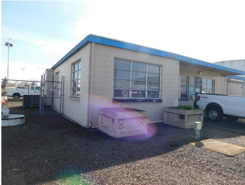
Picture 9. View of office building.
