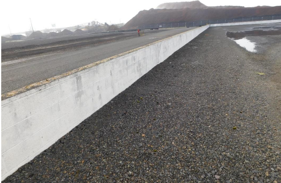
Picture 5. Typical view of containment wall.
