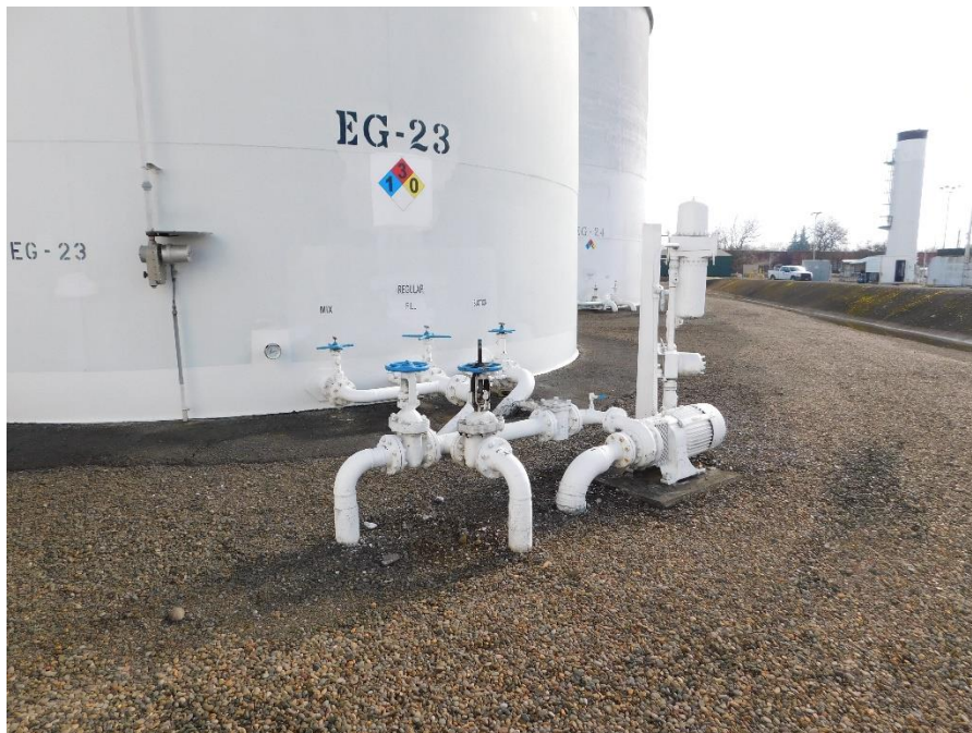
Picture 4. Typical view of buried piping.
