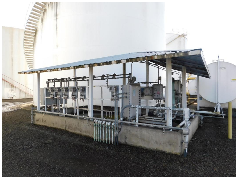
Picture 8. Typical canopy structure.
