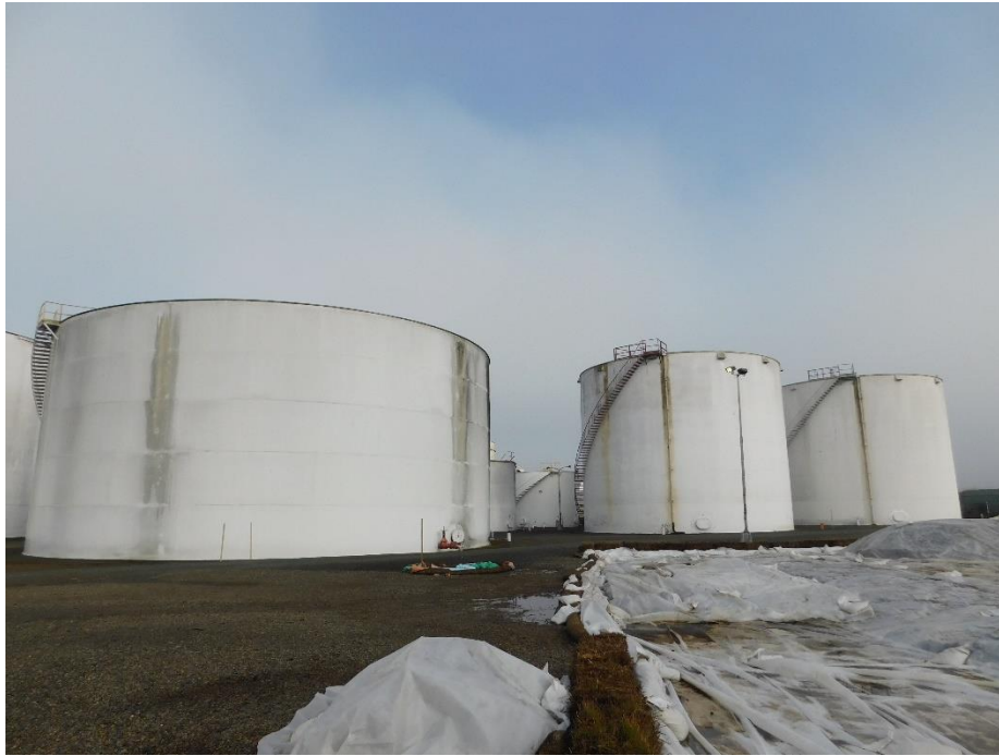
Picture 1. Typical view of tank farm.
