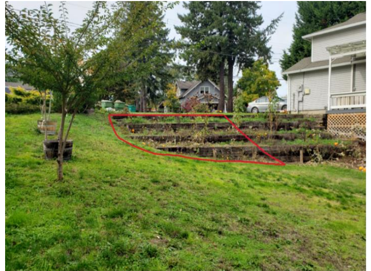
Figure 2 the existing railroad ties will need to be removed at 740 Wynooski St and the existing 40% slope will need to be filled in to about a 20% accessible slope
