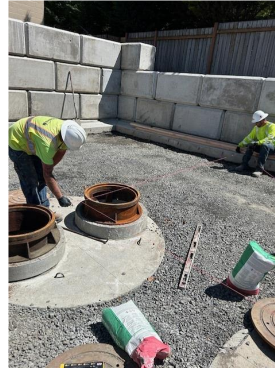
72" Manholes Being Set by Crew for decant at PW maintenance yard
