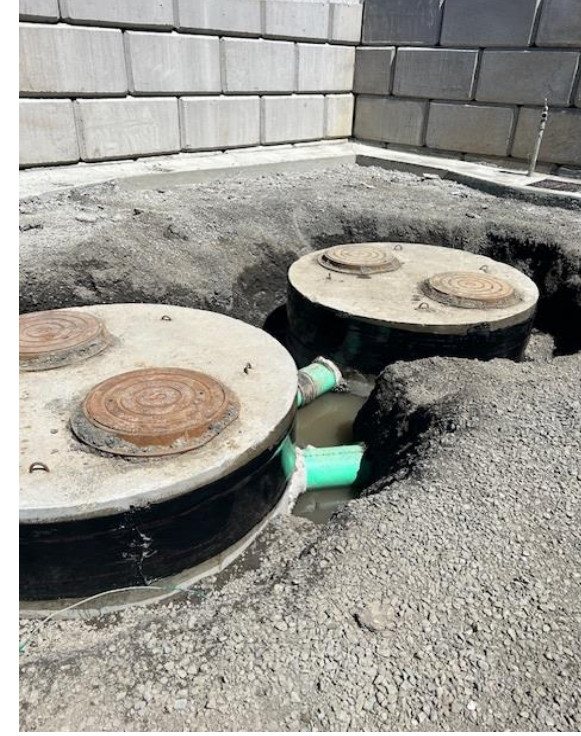
72" Manholes Being Set by Crew for decant at PW maintenance yard
