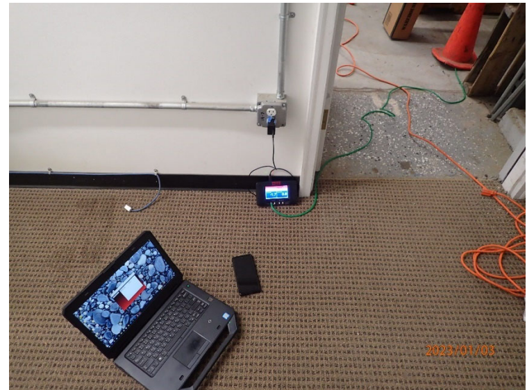
TEC DG-1000 pressure gauge deployed to monitor differential sub-slab pressure at SUB18 (inside removal action area) vs. indoor air.
