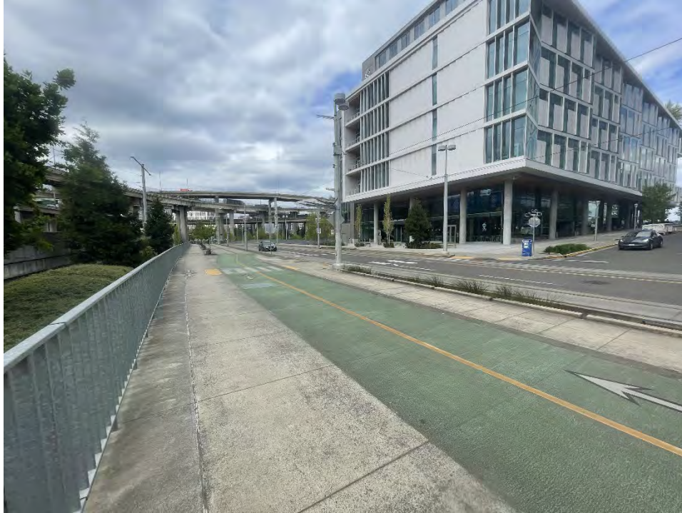
Photograph 9. South Meade Street, looking northeast.
