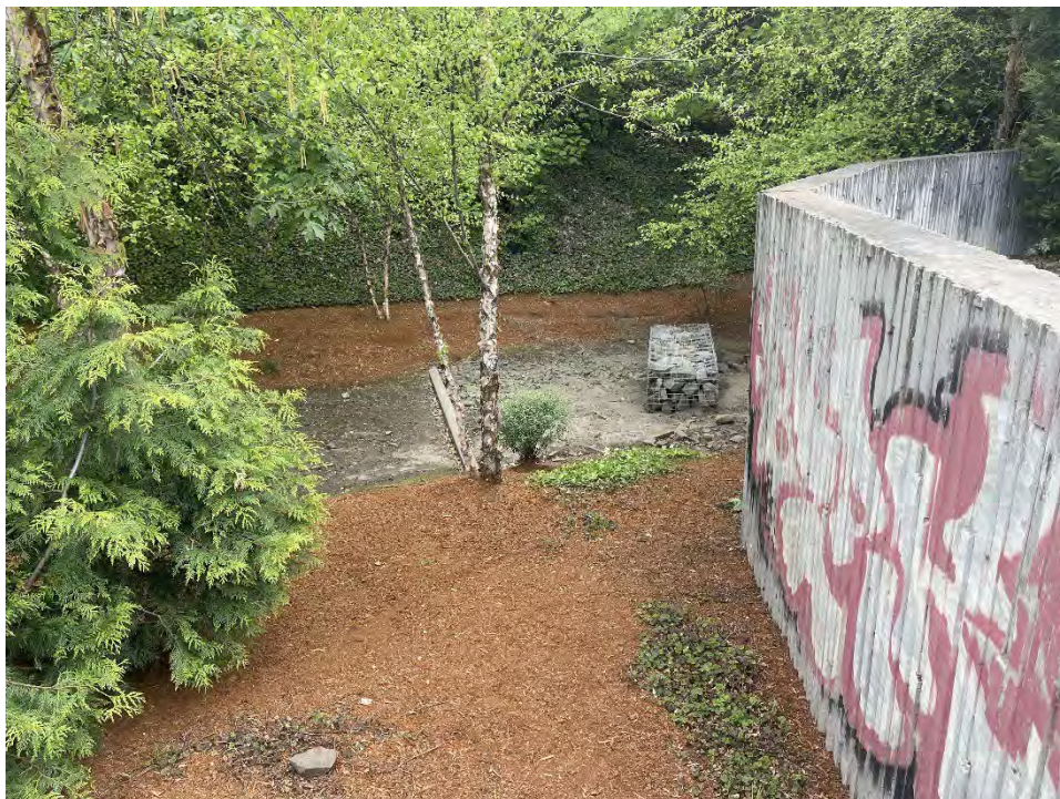
Photograph 29. Stormwater swale, looking west.
