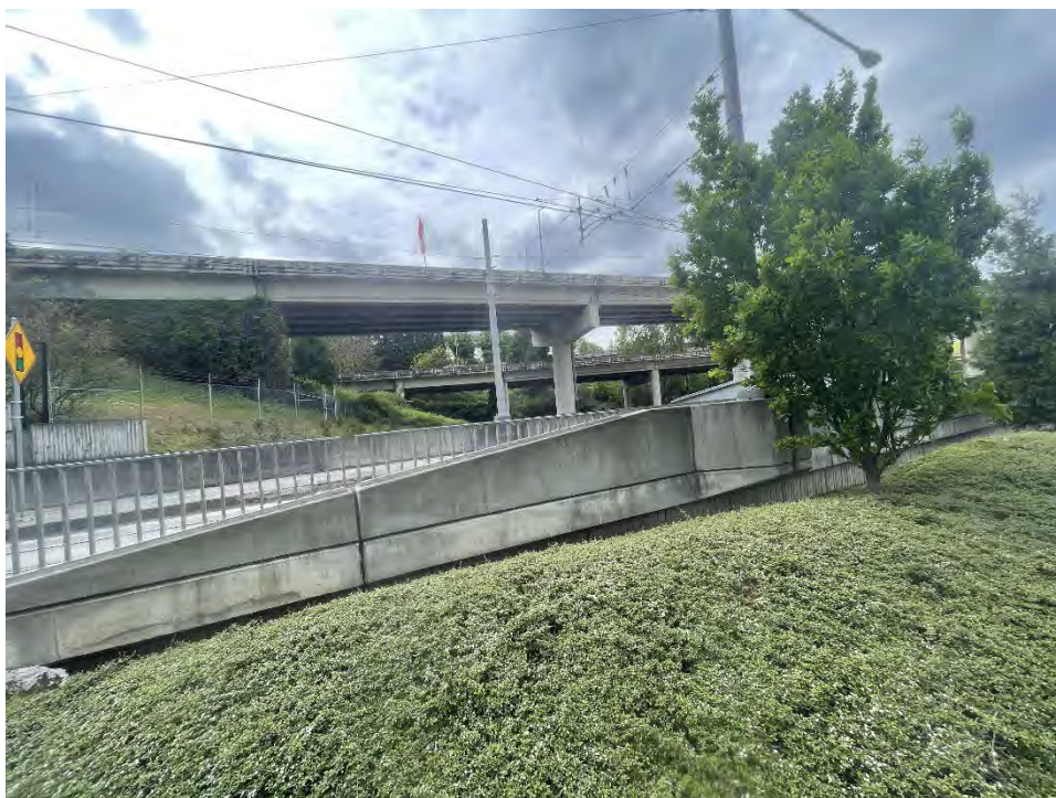
Photograph 30. TriMet light rail, looking northwest.
