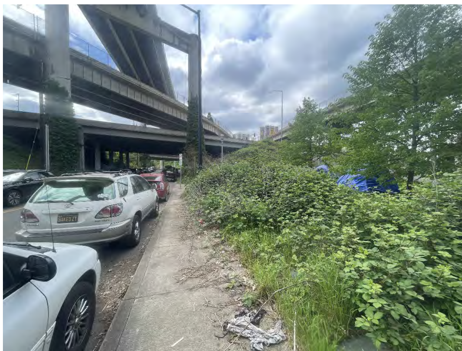
Photograph 1. Northwest corner, looking east.
