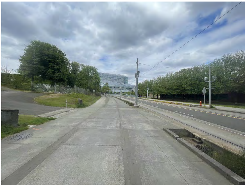
Photograph 15. Southeast corner, looking north.
