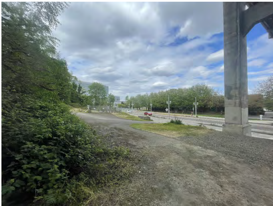
Photograph 17. Southwest corner, looking northeast.
