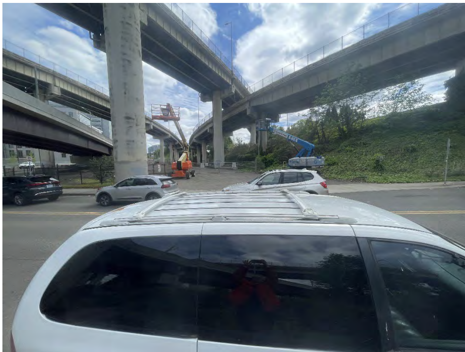
Photograph 3. Northwest corner, looking south.
