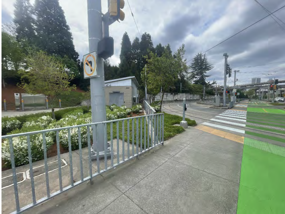
Photograph 23. Maintenance shed, looking northwest.
