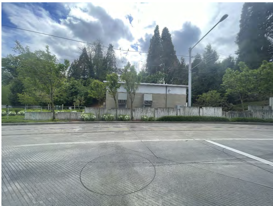
Photograph 22. Maintenance shed, looking south.
