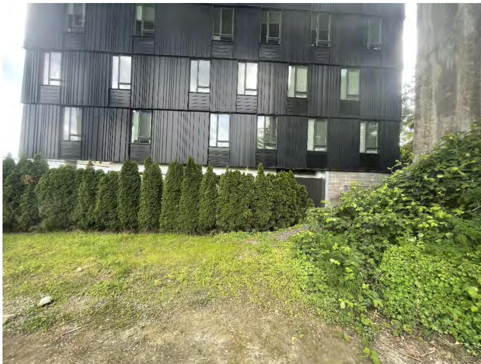
Photograph 19. Southwest corner, looking south.
