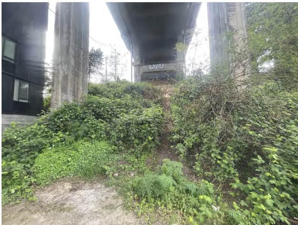
Photograph 20. Southwest corner, looking west.
