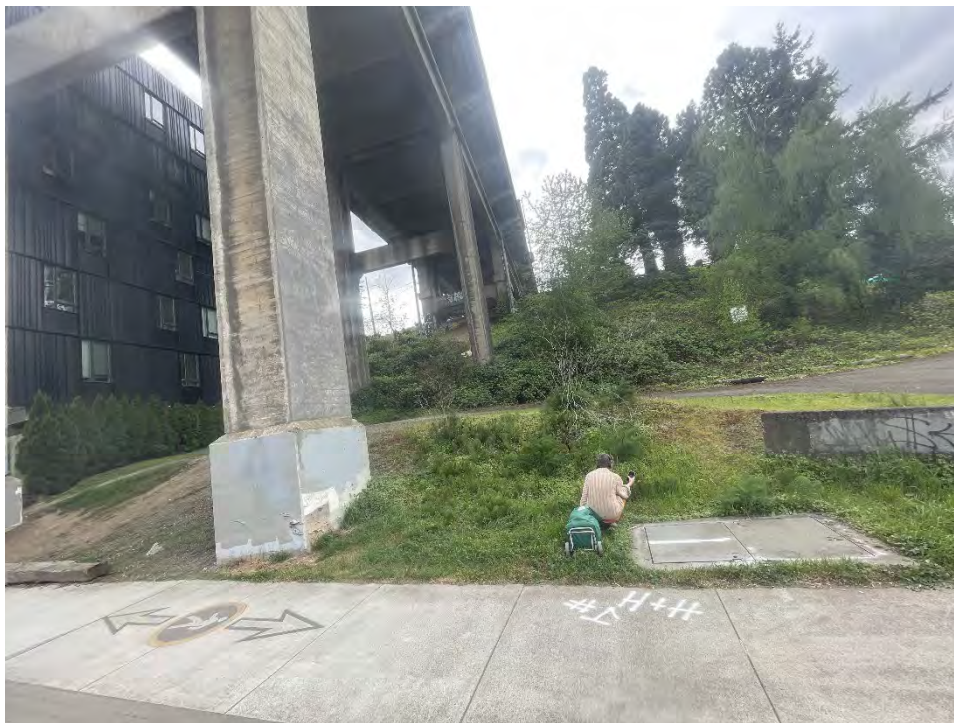
Photograph 13. Southeast corner, looking west.
