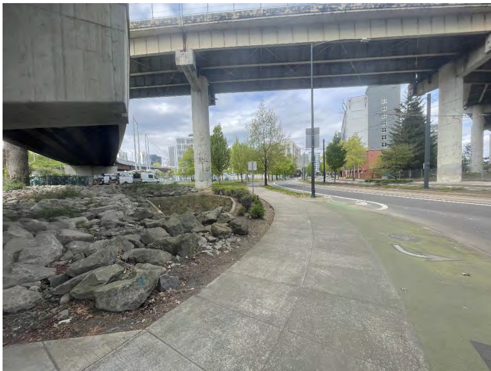
Photograph 7. Northeast corner, looking north.
