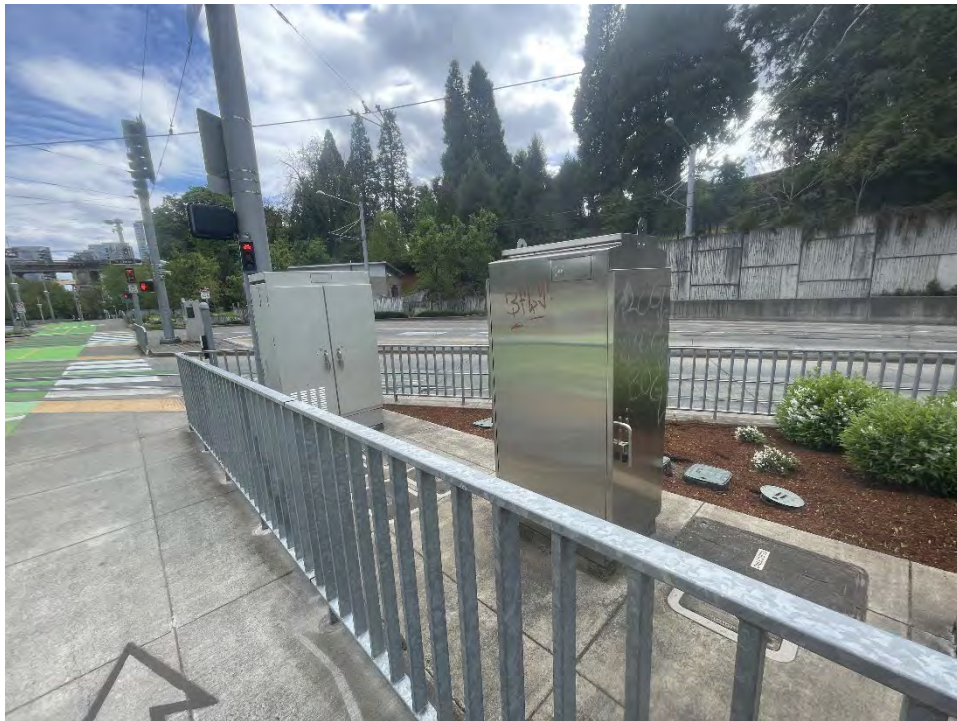
Photograph 26. TriMet light rail and storage box, looking southwest.
