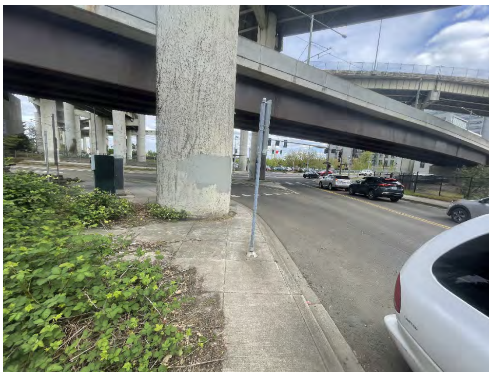
Photograph 2. Northwest corner, looking west.
