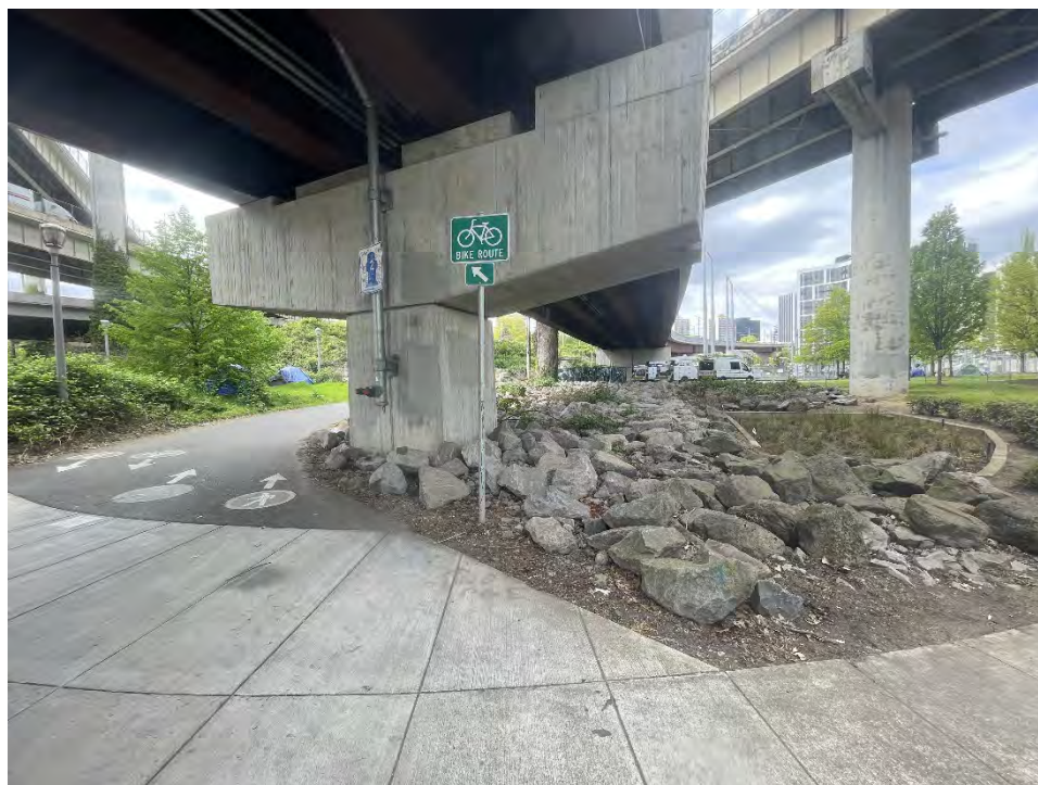
Photograph 5. Northeast corner, looking north.
