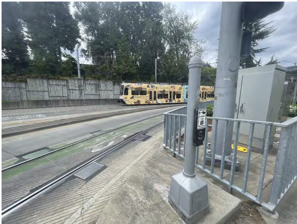
Photograph 24. TriMet light rail and storage box.
