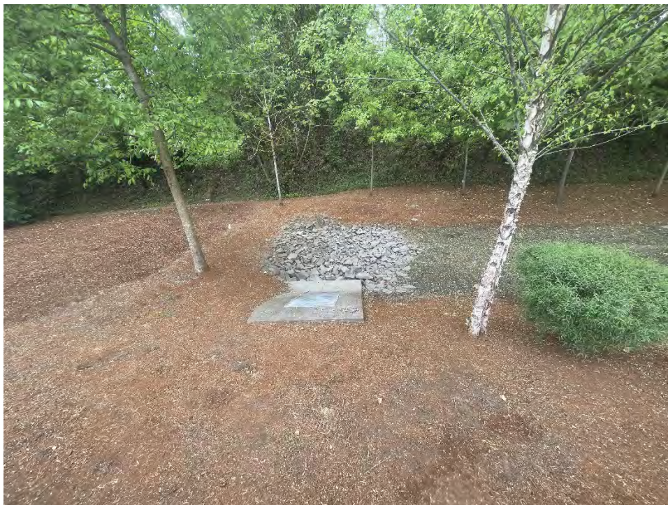
Photograph 27. Stormwater swale, looking east.
