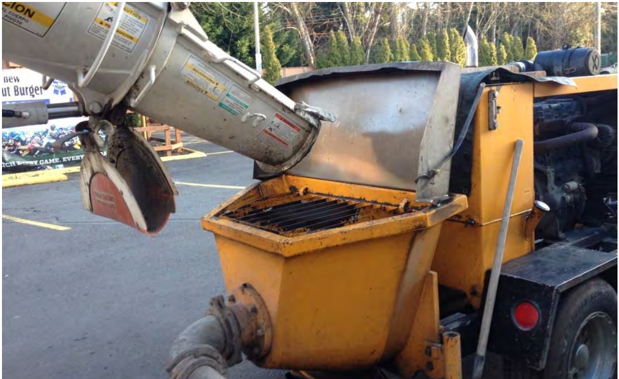
Photograph 7 – Concrete was poured from the truck to a concrete pump.
