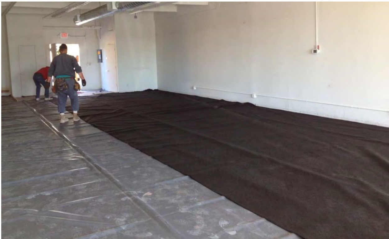
Photograph 6 – Protective geotextile fabric being placed over the PVC liner.
