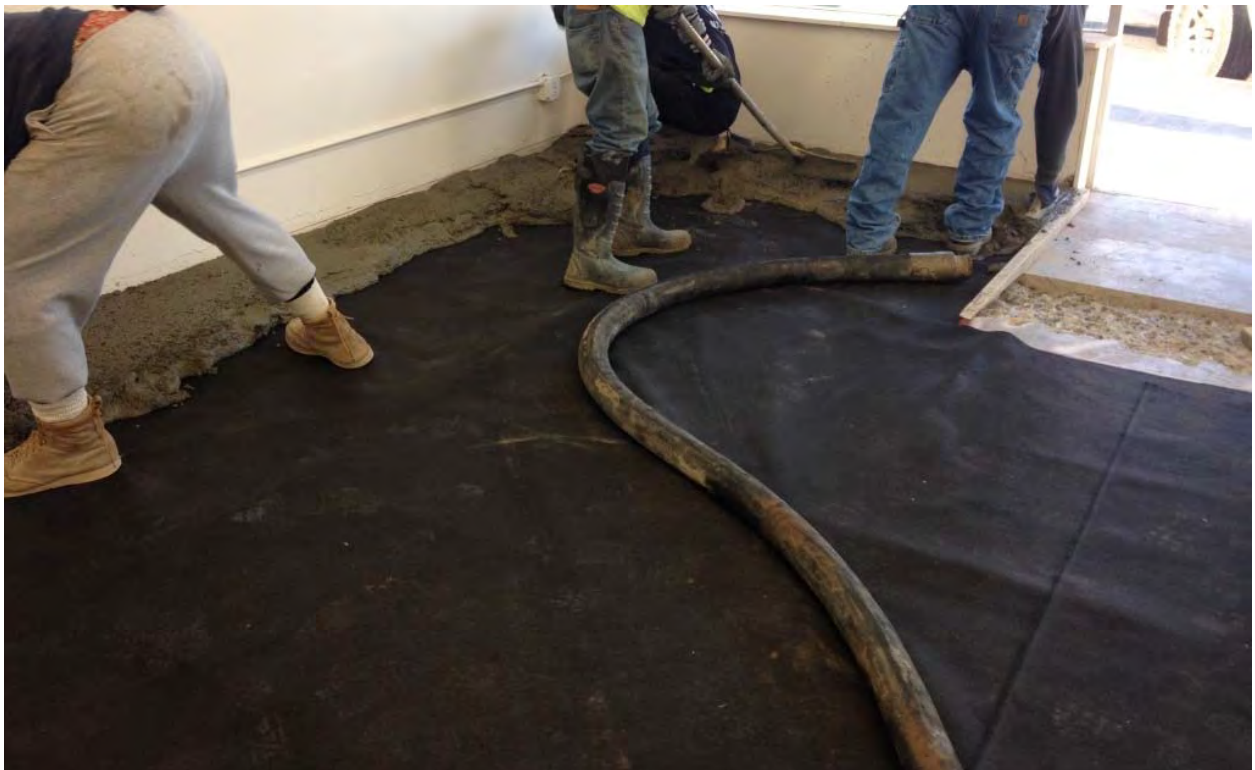
Photograph 8 – Beginning of concrete placement.
