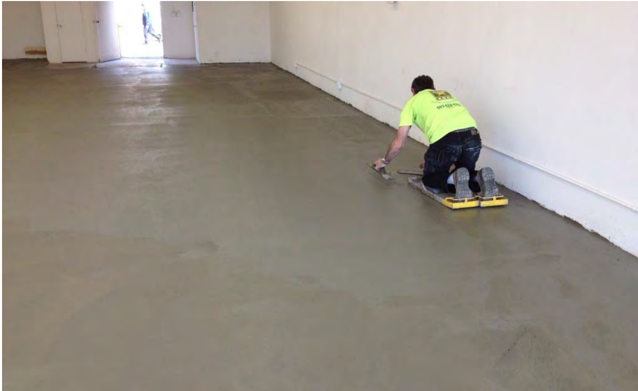
Photograph 11 – The concrete was worked multiple times until smooth.
