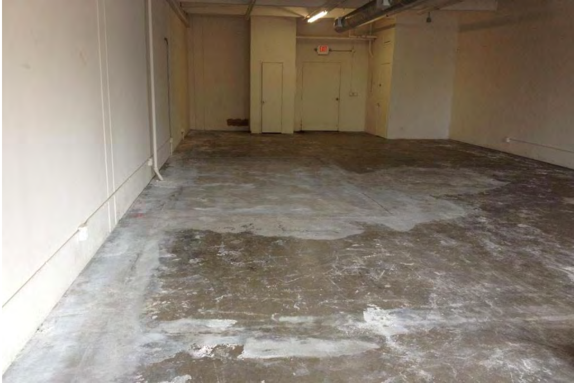
Photograph 3 – Additional photograph of the interior space to receive a vapor barrier.
