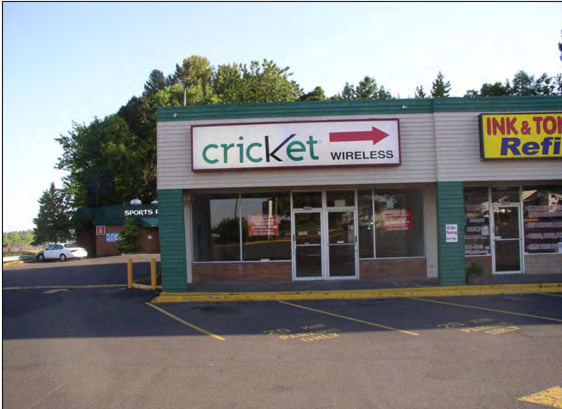
Photograph 1 - Storefront of former dry cleaner (with Cricket Wireless sign).
