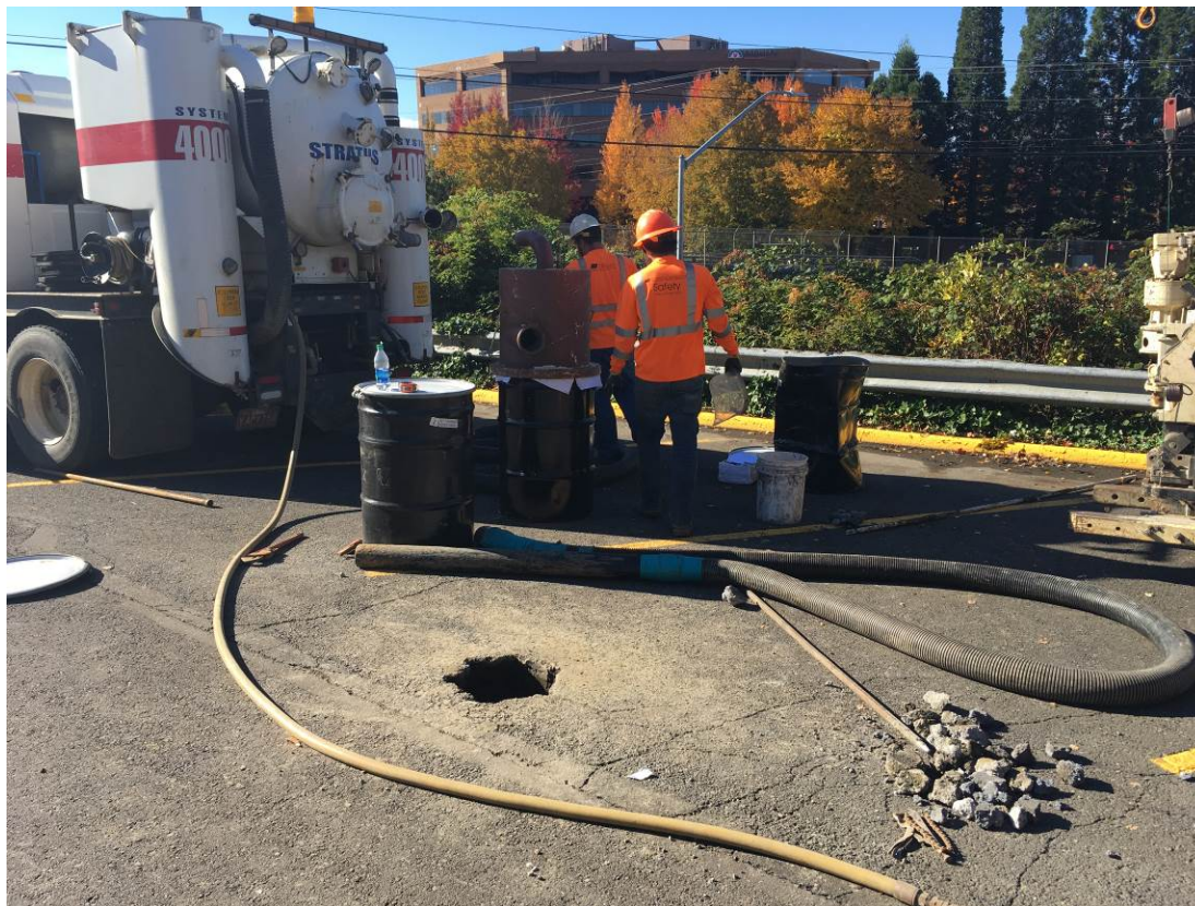
Photograph 4 – Air knifing with vacuum truck at MW-2.
