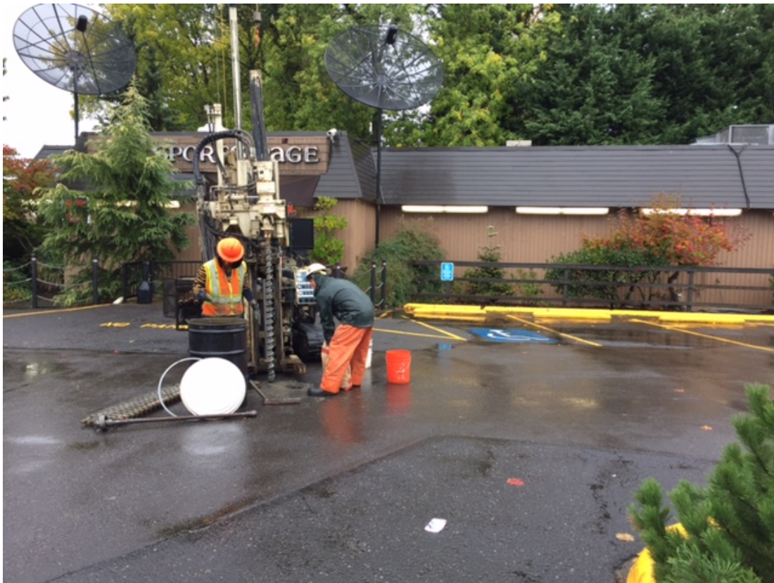
Photograph 2 – Monitoring well MW-1 abandonment.
