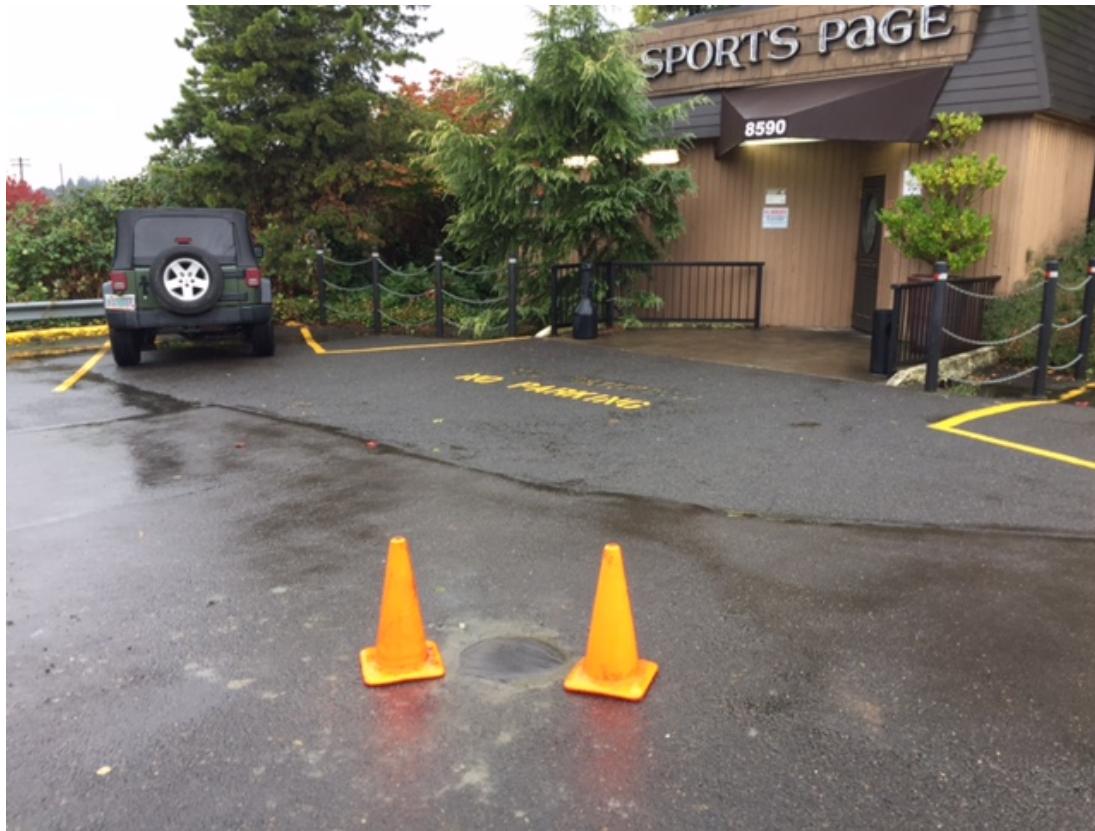
Photograph 3 – View of surface completion at monitoring well MW-1.
