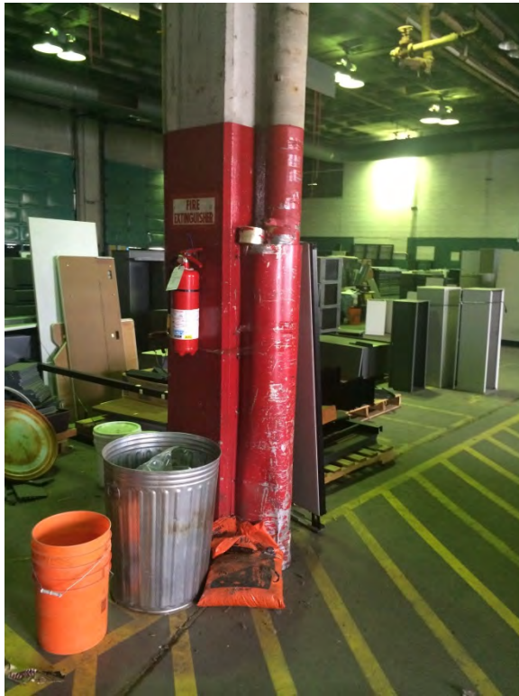
VIEWS OF A CONCRETE COLUMN AND INSULATED DRAINPIPE LOCATED IN THE WESTERN SHOP AREA. RED LEAD-BASED PAINT WAS IDENTIFIED ON THIS COLUMN.
