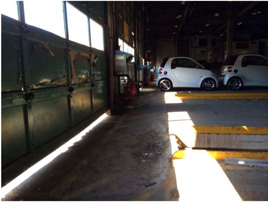
VIEW OF DIESEL PUMPS LOCATED ALONG THE SOUTH WALL OF THE EAST WING.
