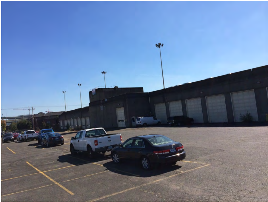
VIEW OF THE PROJECT SITE BUILDING. PHOTOGRAPH TAKEN FACING SOUTHEAST.
