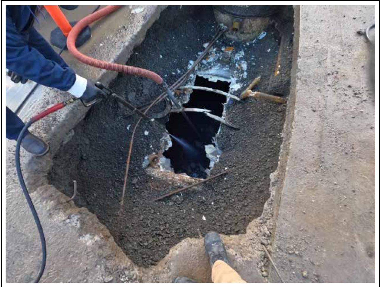
Photo 3: Tank being Cleaned
