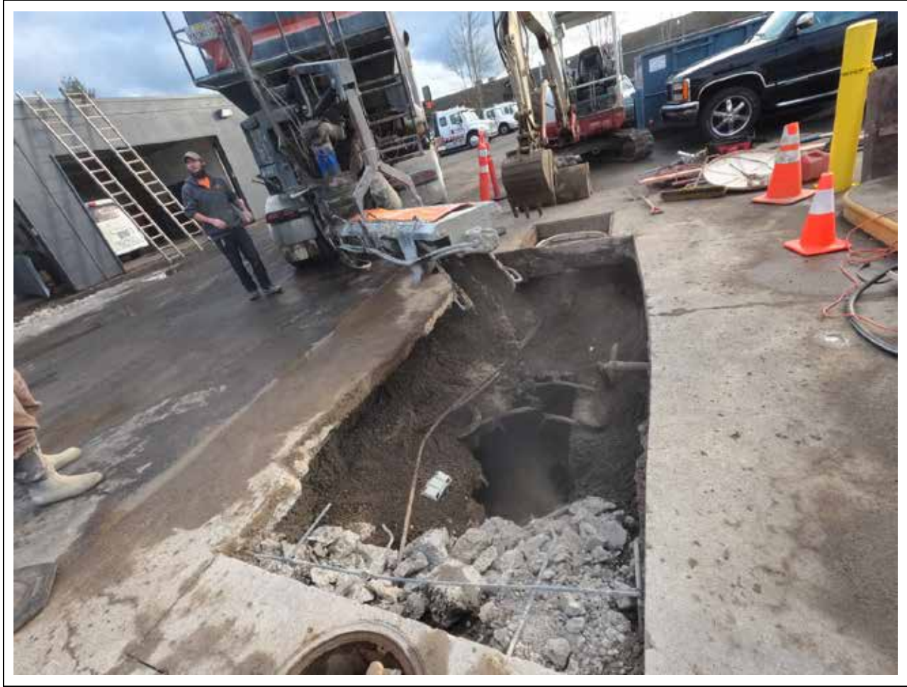
Photo 4: Tank being filled with CDF
