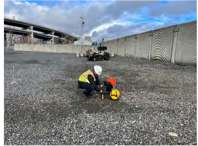
Developing one of the temporary wells.
