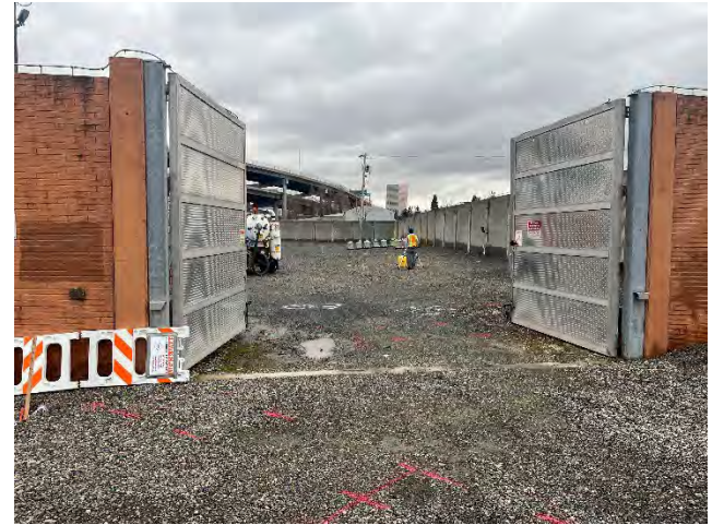
Property line being marked on PG&E property.
