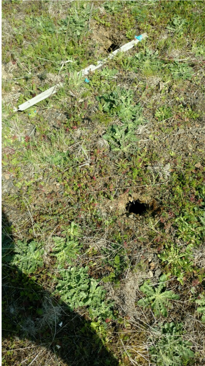
Photo 1: 04/20/2016: One of two animal burrows identified during the Annual Cap Inspection
