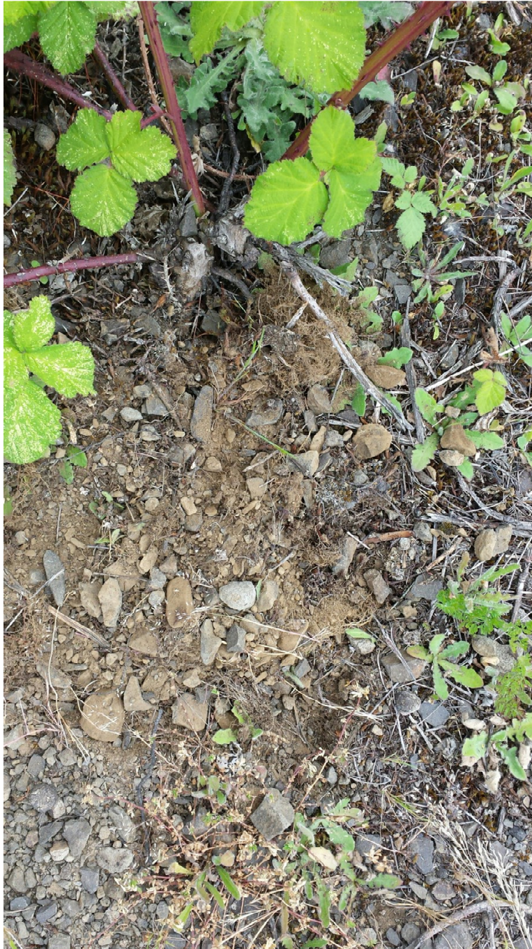
Photo 3: 05/18/2016- Photo of filled animal burrow which was identified during the annual cap inspection
