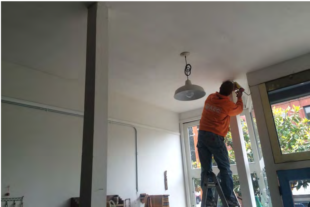
Photograph 18 – AEC crew sealing gaps in the first floor roof. Photograph taken facing south-southeast.
