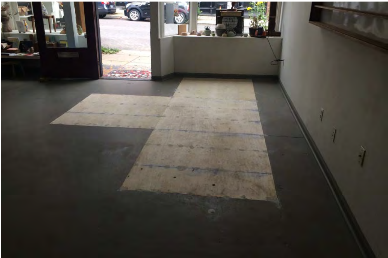
Photograph 16 – The new plywood panels installed following IRAM installation. The panels were subsequently painted by the first floor tenant. Photograph taken facing south.
