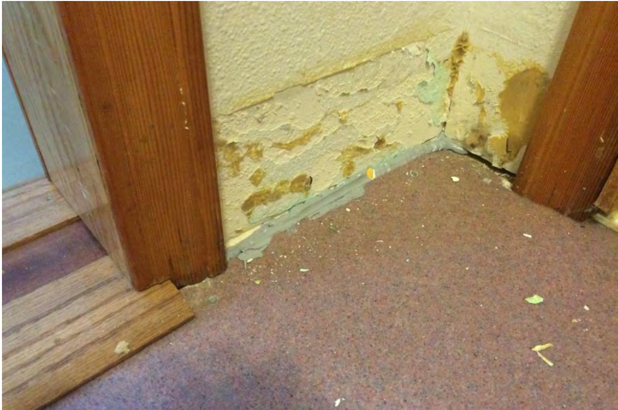
Photograph 17 – Existing rubber trim in the bathroom was removed so that gaps (potential migration pathways) could be sealed. The trim pieces were replaced following caulking.
