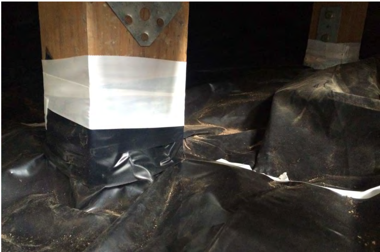
Photograph 14 – New moisture barrier secured to a building support pier using tape and epoxy sealant.
