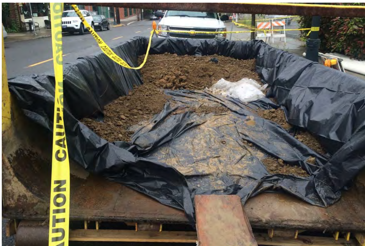
Photograph 6 – Drop box used to stage excavated soil. Ultimately 3 cubic yards of soil was excavated and disposed of at Chemical Waste Management's Subtitle C landfill in Arlington, Oregon. Photograph taken facing west.
