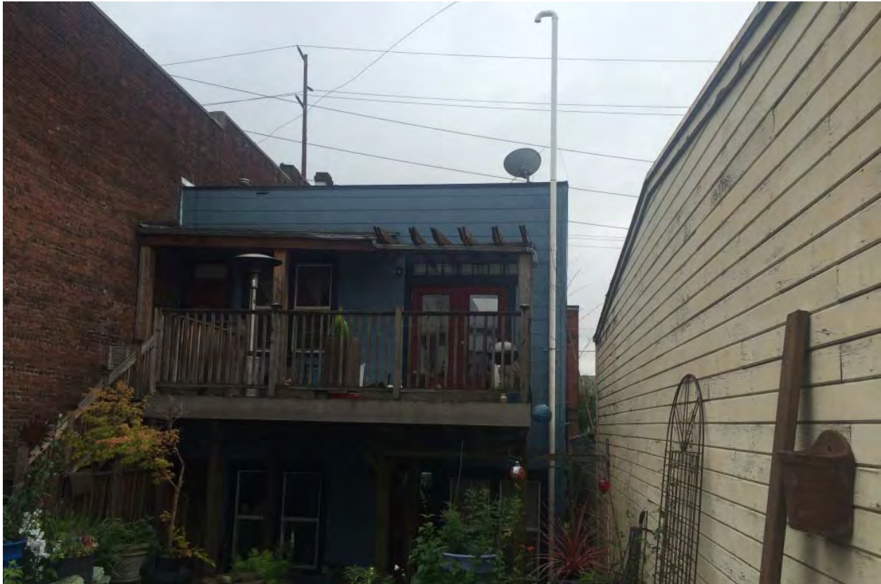
Photograph 13 – The backyard area of the site, with the exhaust stack secured to the northwest corner of the building, and venting 10 feet above the roofline. Photograph taken facing south.
