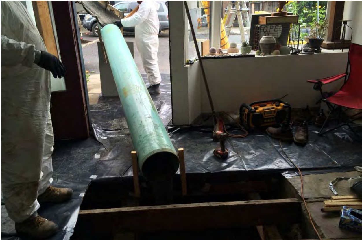
Photograph 7 – Compact density fill being placed as backfill for the source area soil excavation. Photograph taken facing south.
