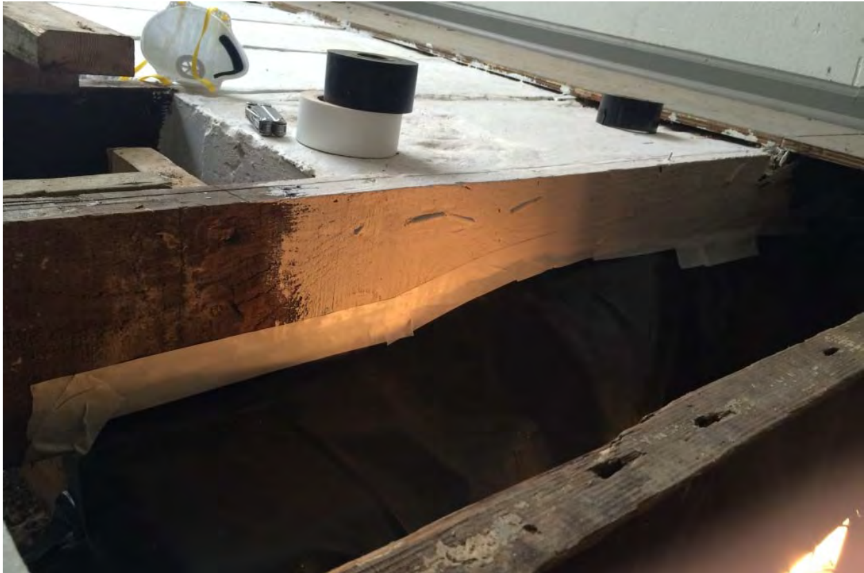
Photograph 9 – Concrete block and floor joist covered in latex sealant showing where the new moisture barrier is sealed to the joist using tape and epoxy sealant. Photograph taken facing southwest.
