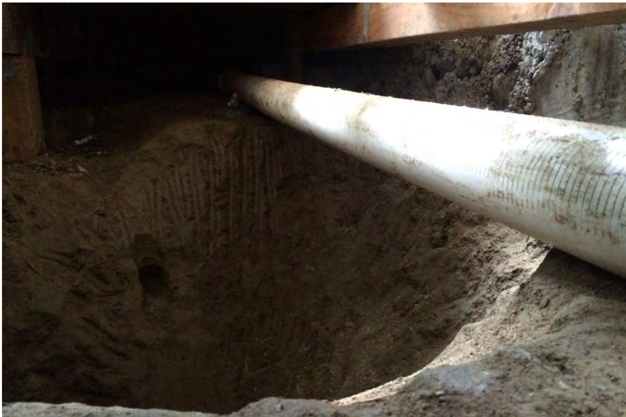
Photograph 10 –The source area soil excavation can be seen in this photograph with the slotted PVC gas collection pipe placed over it. The excavation was subsequently filled using compact density fill. Note the concrete block to the right and a building support pier to the left limiting excavation.
