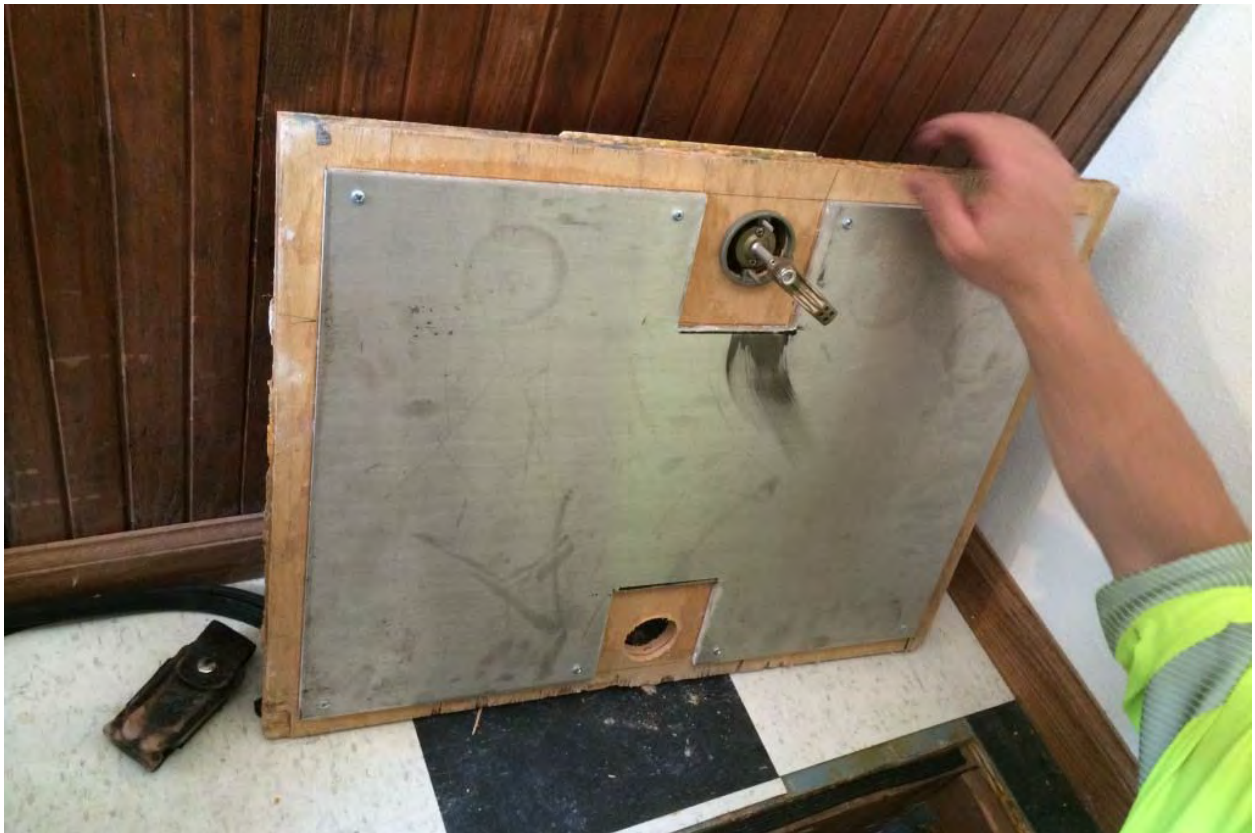
Photograph 19 – Modifications being made to the underside of the crawlspace access hatch. Including an aluminum plate and dual locking mechanisms.
