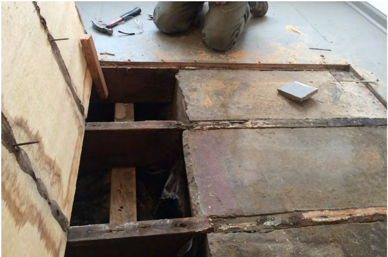
Photograph 3 – Portion of the large concrete block uncovered once the floor panels were removed.
