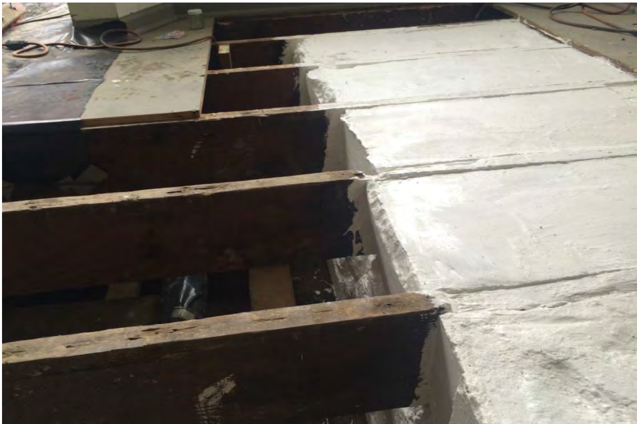
Photograph 8 – Concrete block on the right covered with latex sealant to mitigate potential off-gassing.
