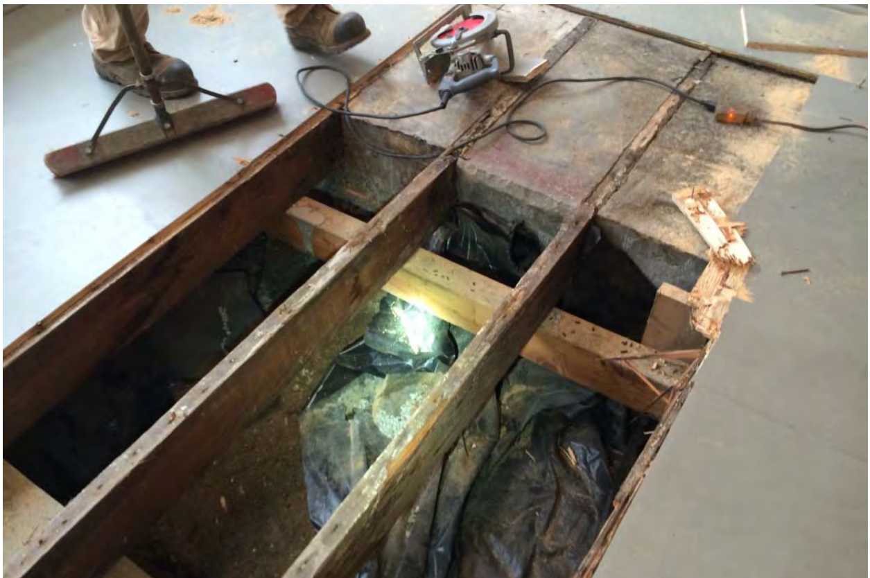
Photograph 4 – Large concrete block and the existing moisture barrier. The soil adjacent to the block was excavated as source soil.
