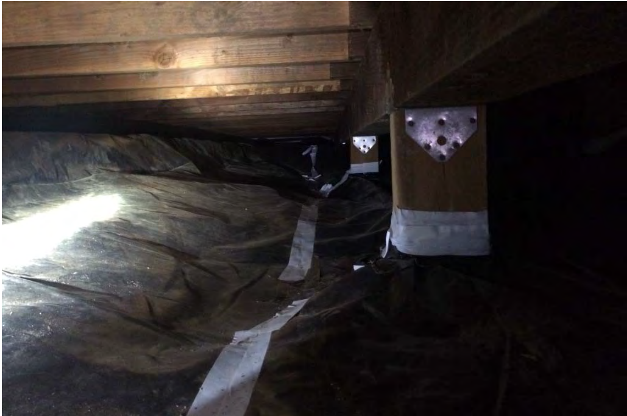
Photograph 15 – New moisture barrier installed in the crawlspace. Barrier is sealed to support piers and seams in the moisture barrier are taped together.
