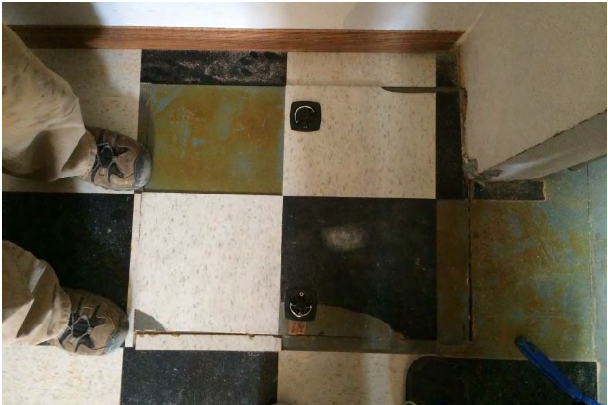
Photograph 20 – Crawlspace access hatch with flush mounted dual locking mechanisms installed.
