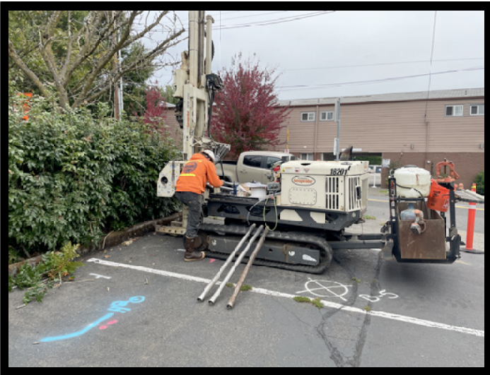
Photograph 2: Location of Phase II ESA boring P1. The location of geotechnical boring B-5 is indicated with white spray paint. Photo taken facing north. N Overlook Blvd is in the background.
