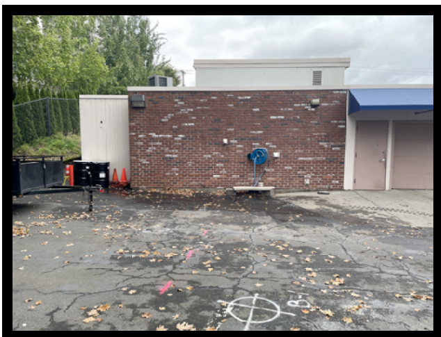
Photograph 12: View facing north of the former waste oil tank area on the south side of the Subject Property building. The spray painted location of geotechnical boring B-1 was moved further east than shown to avoid potential utility conflicts.
