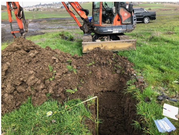
3. Test Pit TP14.
