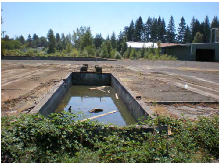
PHOTO 6 Former Dip Tank #2 concrete containment vault prior to rainwater and debris removal.
