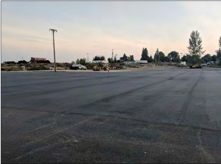
PHOTO 29 Completed paving. View to the northwest.
