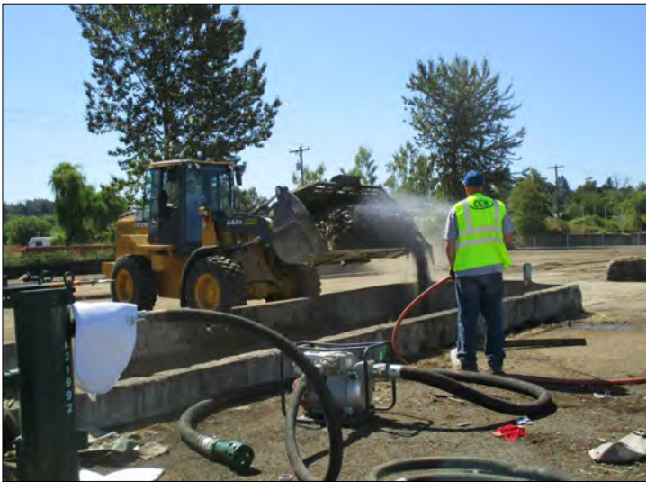
PHOTO 8 Placement of soil fill in Former Dip Tank #2 concrete containment structure.
