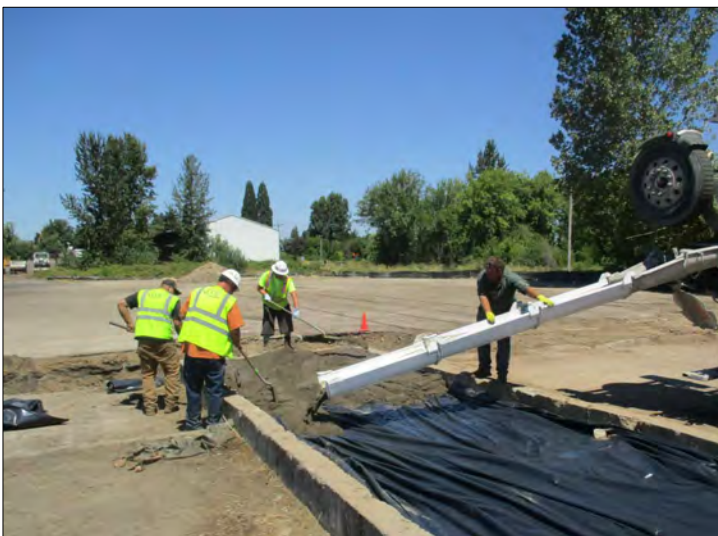
PHOTO 9 Placement of concrete cap over fabric and soil fill in Former Dip Tank #2 concrete containment vault.
