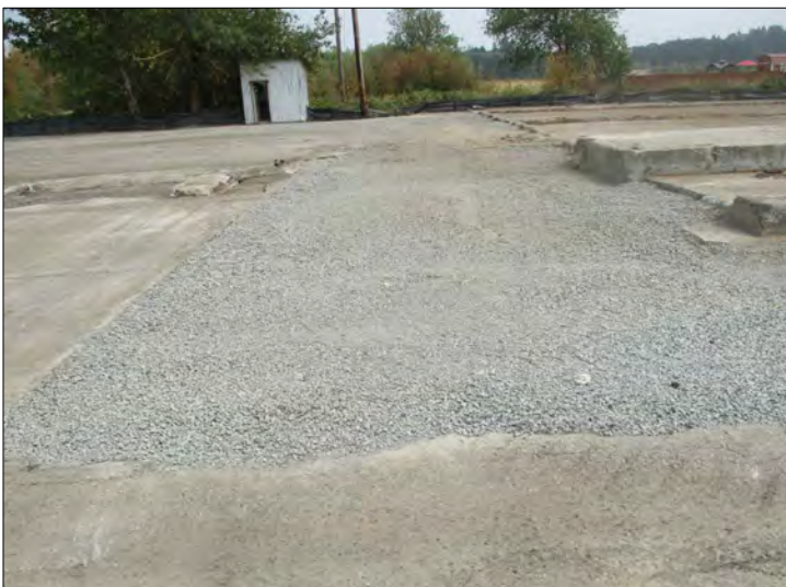
PHOTO 21 Hot spot soil excavation after backfill placement. View from the west.
