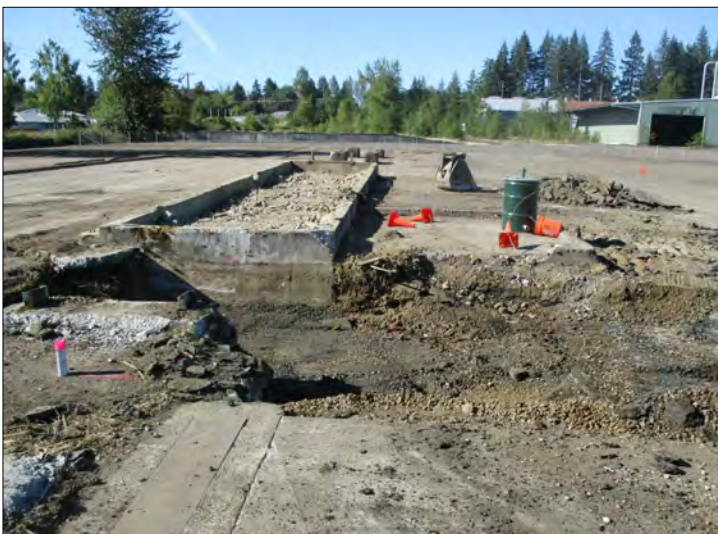
PHOTO 18 Hot spot excavation. View from the north.
