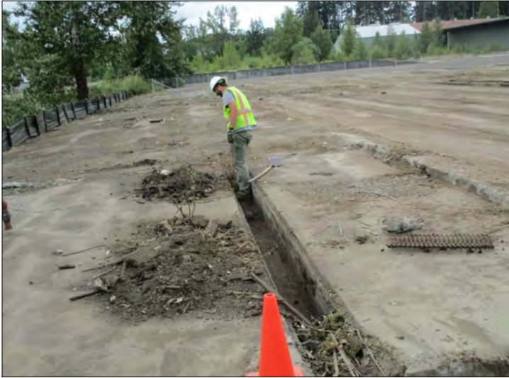
PHOTO 25 Debris cleaning, existing concrete surface preparation for asphalt concrete overlay placement.
