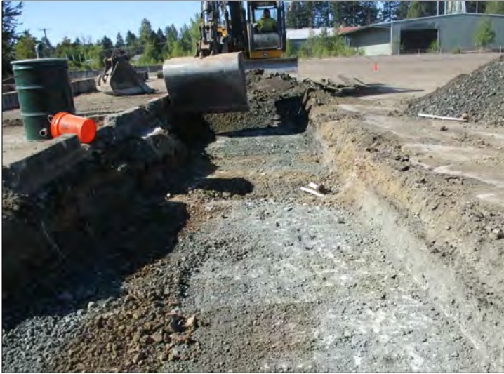
PHOTO 19 Hot spot excavation. View from the north.
