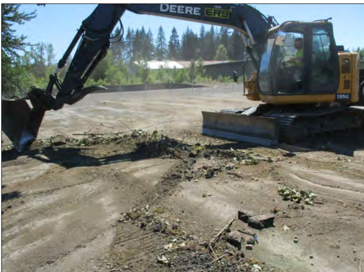
PHOTO 24 Debris cleaning, existing concrete surface preparation for asphalt concrete overlay placement.
