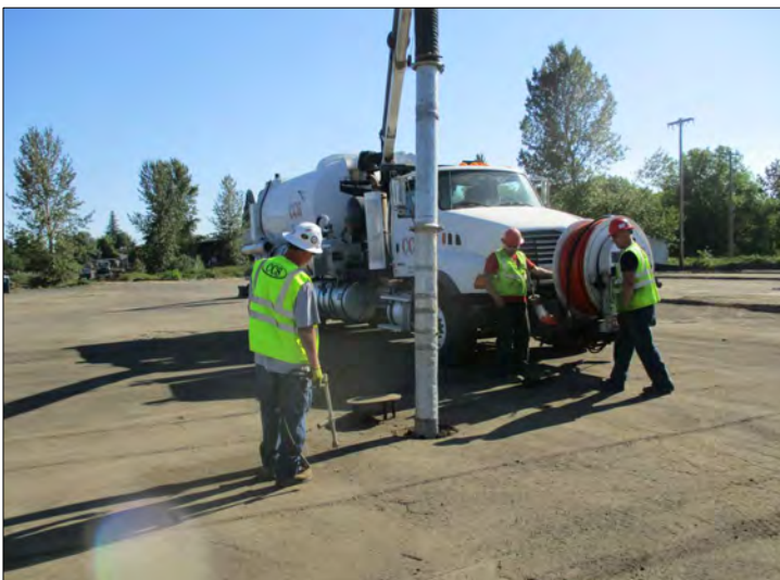
PHOTO 3 Removal of sediment water slurry from catch basin with vacuum truck.
