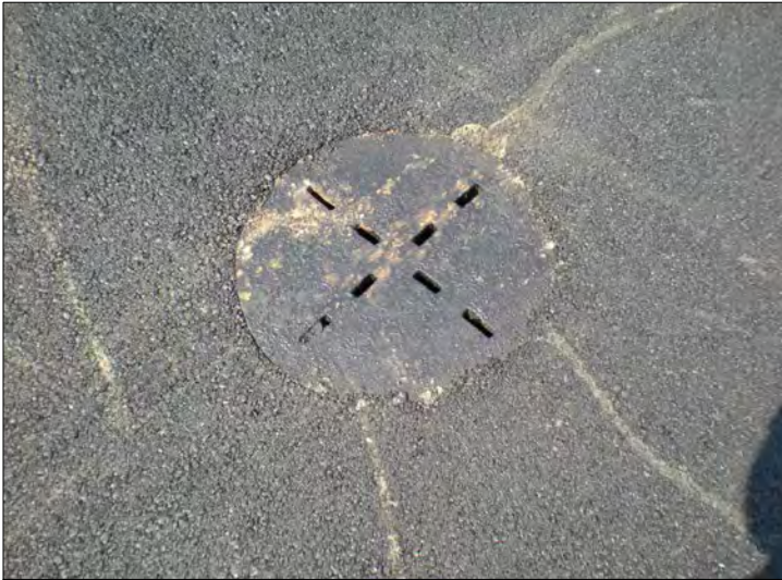
PHOTO 5 Catch basin cover final.
