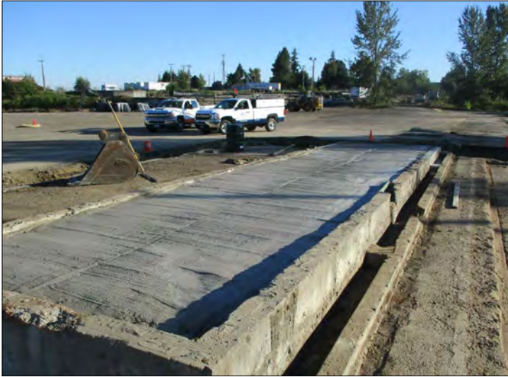
PHOTO 10 Finished concrete cover on Former Dip Tank #2 concrete containment vault.
