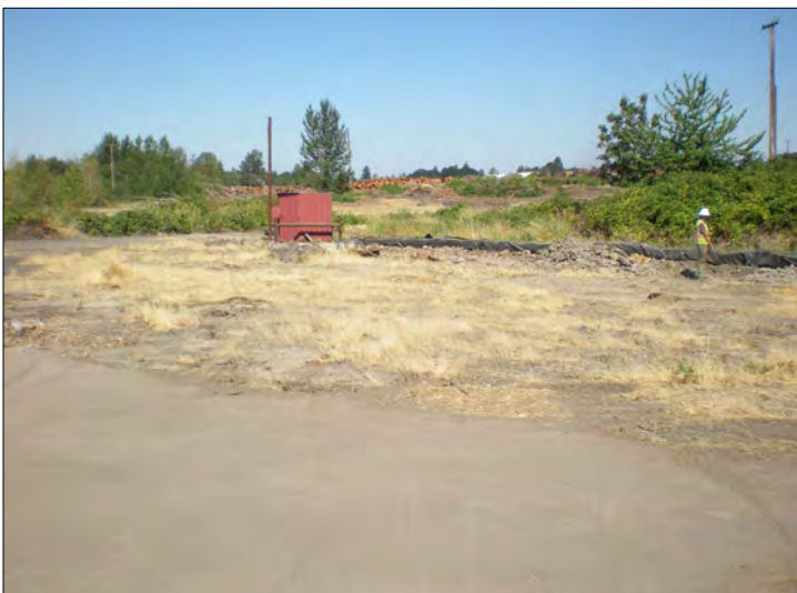
PHOTO 12 Western habitat area surface preparation.
