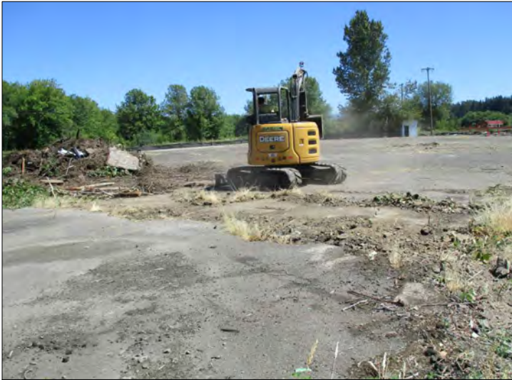
PHOTO 23 Debris cleaning, existing concrete surface preparation for asphalt concrete overlay placement.
