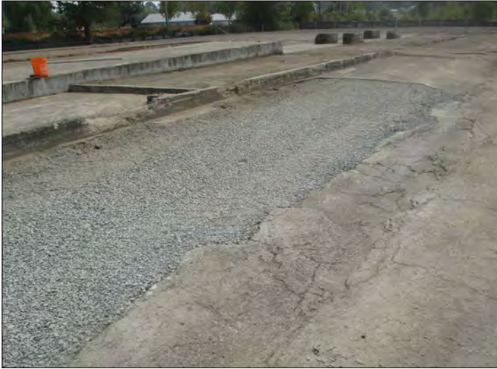
PHOTO 22 Hot spot soil excavation following backfill placement. View from the northwest.
