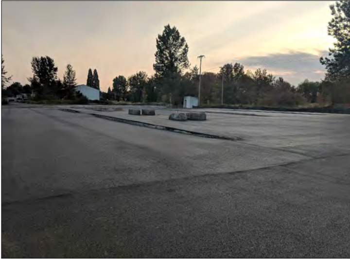
PHOTO 28 Completed paving. View to the northeast.
