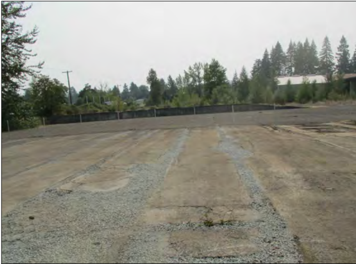
PHOTO 26 Following placement of gravel fill surface preparation for paving.
