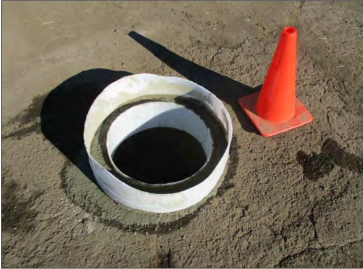
PHOTO 4 Cleaned catch basin.
