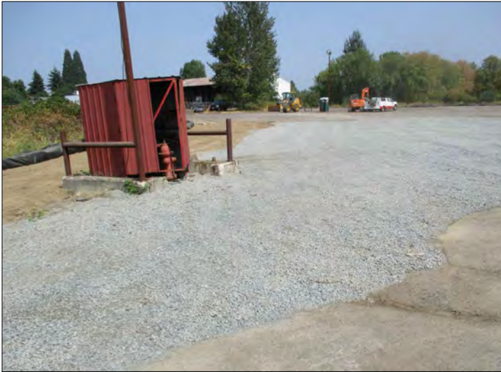
PHOTO 14 Western habitat area after topsoil and gravel placement.
