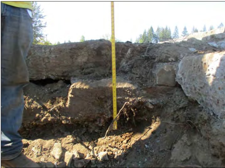
PHOTO 20 Hot spot soil excavation final depth.
