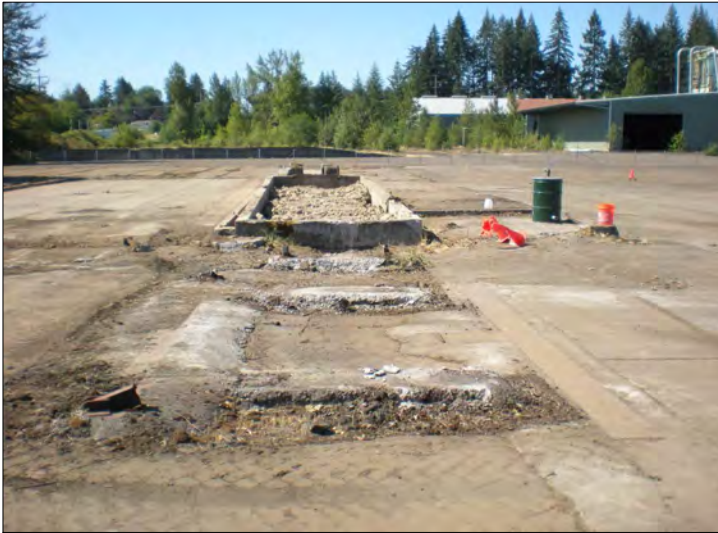
PHOTO 17 Hot spot soil area prior to excavation. View from the north.
