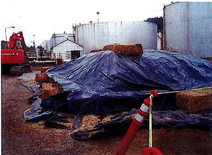
Dirt collection area 7/28/11
