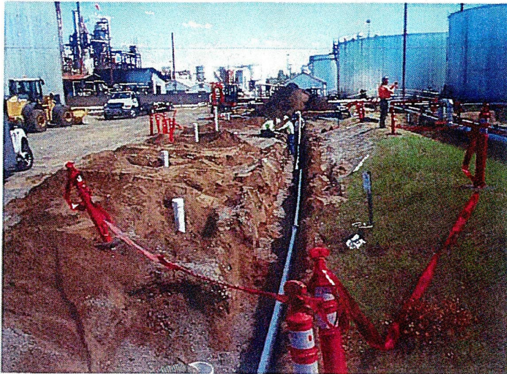
SVE trench inside of recovery wells 7/27/11
