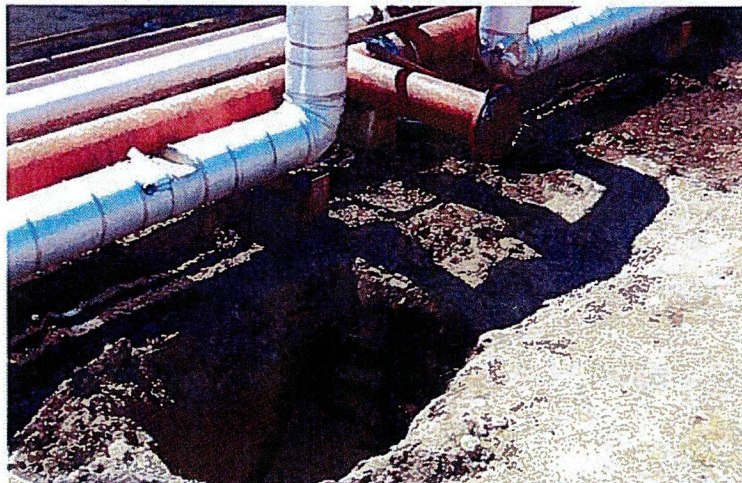
Hot Zone Test Hole 7/21/11
