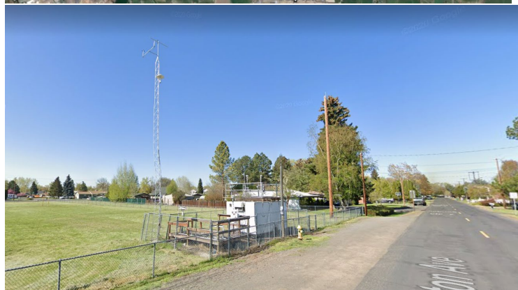
Klamath Falls KFP Air Monitoring Station.
