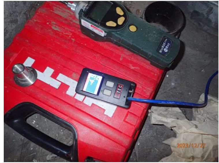
Communication testing was performed at all communication test ports to confirm negative pressure-field extension beneath the slab.
