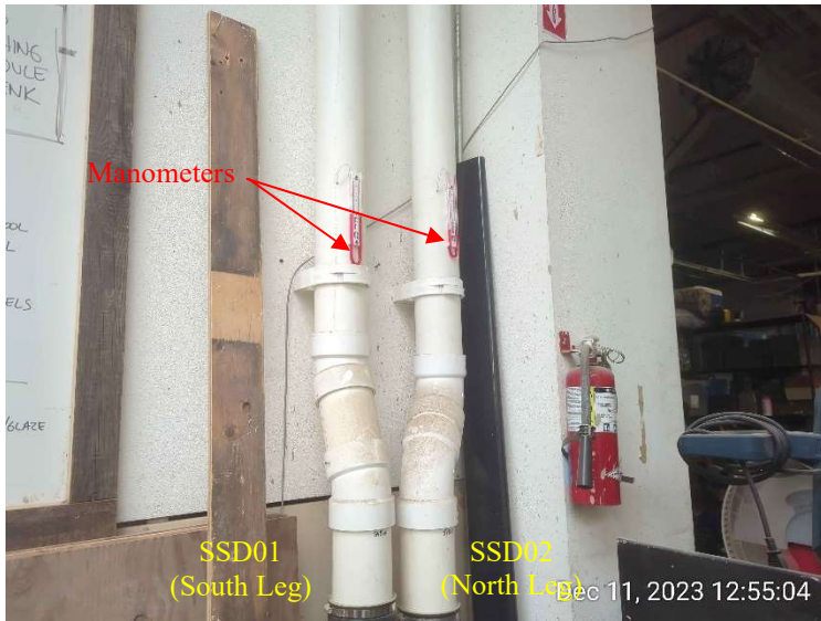
Interior portion of vent risers, note U-tube manometers on each vent riser to provide visual confirmation of system operation.
