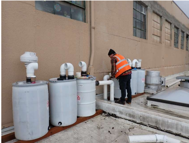
Positioning the granular activated carbon (GAC) units in preparation for activating the sub-slab depressurization (SSD) system.
