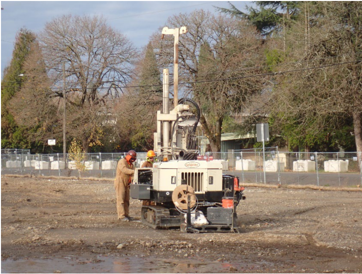
On November 19 and 30, 2023, a direct-push drill rig was used to advance borings EB01 through EB10.
