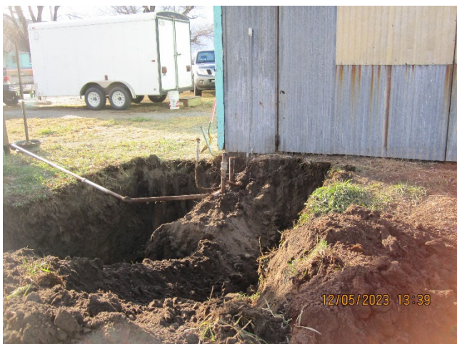
Photo 5: Concrete pad has been removed and UST is exposed.
