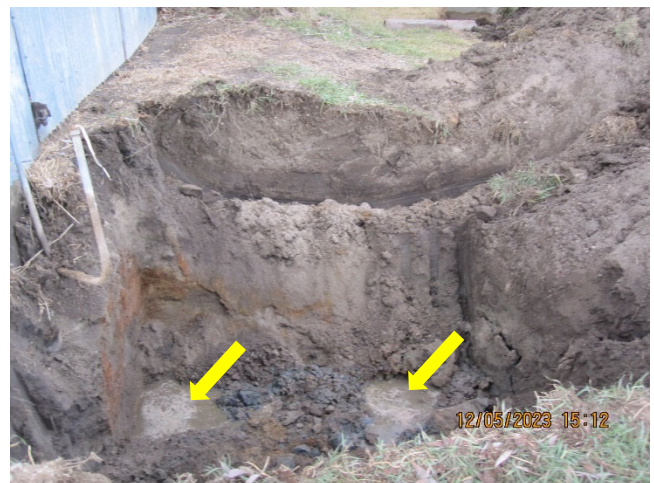
Photo 16: View of excavation before backfilling. Arrows point to soil sample locations.
