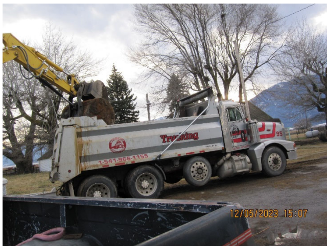
Photo 15: EOER is placing UST in dump truck for transport to EOER's Pendleton yard.
