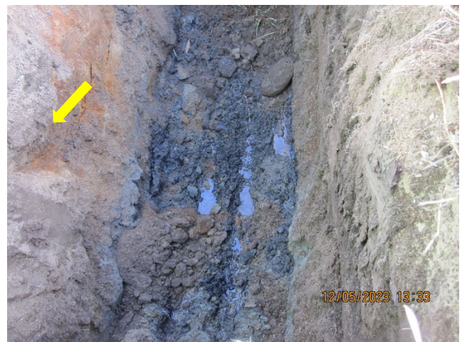
Photo 4: Looking down into excavation; sheeny shallow groundwater is visible. Arrow points to UST.
