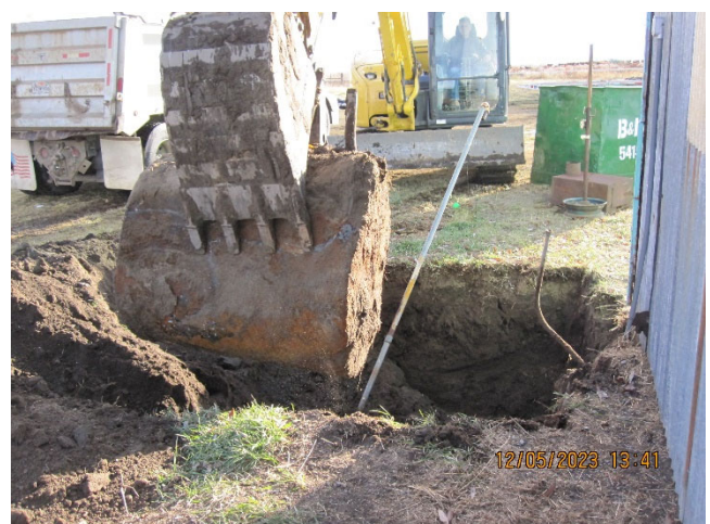
Photo 6: EOER is removing UST from excavation with excavator bucket.
