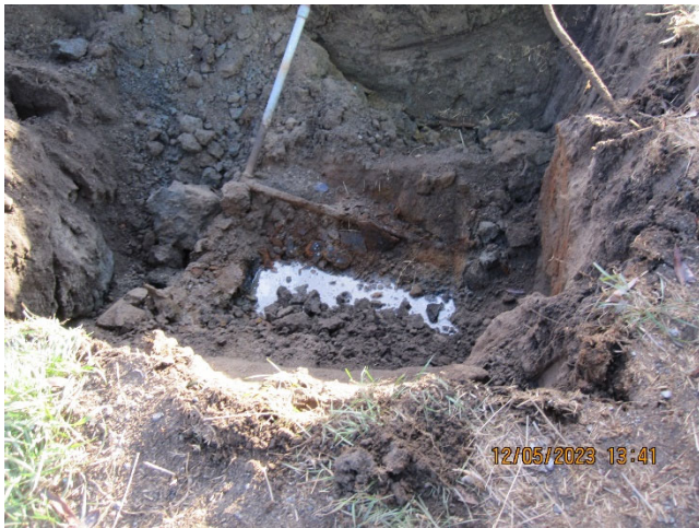
Photo 7: Looking down into excavation after UST was removed.
