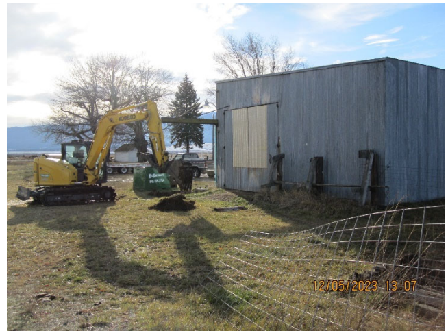
Photo 2: Looking southwesterly; excavator starting to uncover unregulated UST.
