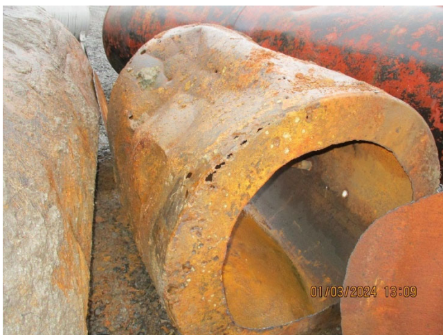
Photo 17: Looking at exterior of UST after being cleaned by EOER. Photo provided by EOER.
