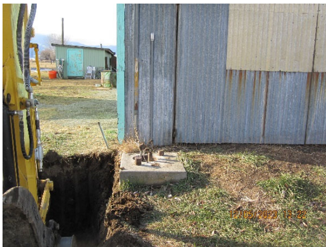
Photo 3: Looking westerly while excavating along the side of UST.
