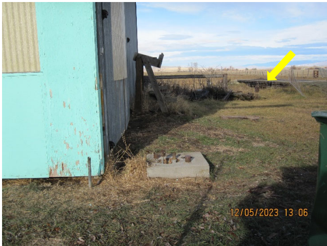
Photo 1: Looking north at concrete pad for former pump. Shop to left; arrow points to bridge over Rock Creek.
