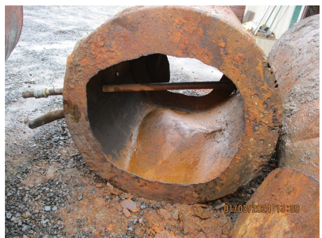
Photo 18: Looking at interior of UST after being cleaned by EOER. Photo provided by EOER.
