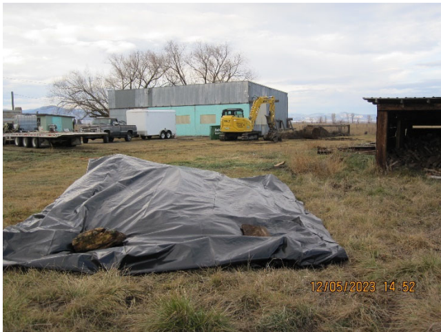
Photo 13: Looking northerly at covered stockpile, shop in background by excavator.
