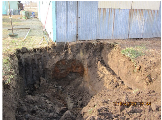
Photo 8: Looking across excavation after UST was removed.
