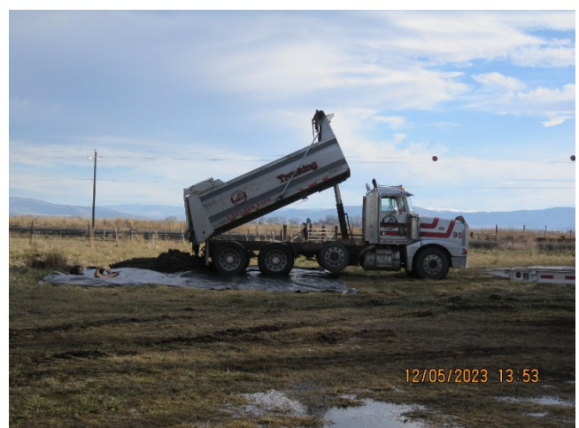
Photo 12: Stockpile on visqueen is from HOT. EOER is adding 3 buckets of impacted soil from UST pit.
