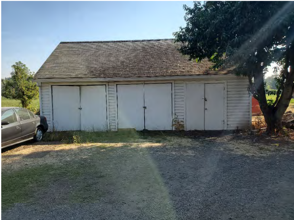
View of equipment storage building (locked), looking east.
