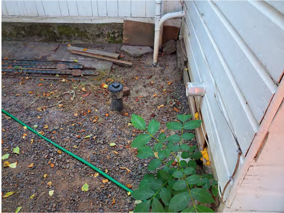
A third apparent sewer cleanout pipe north of duplex.
