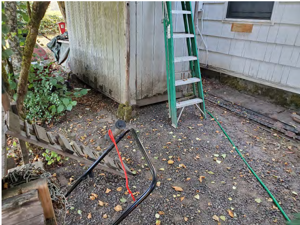
View of apparent sewer cleanout pipe on north side of duplex.
