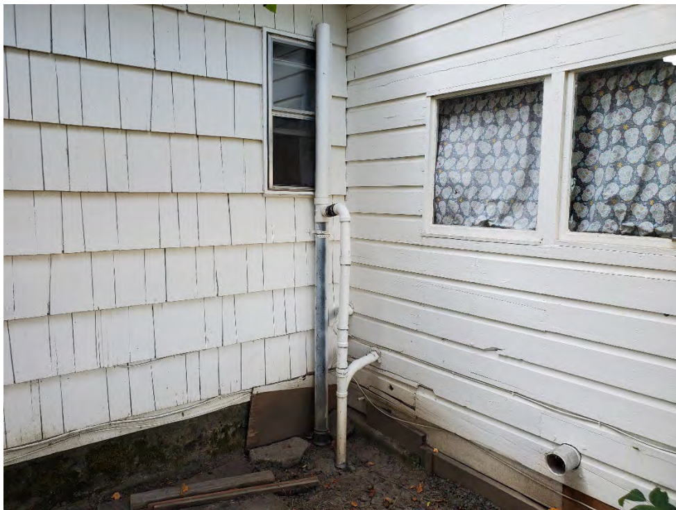
View of utility pipe with vent on north side of duplex.
