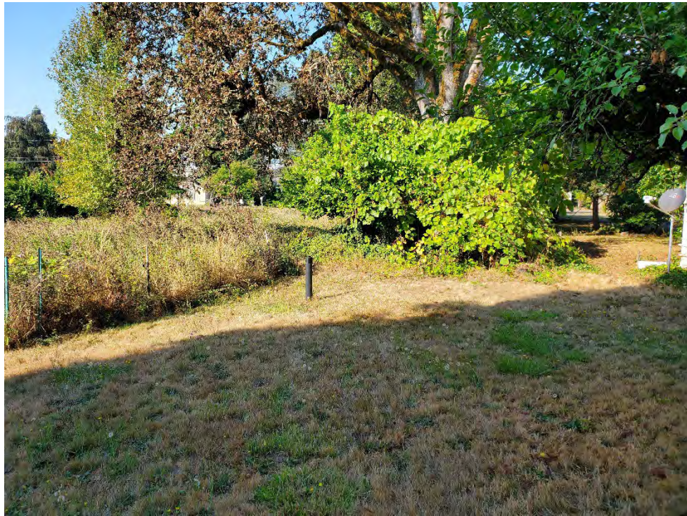
View of apparent sewer cleanout pipe south of farmhouse.
