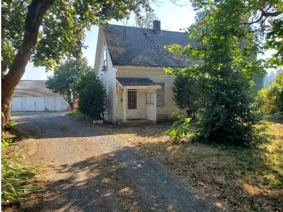
View of equipment storage building (behind farmhouse) and farmhouse, looking east.
