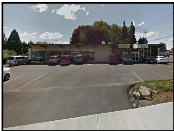
PHOTOGRAPH NO. 1 – Front view of building.
