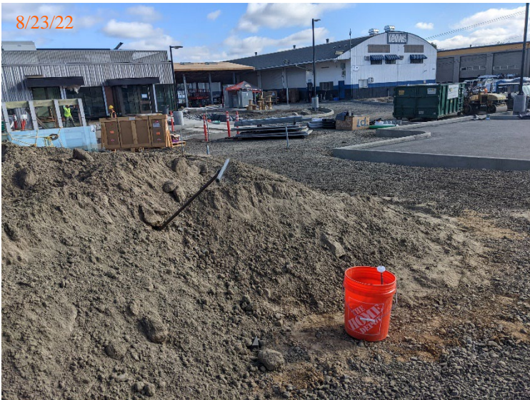
A decontaminated stainless-steel hand auger was used to collect sample increments.
