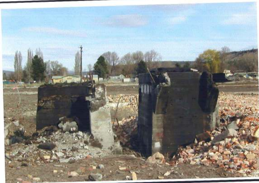
View of heavily stained foundations and soil at the former Powerhouse.
