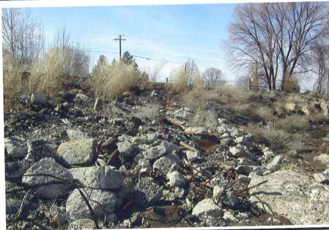
Detailed view of concrete rubble used as log pond fill materials.
