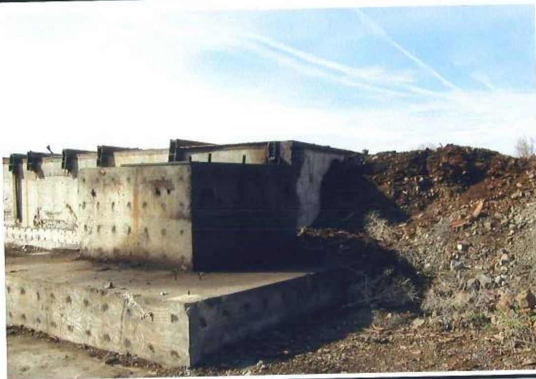
Detailed view of heavily stained concrete at former Small Log Mill debarker.
