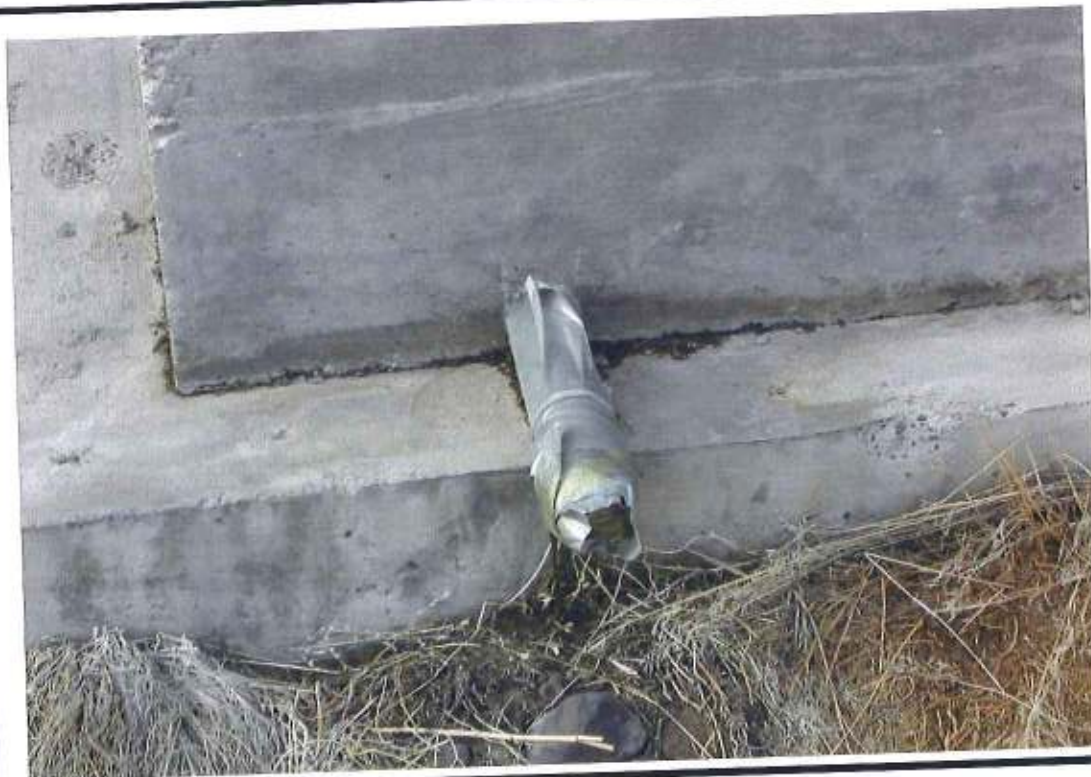
View of stormwater drain covered with duct tape at the AST containment basin.
