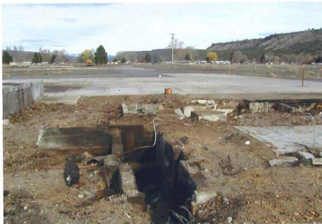
View of heavily stained foundations and soil associated with the main Planner Drive Gear in the former Planner Building.
