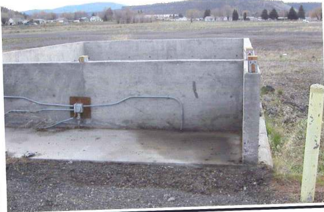
View of stained soil suspected to be associated with product overfilling at the AST concrete containment basin.
