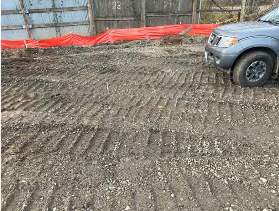
IMAGE 1: Import after bucket compaction and trackwalking, but prior to proofroll.
