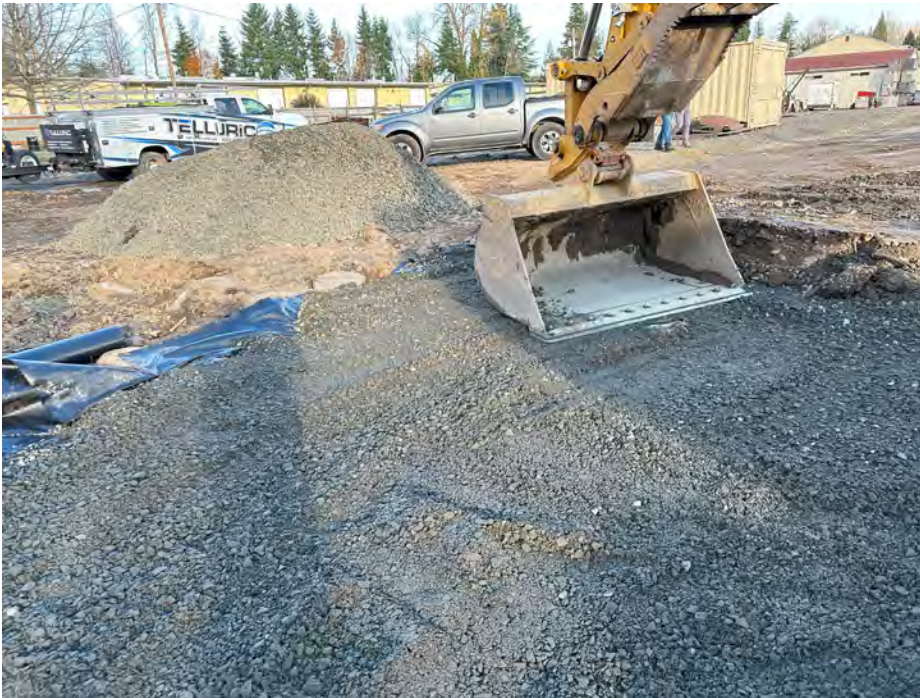
IMAGE 1: Water management completed prior to compaction efforts.
