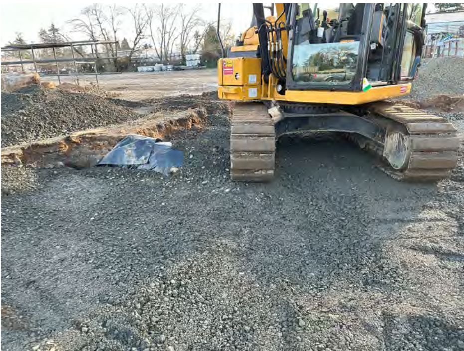
IMAGE 2: Track Walking and bucket compaction of import.
