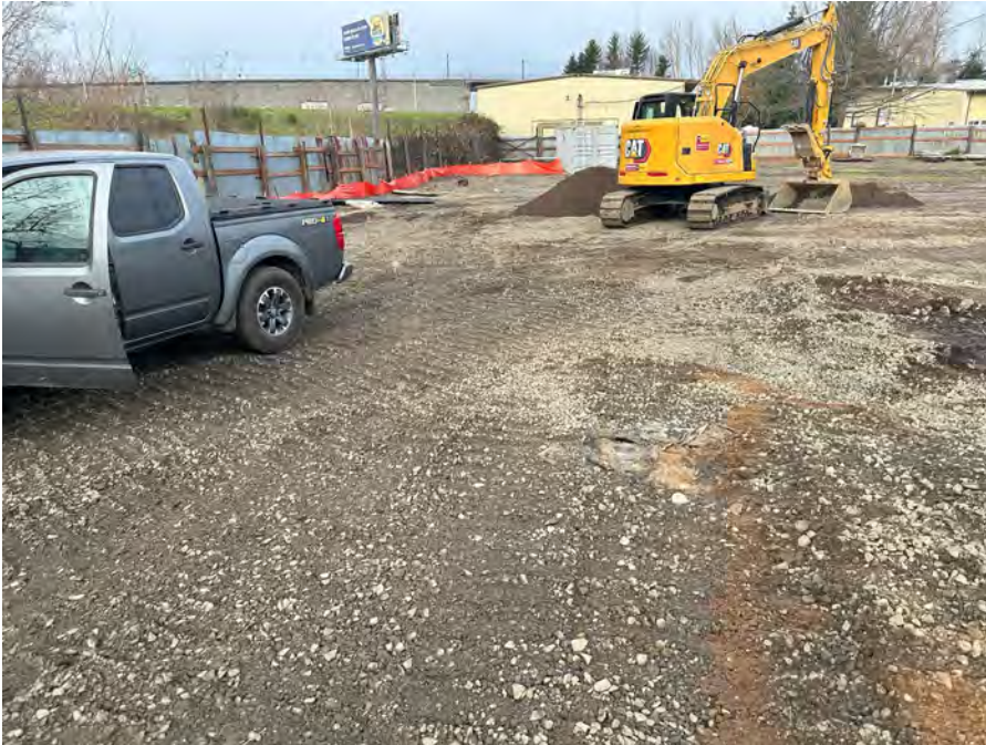
IMAGE 1: Import after bucket compaction and trackwalking, but prior to proofroll.
