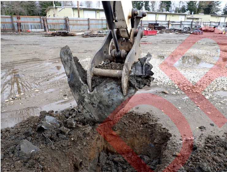
Metal, plastic, and rubber debris was encountered in the upper two feet of the test pit exploring a suspected infiltration pit (MA25).
