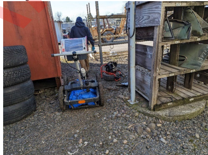
View of circular concrete cover capping a drywell (UIC) on the south side of the main warehouse building (MA03), view south. The shelving was subsequently moved to provide access for drilling.
