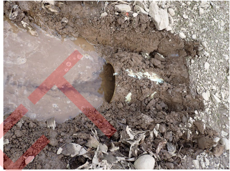
An 8-in ABS pipe was exposed on the east side of the suspected infiltration pit. Water was present in the pipe and pit.
