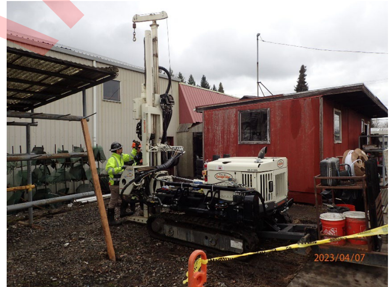
Drill rig set up at EB06 adjacent to the UIC at the site. Soil and reconnaissance ground water samples were collected from this boring.
