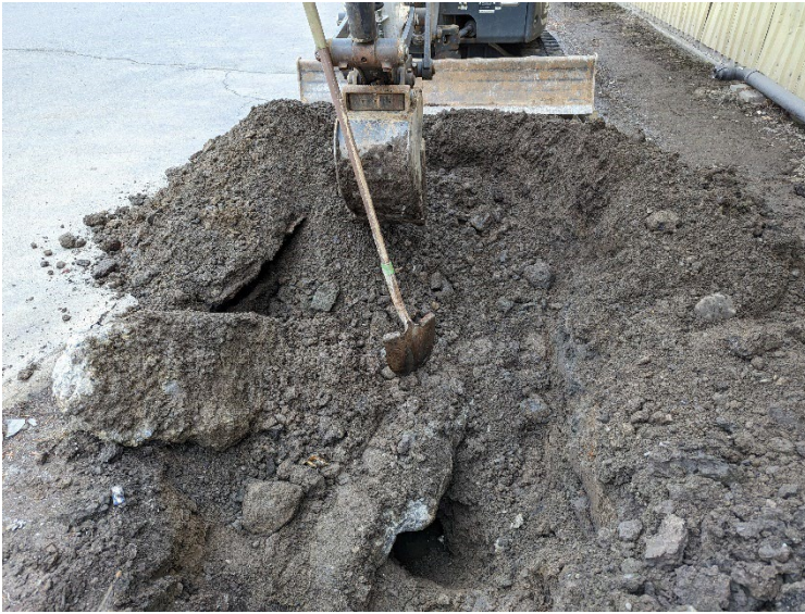
Excavation of MA02 near the NE property margin. Observations were suggestive of an old septic tank.
