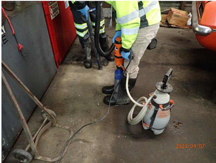
Coring through the concrete slab at EB07 next to the used oil ASTs in the southeast part of the shop building.
