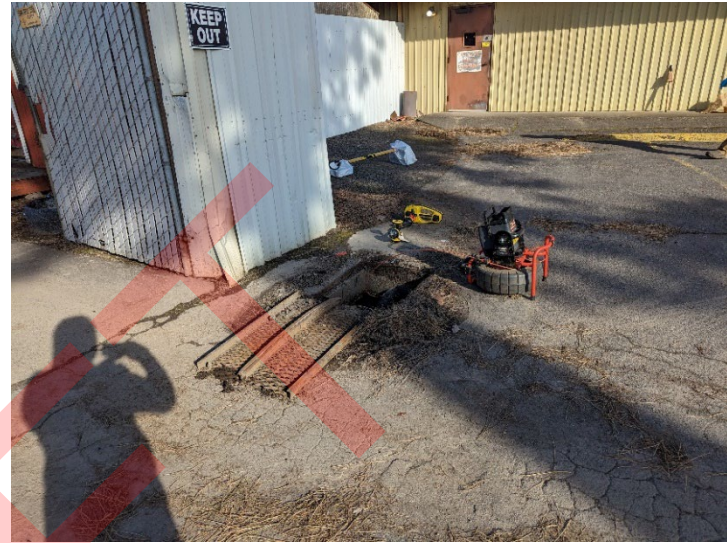
The catch basin on the south side of the building (MA01) was investigated using a SeeSnake downhole camera to confirm point of discharge.
