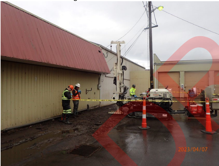
Cascade Drilling's direct-push drill rig advancing boring EB01 at the west end of the suspected septic tank near the NE property margin.
