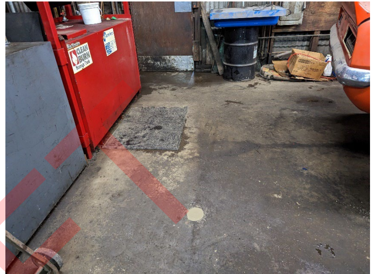
After sampling, the core hole was patched with concrete.
