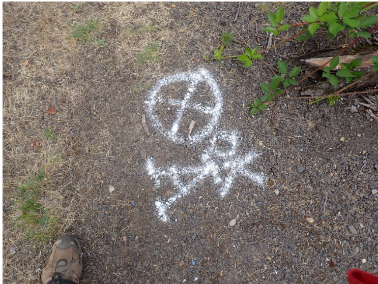
Cleared boring location.
