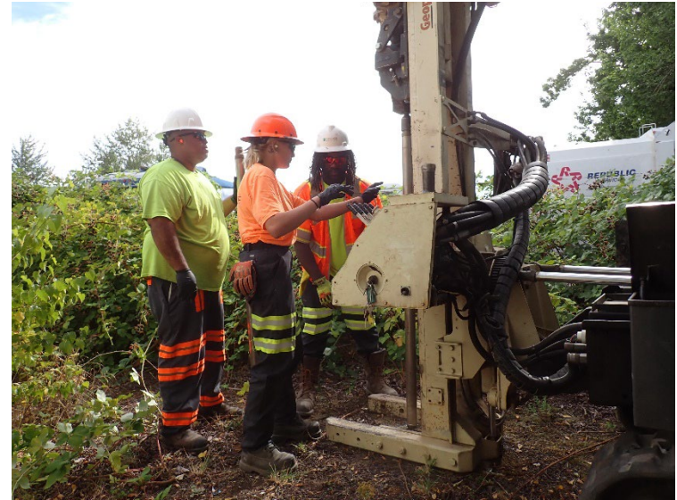
Direct-push drill rig set up at B24 on the east side of the warehouse.
