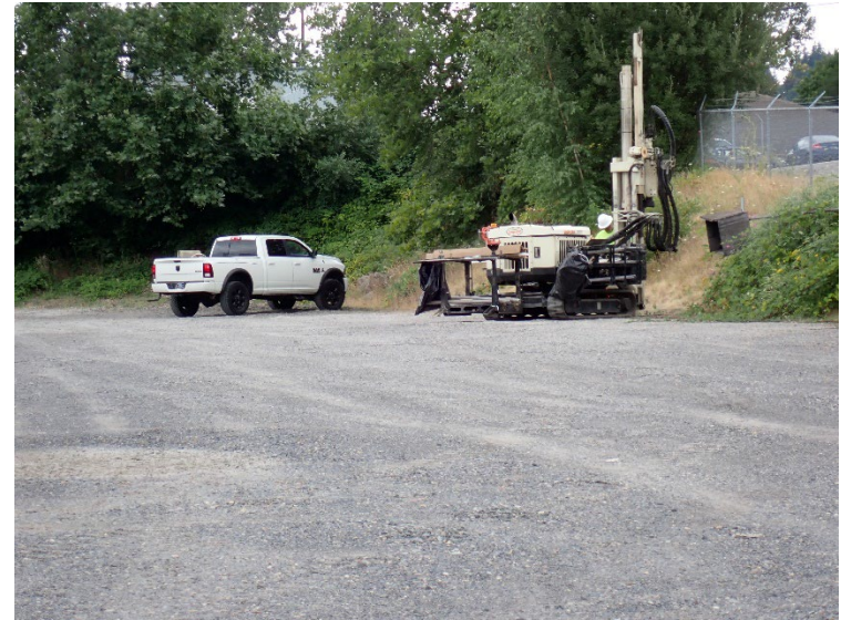
Drill rig set up at B22 along the western property margin.
