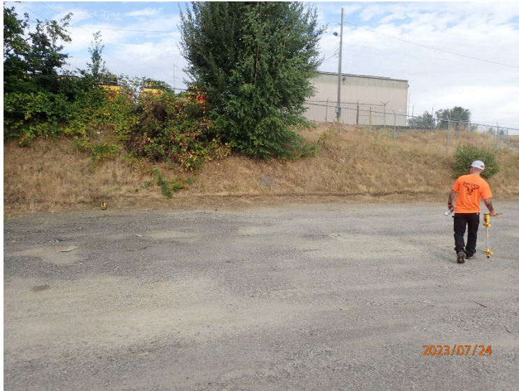
Private locator clearing boring locations of utilities.
