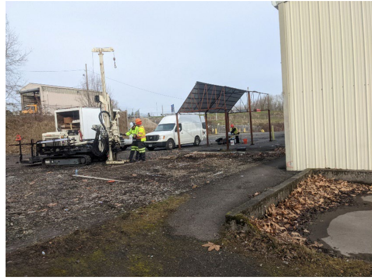
View of direct-push (DPT) drill rig installing a temporary boring for the purpose of sampling soil and reconnaissance ground water.
