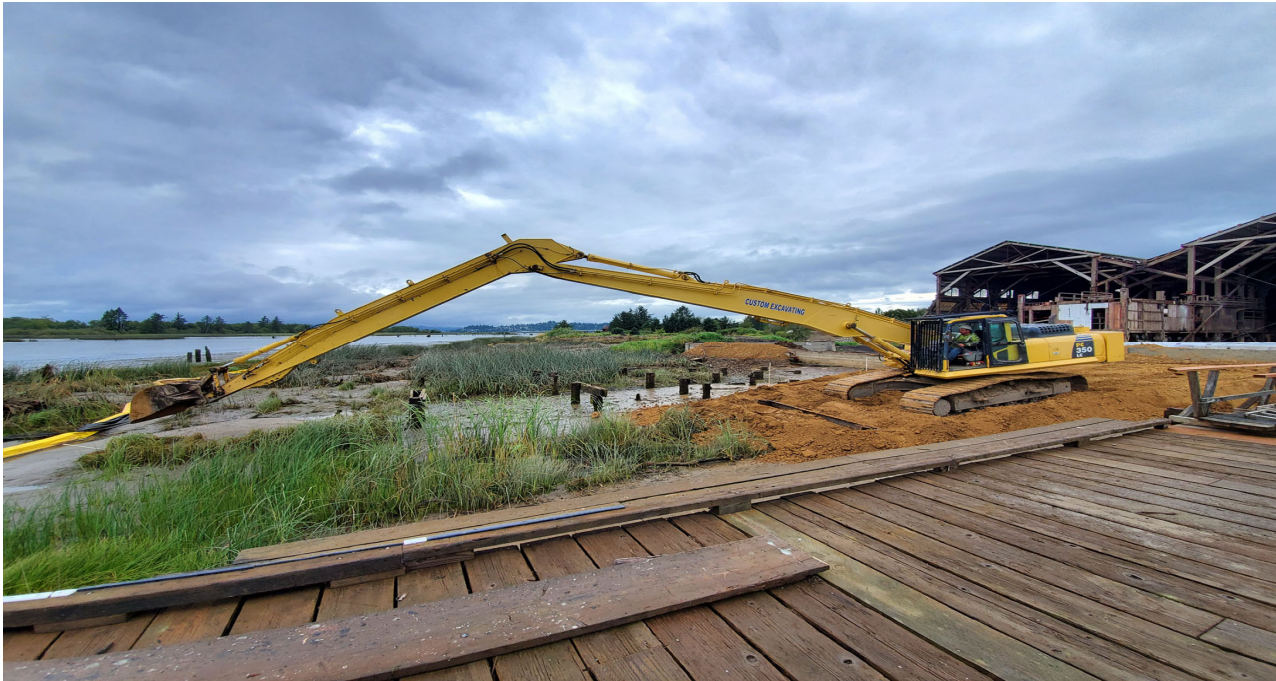
Photo 1: Custom Excavating beginning dredging work at marine way 3. Long reach excavator is operating on a temporary operation pad that was constructed with clean dike material.
