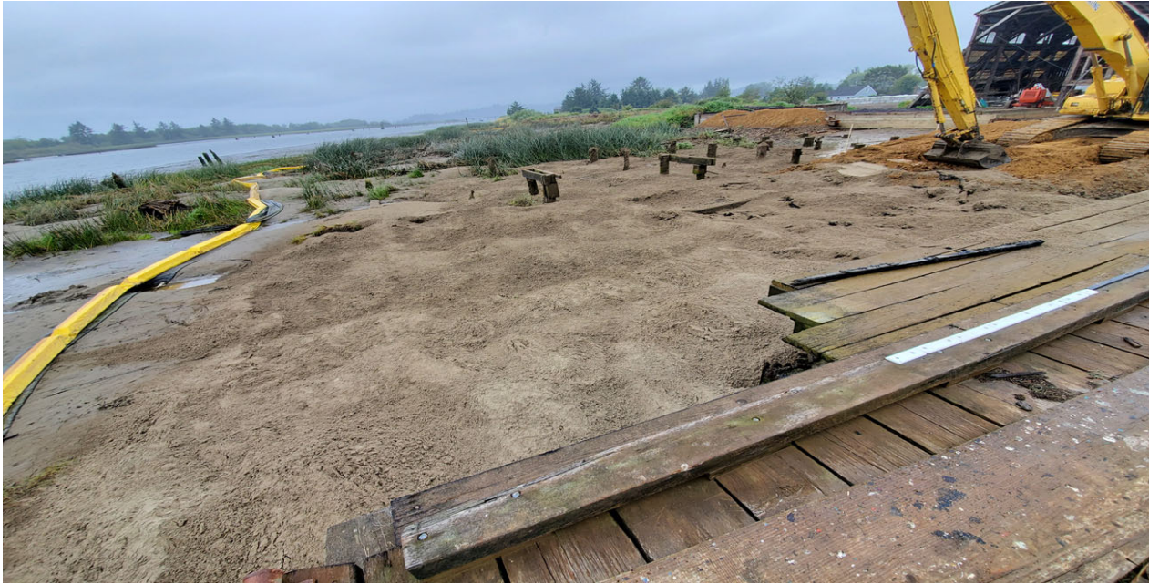
Photo 15: The work area covered with clean layer of sand. Placement of clean sand overlapped previously placed EMNR Sand Layer by couple feet.
