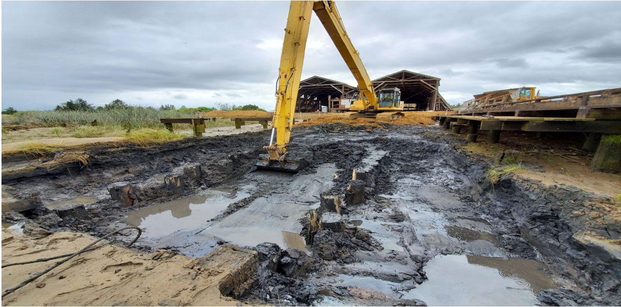
Photo 9: Custom Excavating dredging between pilings in marine way 3
