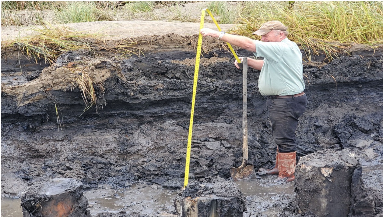
Photo 12: Measured dredge depth of approximately 5 feet at the north edge of marine way 3 dredge area
