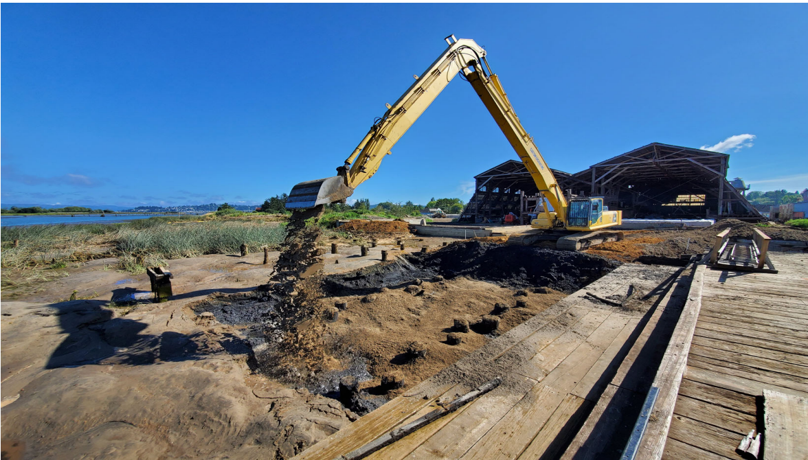
Photo 10: Custom Excavating backfilling dredged section of MW#3 dredge area with clean sand
