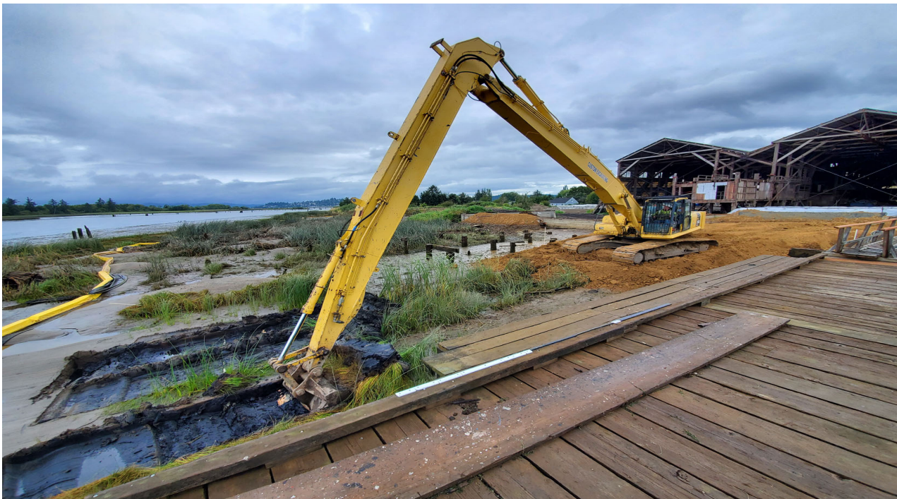
Photo 4: The top layer of sediment being removed in the western third portion of marine way 3
