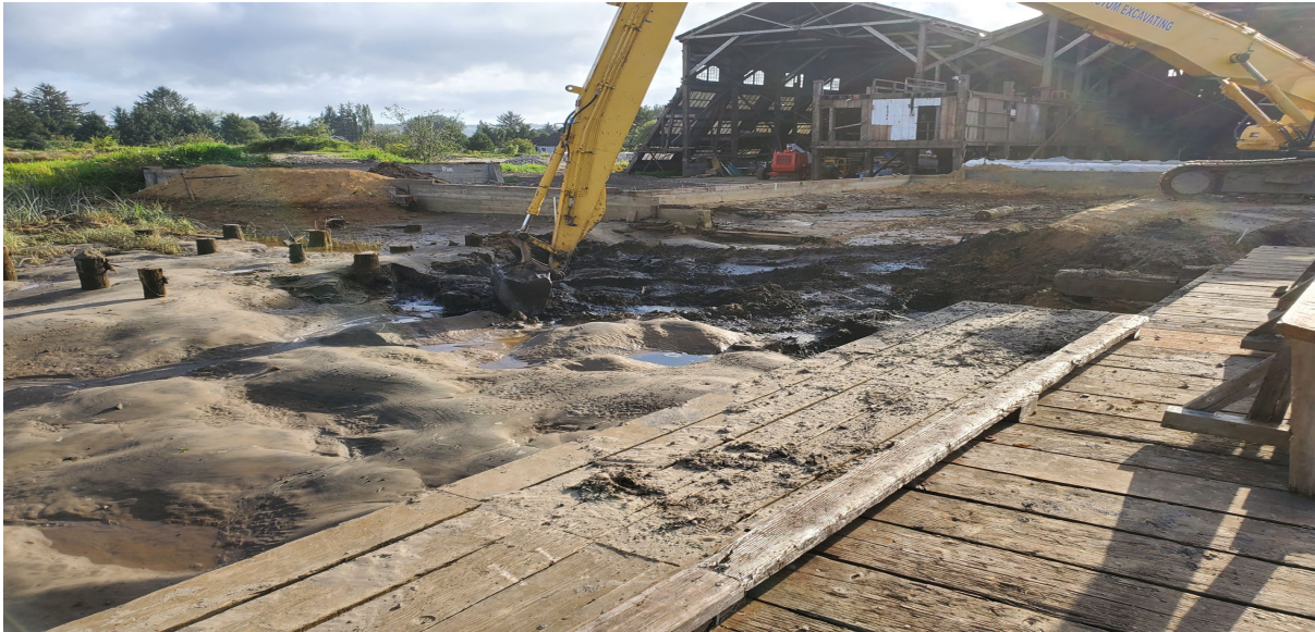
Photo 3: Custom Excavating started working on sediment excavation at the eastern third of MW#3 dredge area
