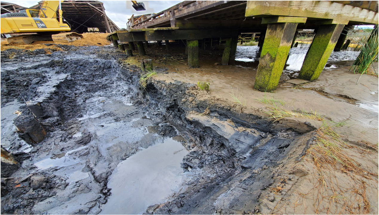
Photo 10: A look at the southern extents of the marine way 3 dredge area, along walkway platform
