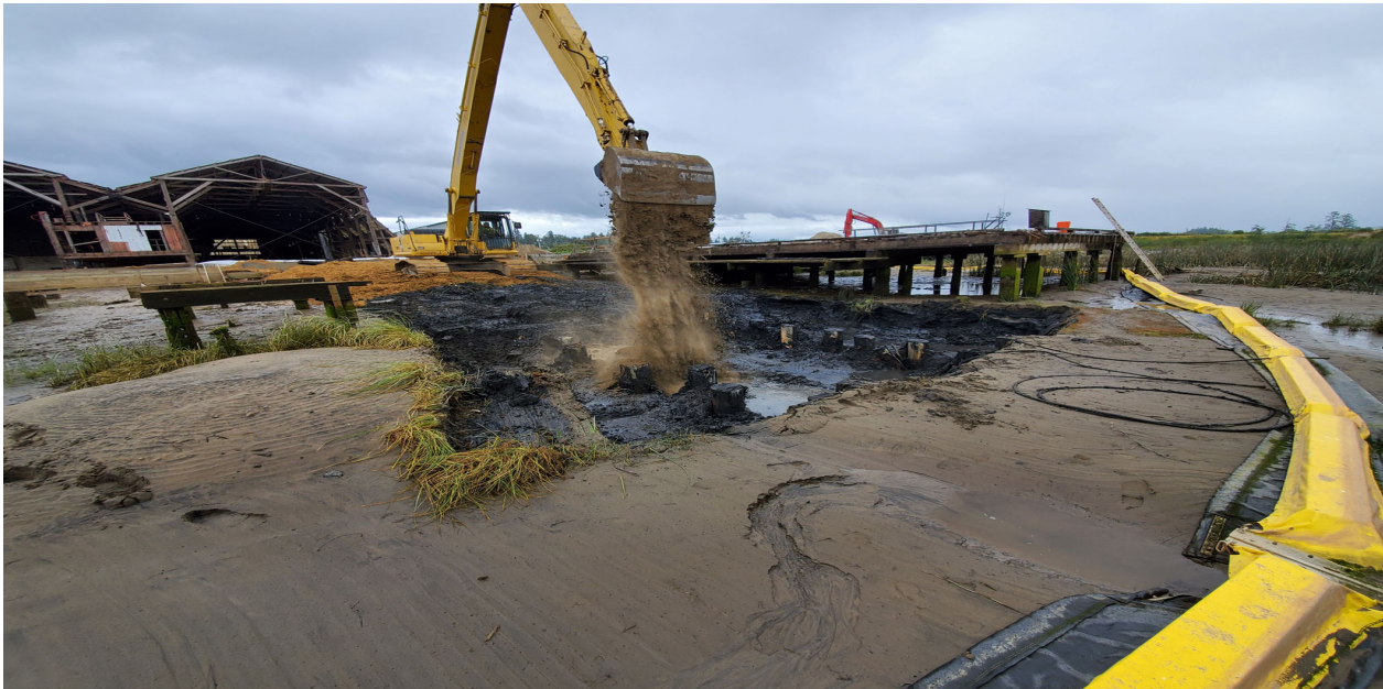
Photo 13: Custom Excavating backfilling marine way 3 dredge area with clean sand. Existing untreated pilings, that are approximately 18-inches apart, left in place and will have up to 18-24 inches of clean sand cover
