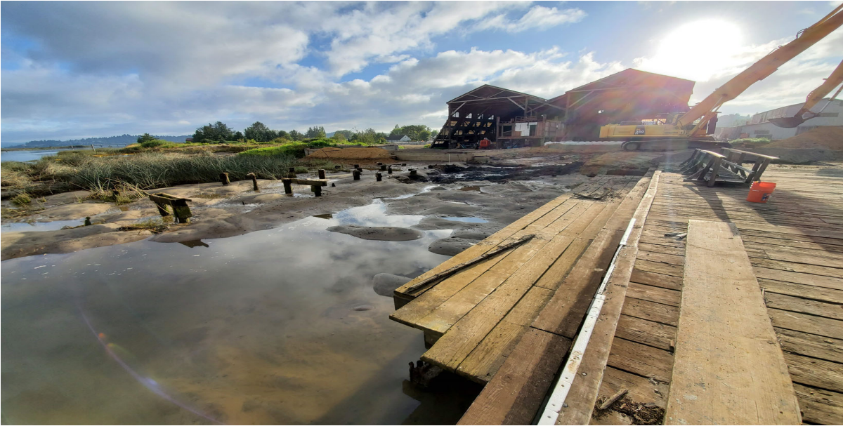
Photo 2: MW#3 progress view showing backfilled sand on the western two third, eastern third remaining to be dredged and backfill
