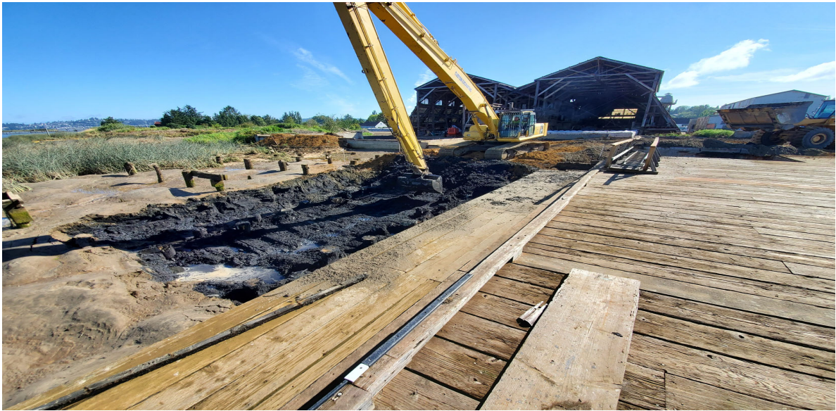
Photo 7: Custom Excavating excavating sediment at MW#3 dredge area, left-in-place, non-treated pilings are approximately 2 feet apart, and sticking up approximately 2 feet from the bottom of the excavation
