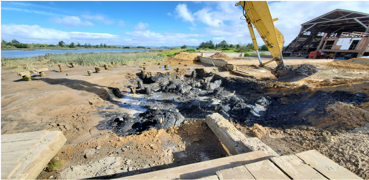
Photo 5: Custom Excavating eastern third of MW#3 dredge area, excavating between existing pilings that are approximately 18-24" apart
