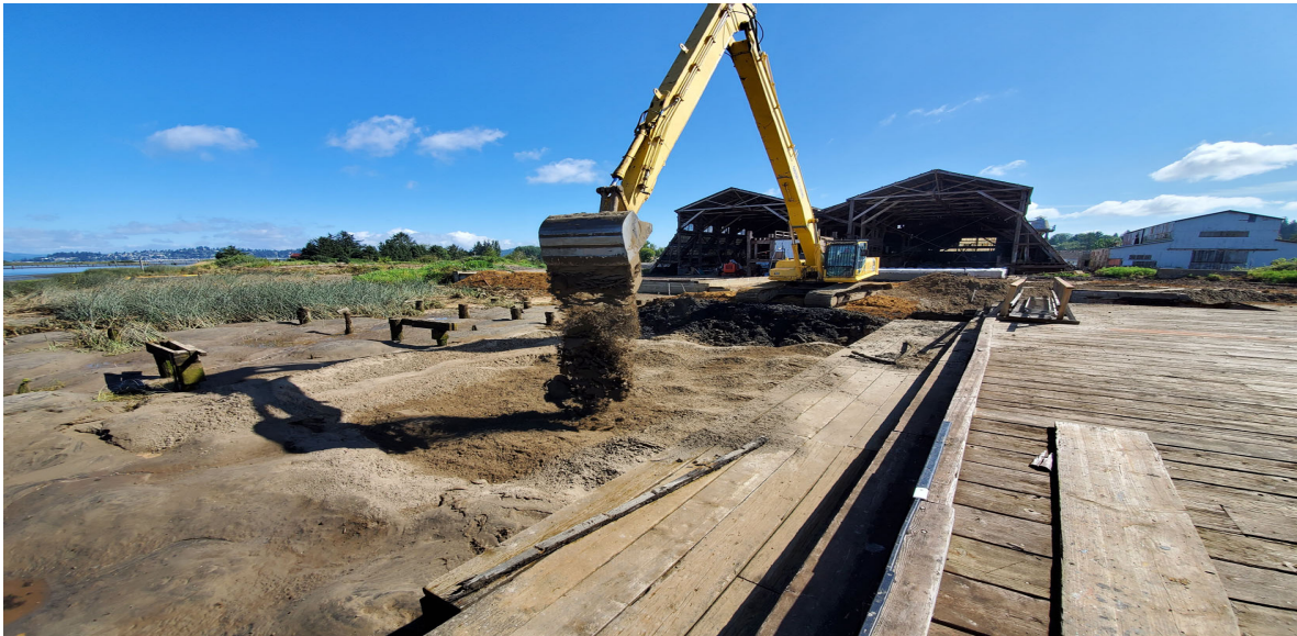
Photo 11: Custom Excavating backfilling dredge area with clean sand
