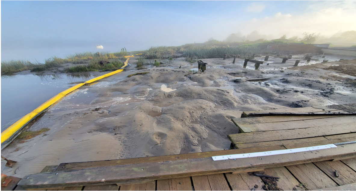
Photo 1: Clean sand-backfilled western most section of MW#3 dredge area
