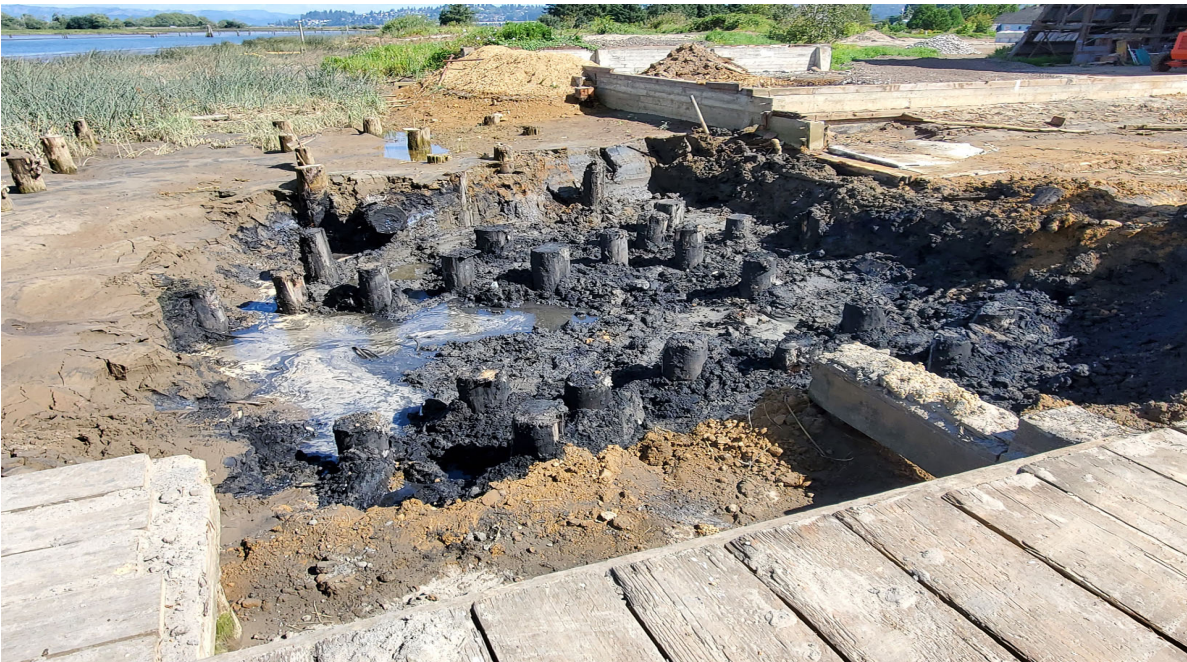
Photo 8: Bottom of sediment excavation at MW#3, untreated pilings terminate approx. 18-24 inches from the bottom, will receive 24-30 inches of clean sand cover
