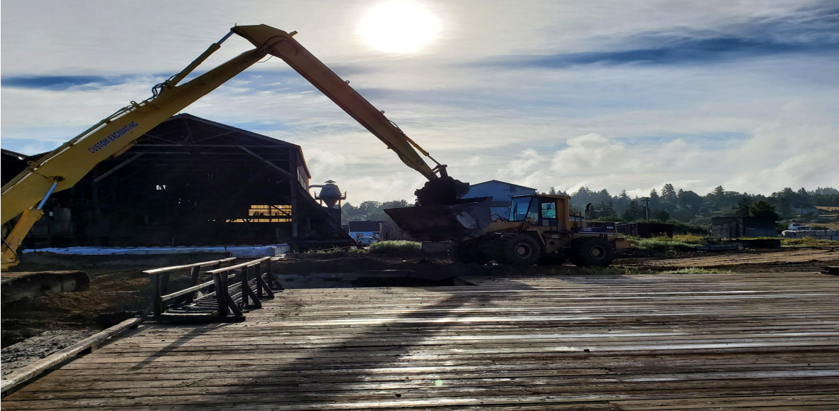
Photo 3: Custom Excavating loading the front loader with excavated sediment to transport to north sediment containment cell
