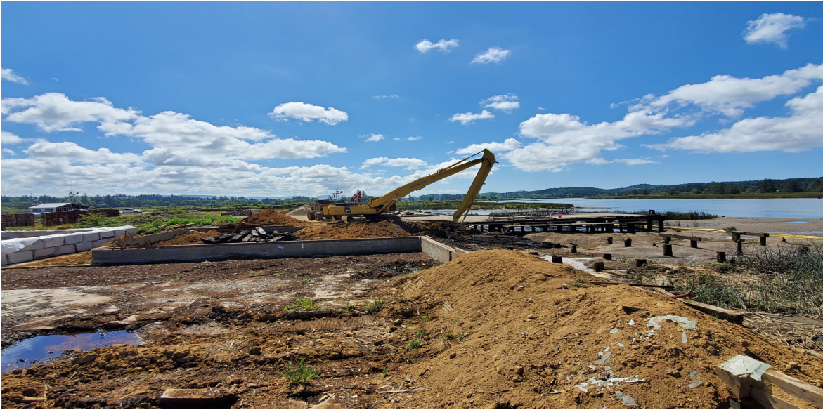
Photo 13: Custom Excavating dredging eastern portion of MW#3 dredge area, looking south from north section of existing dike wall
