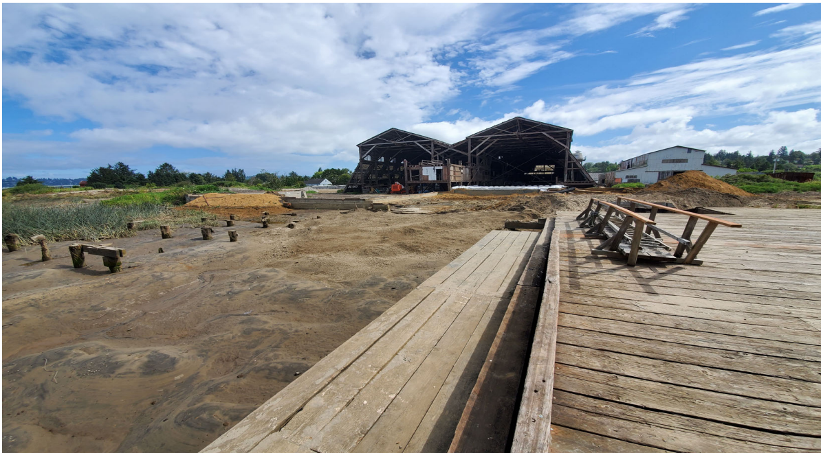
Photo 10: Final Surfacing at MW#3 Dredge Area: dredge and backfill work completed
