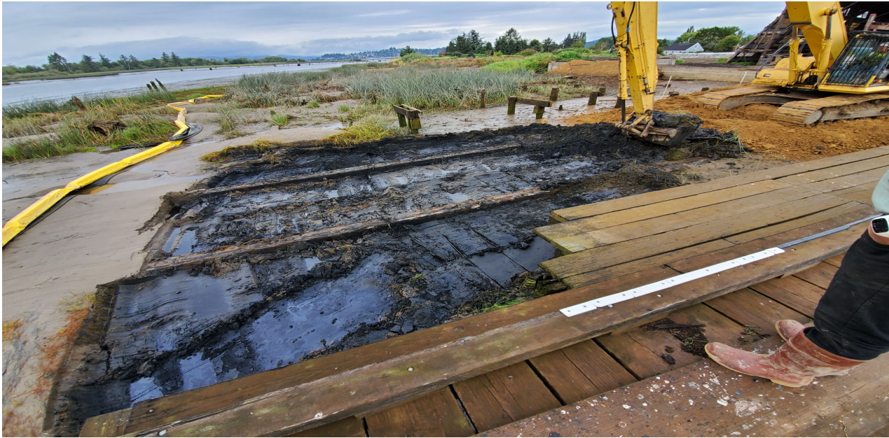
Photo 5: Exposed rail support structure in the western portion of marine way 3
