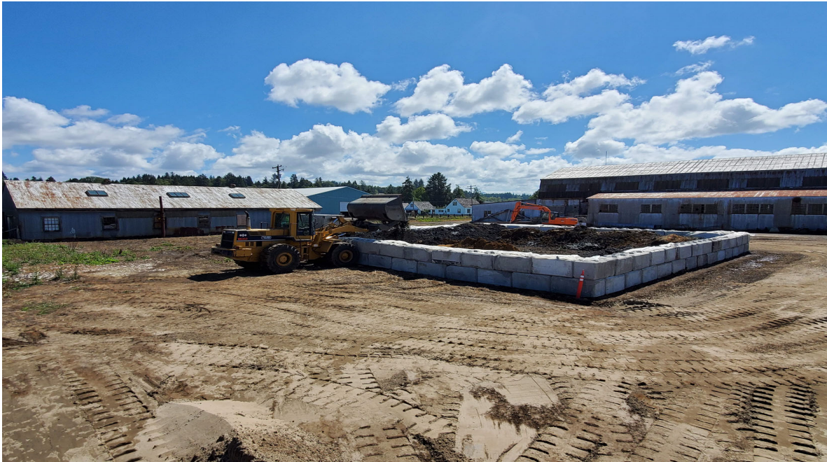
Photo 12: Front loader unloads excavated sediment to north sediment containment cell
