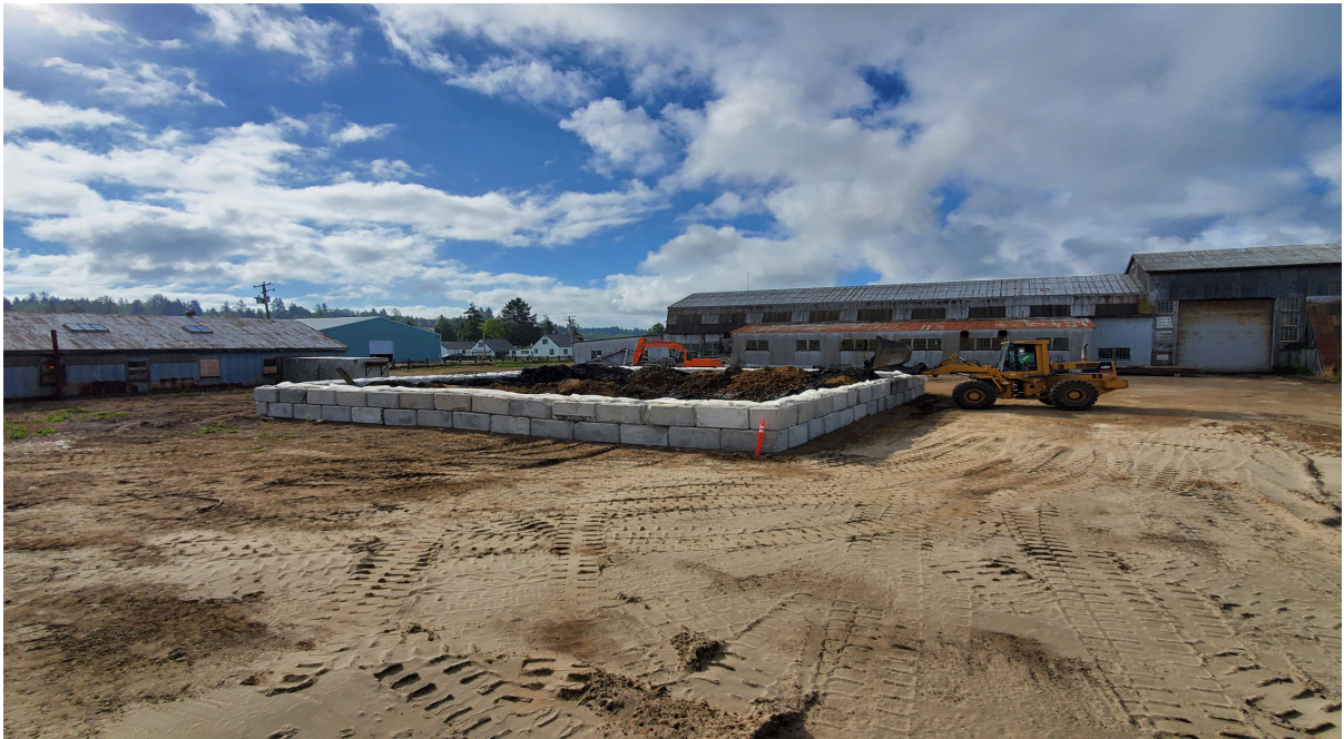
Photo 4: Front loader unloading excavated sediment at north sediment containment cell
