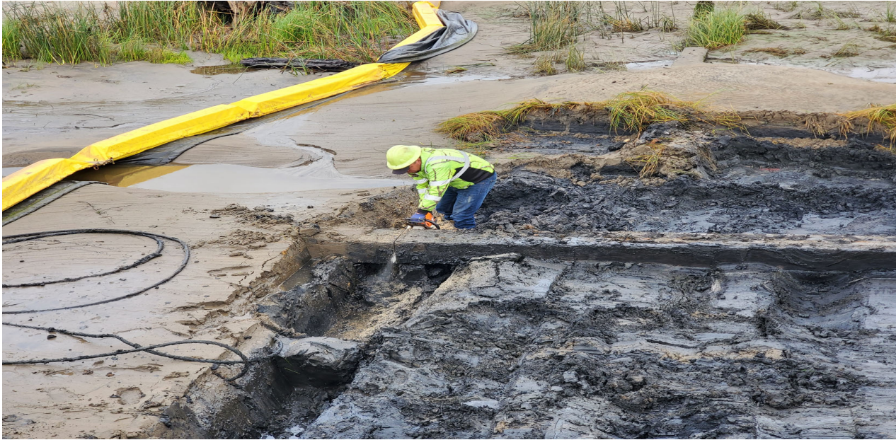
Photo 7: Custom Excavating using a chainsaw to break up and remove the marine way 3 wooden rail support structure to access the lower sediment
