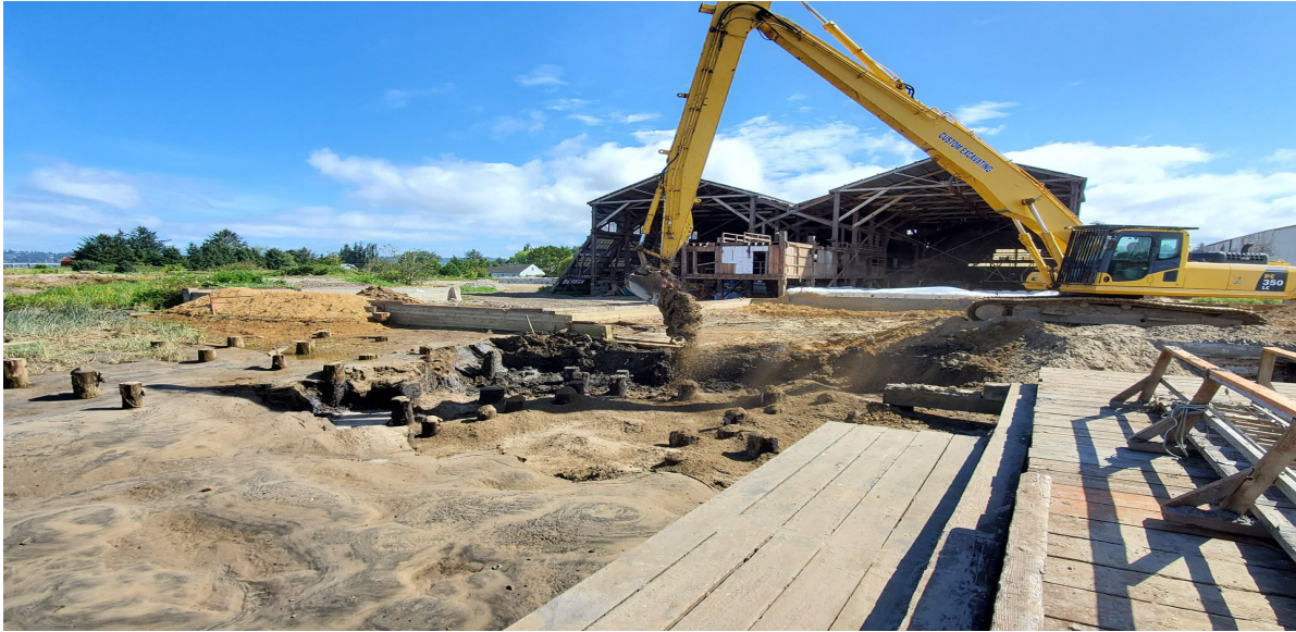
Photo 9: Custom Excavating backfilling eastern most section of the dredged area with clean sand, temporary clay work platform has been removed
