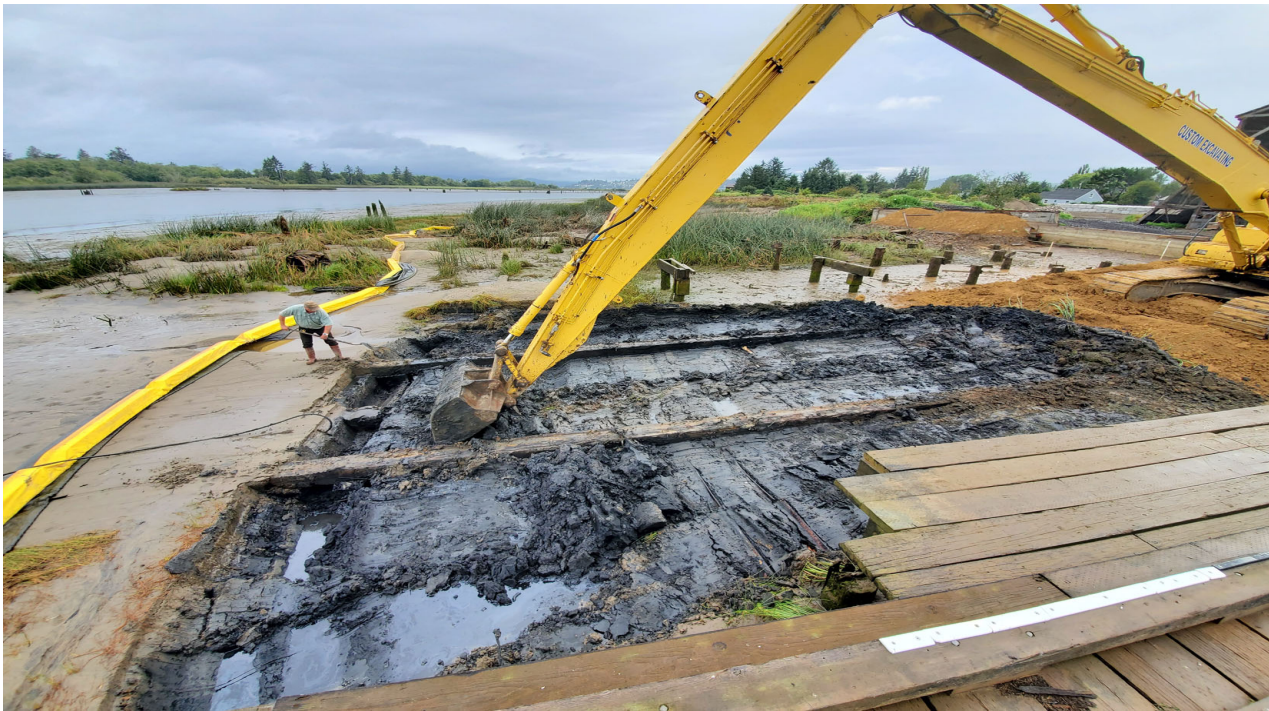
Photo 6: Custom Excavating removing sediment between the rail support structure
