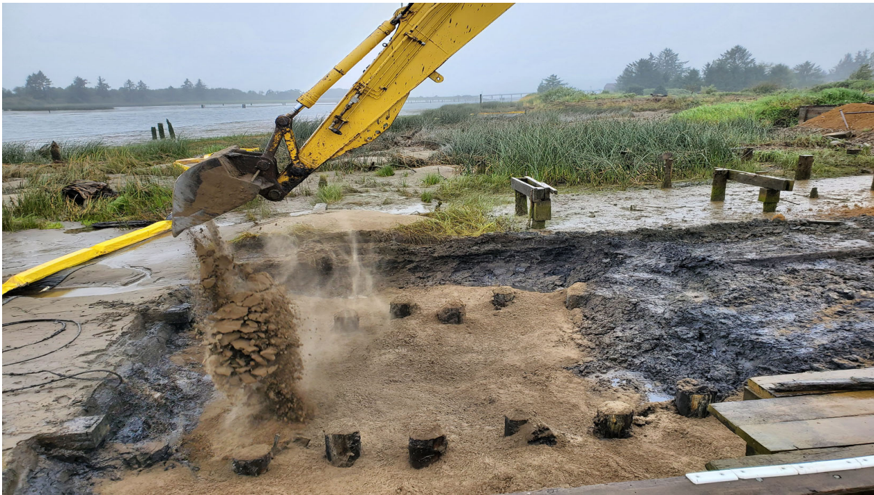
Photo 14: Custom Excavating backfilling marine way 3 dredge area with clean sand
