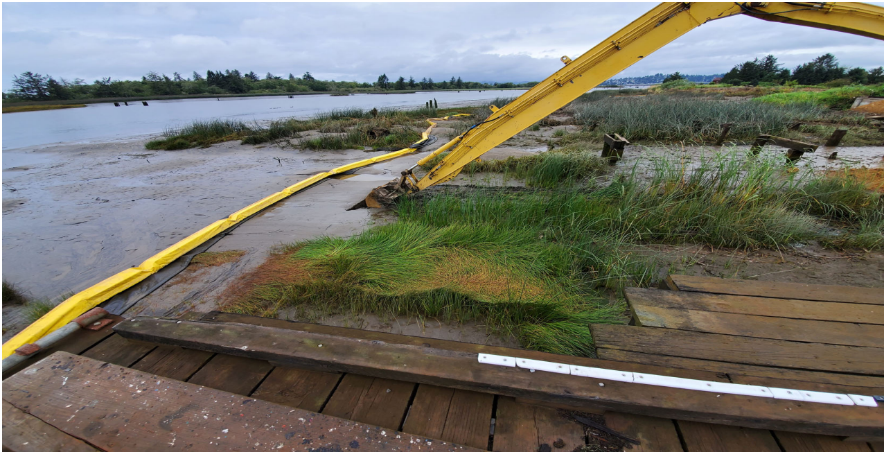
Photo 2: Custom Excavating removing top layer of sediment located above the marine way 3 rail support structure at the western most end of the dredge area
