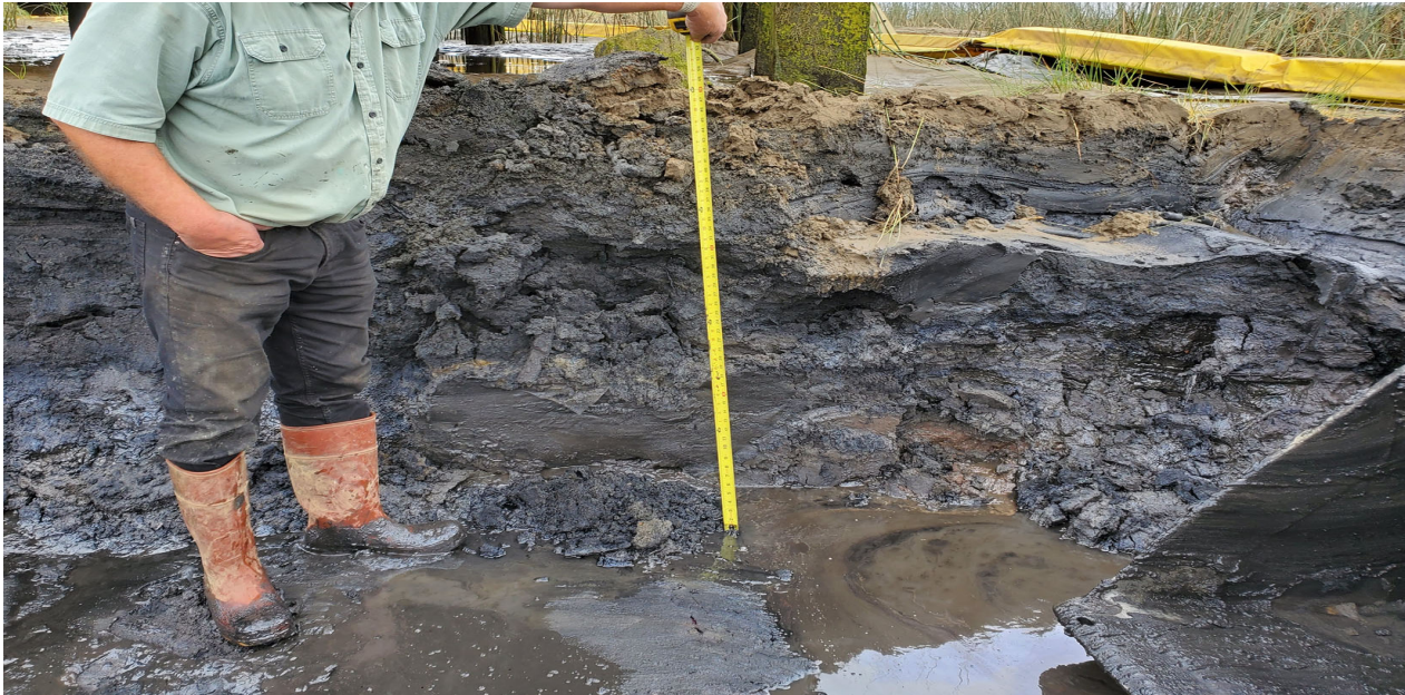
Photo 11: A dredge depth of 4 feet at the southern extents of marine way 3 dredge area
