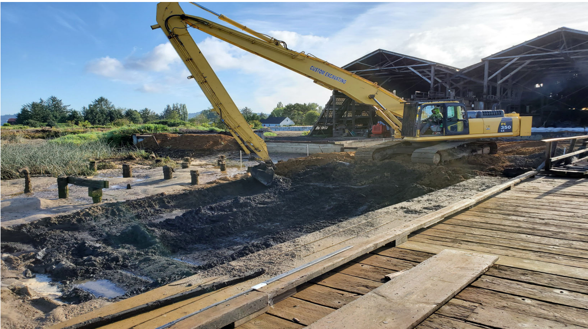
Photo 4: Custom Excavating dredging central portion of MW#3 dredge area
