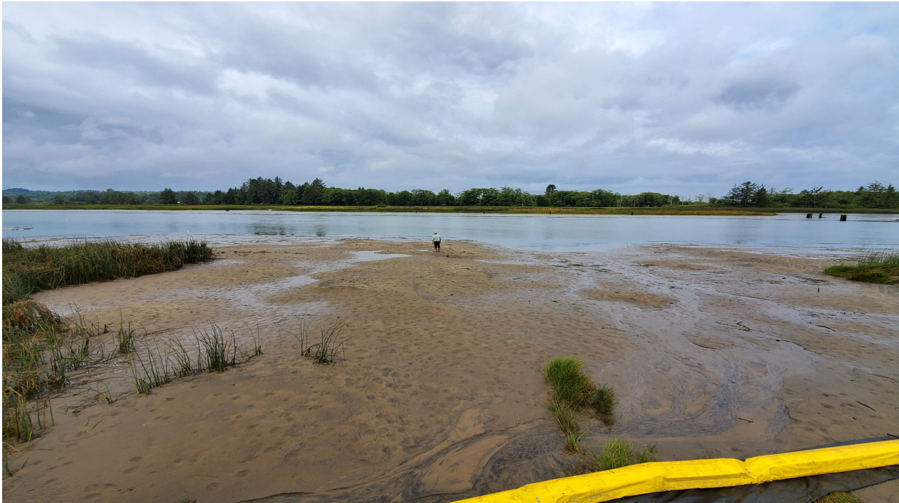
Photo 8: A look at the previously placed EMNR sand layer west of marine way 3 dredge area during low tide
