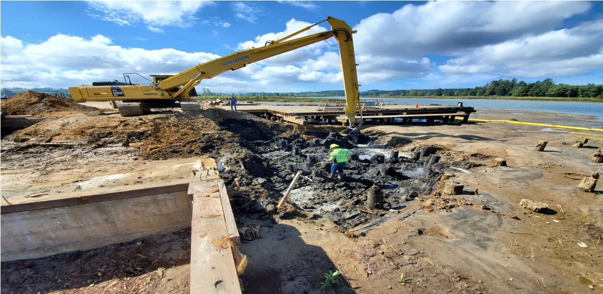
Photo 7: Custom Excavating removing sediment between existing pilings with the help of manual labor within the dredge boundary
