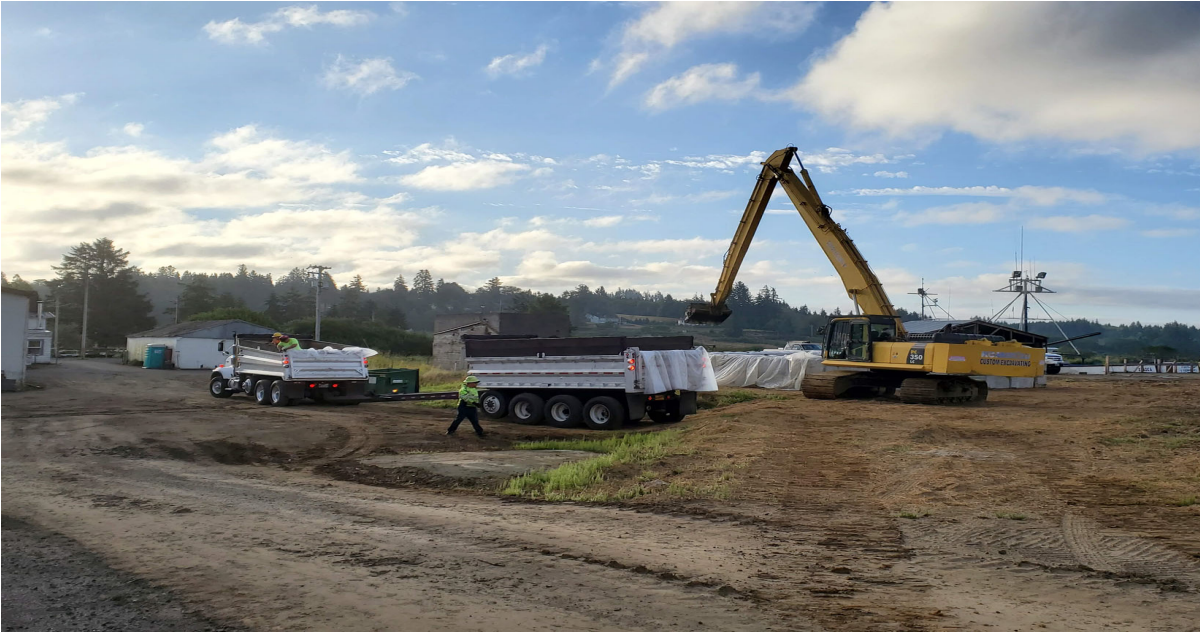
Photo 1: Custom Excavating loading dump truck from south sediment containment cell to haul off excavated material to Hillsboro landfill
