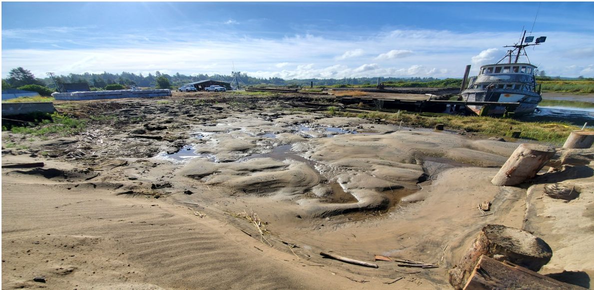
Photo 5: Previously backfilled and EMNR layer placed at MW#2 dredge area
