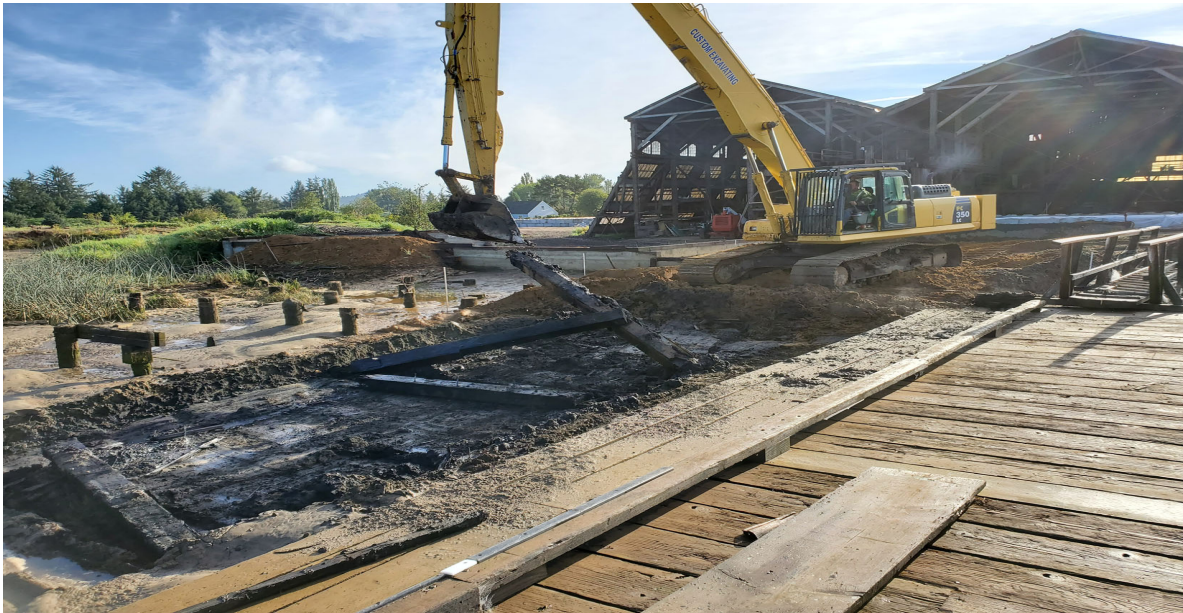
Photo 2: Custom Excavating removing wooden beams that had supported the former rail system for sediment excavation at the central portion of MW#3 dredge area
