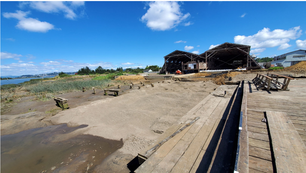
Photo 14: 2/3 of MW#3 dredge area final surface: backfilled and received EMNR Sand layer
