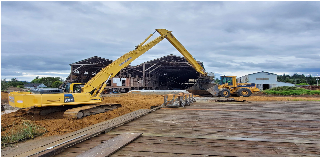
Photo 3: Custom Excavating placing excavated sediment in the front loader
