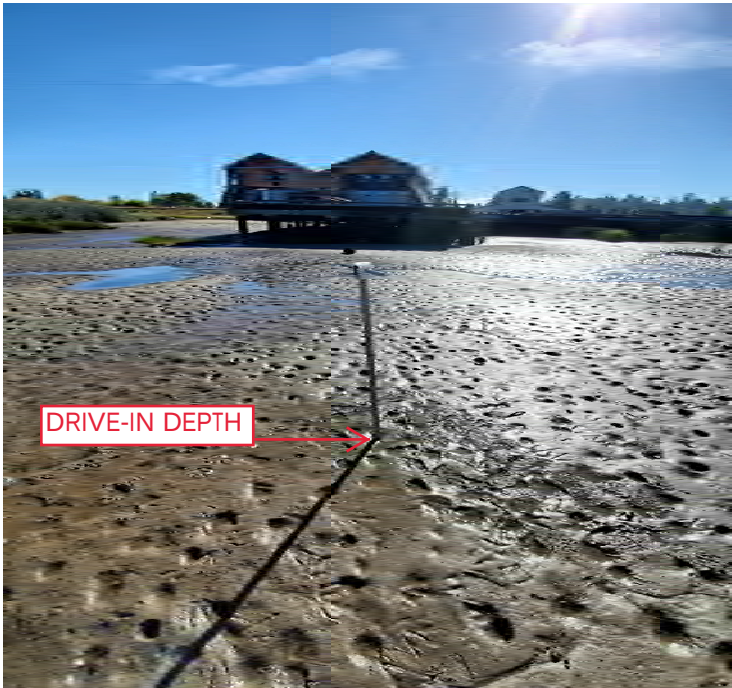
Photo 1: A look at the drive-in location of the russian pete bore at SP 5
