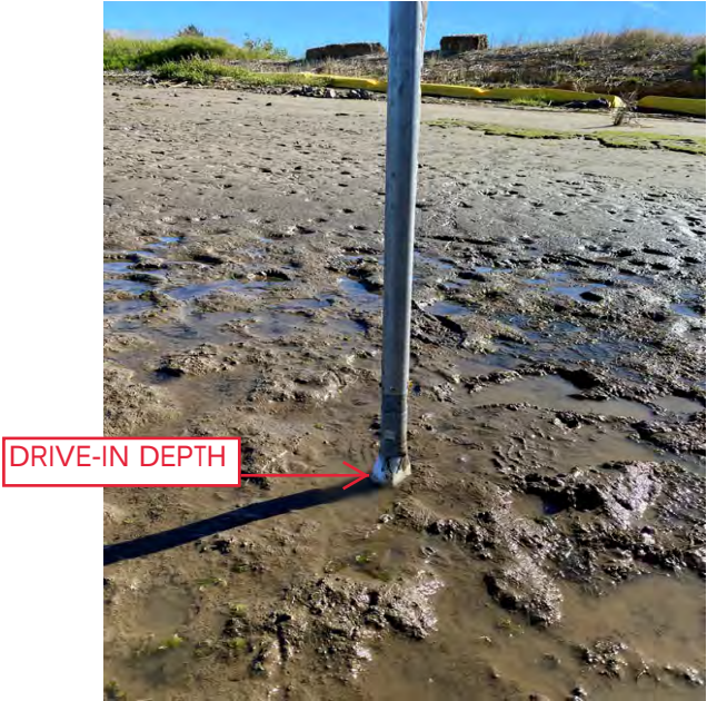
Photo 13: A look at the drive-in location of the russian pete bore at SP 16
