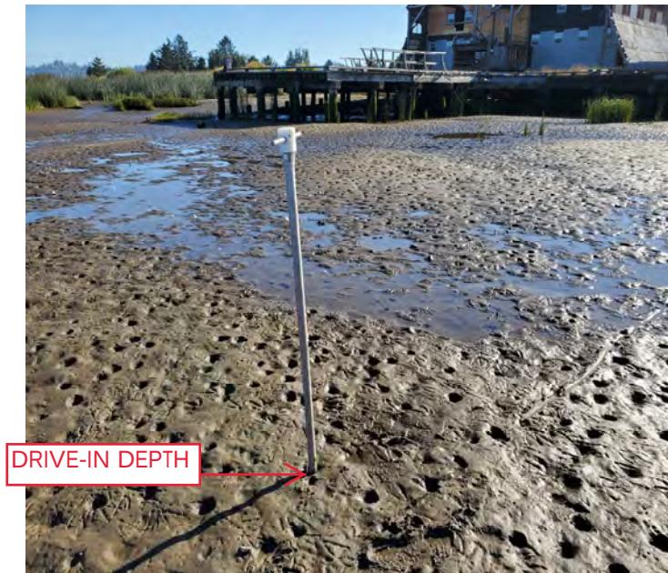
Photo 7: A look at the drive-in location of the russian pete bore at SP 13
