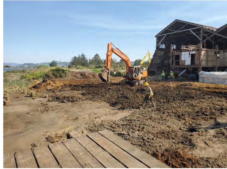
Subgrade being Scarified (Facing North)
