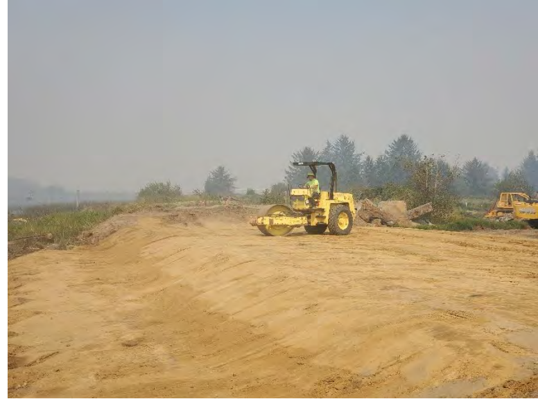
Fill being Keyed into Existing Dike (Facing North)
