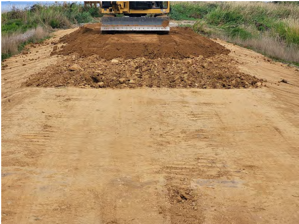
Example of soil being scarified prior to placement of additional lift
