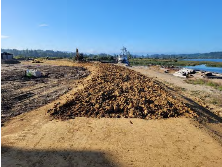
Soil being moisture conditioned
