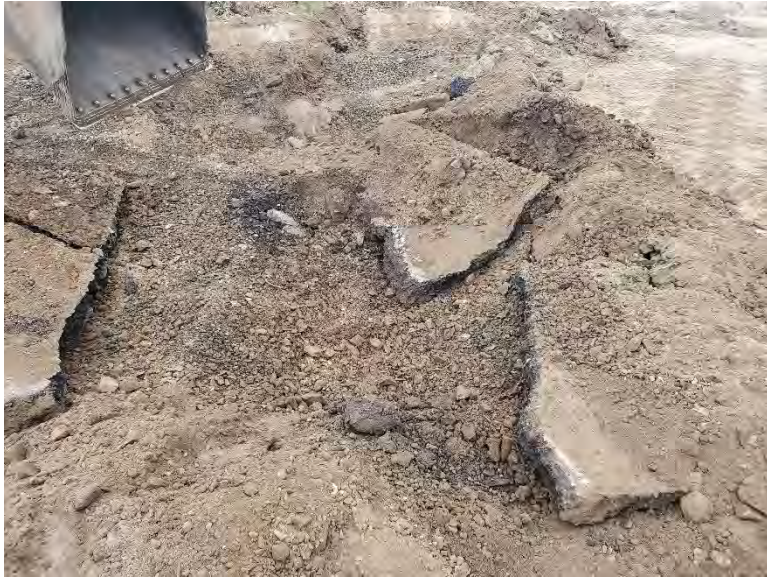
Example of Asphalt and Crushed Rock in Dike Subgrade
