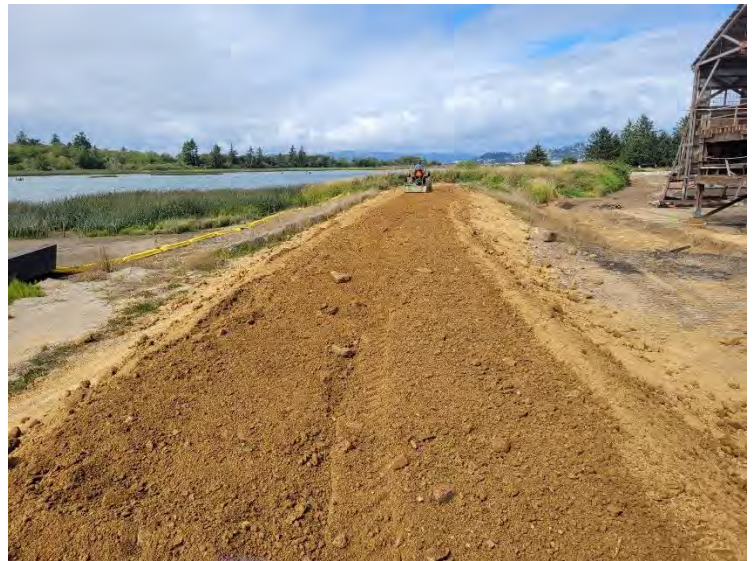
Soil being moisture conditioned
