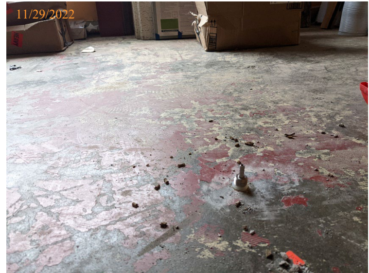
Vapor pin installed in concrete slab floor of former drycleaner shop (space 1220) for collection of SUB08.
