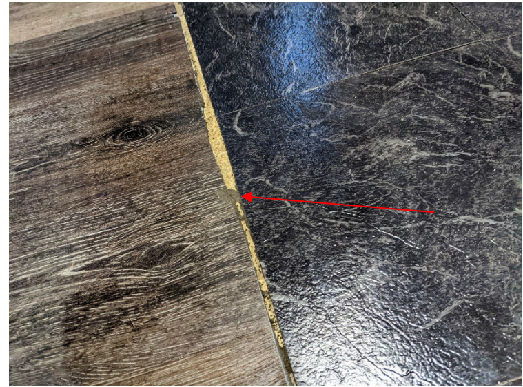
Following sampling, Vapor pins were removed, and slab penetrations sealed with hydraulic cement.
