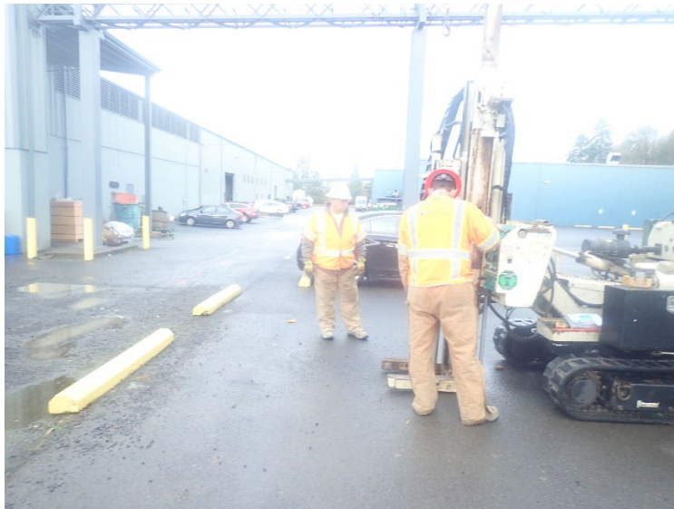
Drill rig set up on boring EB05, looking north.
