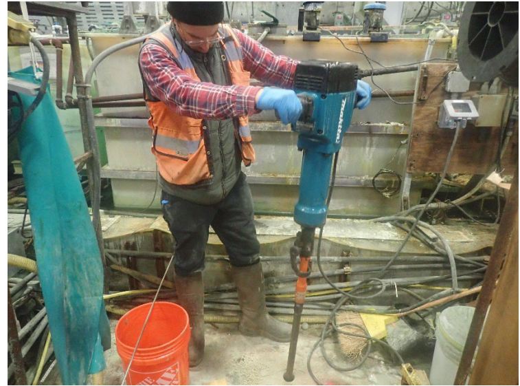
Using DPT to advanced borings EB02 and EB3 inside Bldg. 2.
