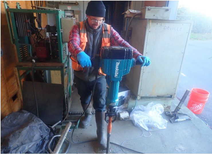
Advancing EB01 on Nov. 18, 2022, using DPT drill rods.
