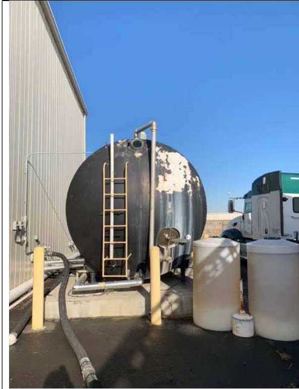
Exterior tank (View 2)
