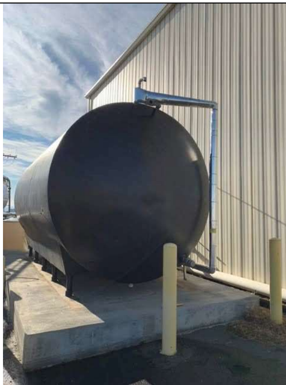
Exterior tank (View 1)
