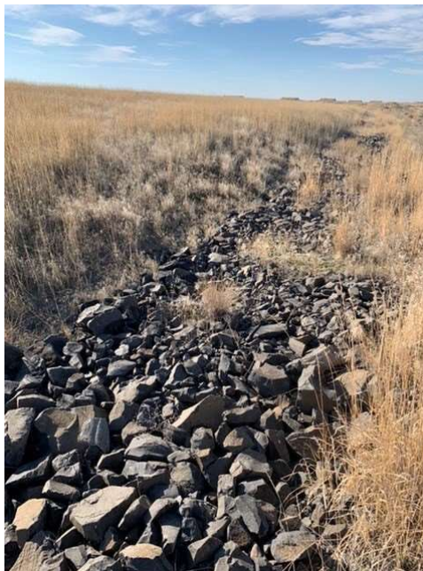
Rock at landfill toe
