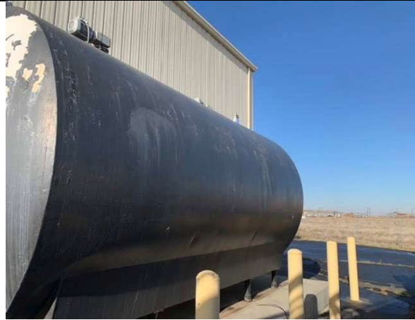
Exterior tank (View 3)
