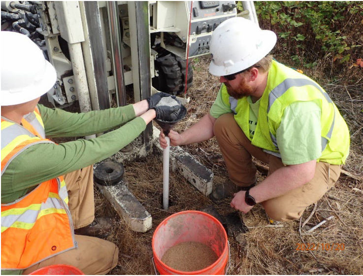
Semi-permanent monitoring points were constructed within the borings.
