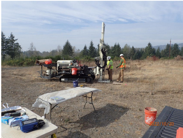
Permanent soil gas monitoring points were installed with the assistance of a direct-push drill rig.
