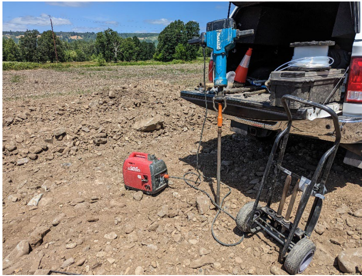
An electric jack hammer was also used to drive temporary soil gas probes in rocky areas.
