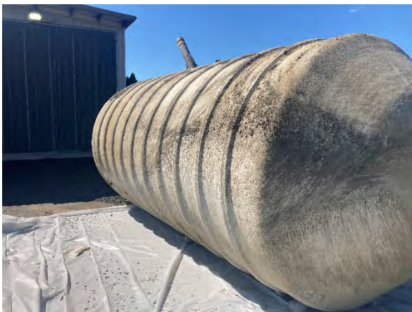
Photo #5 6,000-gallon Jet-A UST after removing from tank nest.
