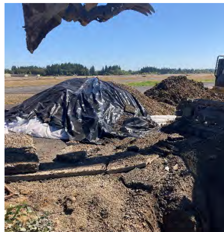
Photo #12 Stockpiled PCS prior to off-Site disposal.
