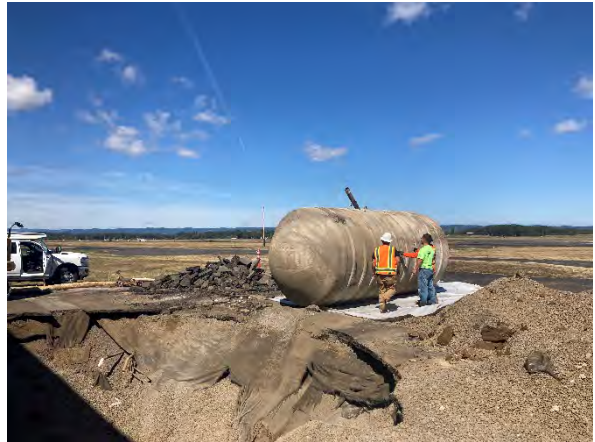
Photo #2 6,000-gallon Jet-A UST after removing from tank nest.
