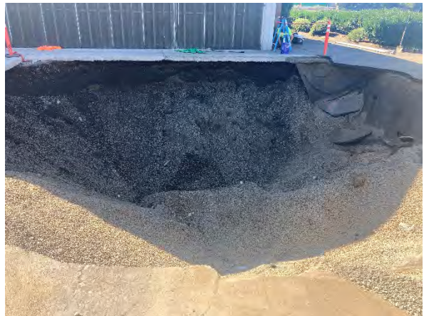
Photo #4 Tank nest excavation looking west southwest.
