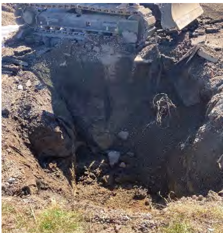
Photo #11 Excavation at former fueling area on northeast portion of property.
