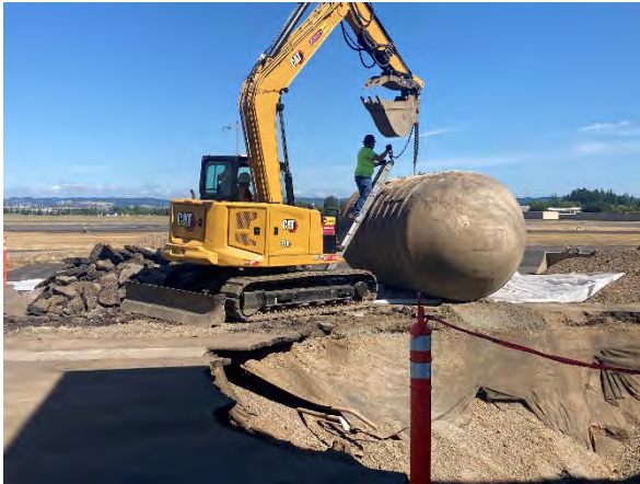
Photo #7 UST being lifted onto trailer for off-Site disposal.
