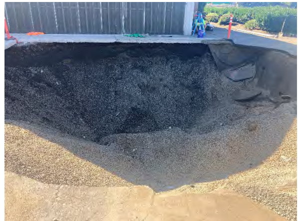
Photo #4 Tank nest excavation looking west southwest.
