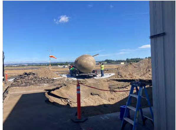
Photo #8 UST being lifted onto trailer for off-Site disposal.
