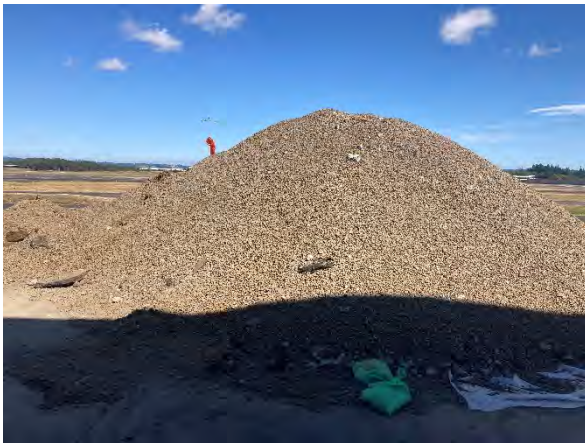
Photo #3 Pea gravel overburden from tank nest during decommissioning by removal.
