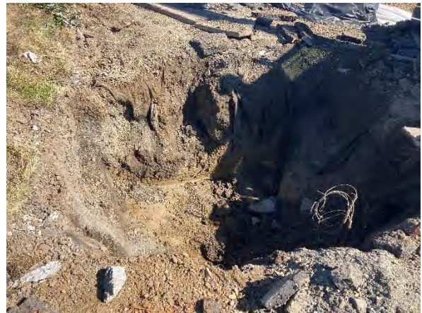
Photo #10 Excavation at former fueling area on northeast portion of property.
