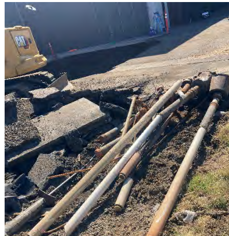
Photo #6 Pumps, risers, fill, and vent lines during decommissioning.
