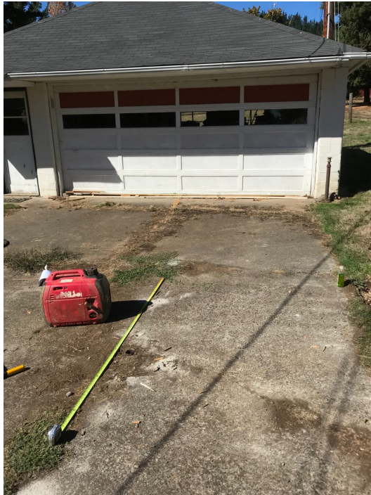
The site had an underground storage tank located south of the garage within the driveway.
