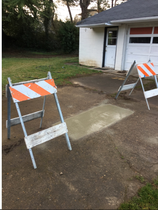
The UST area was restored to grade with a concrete patch.
